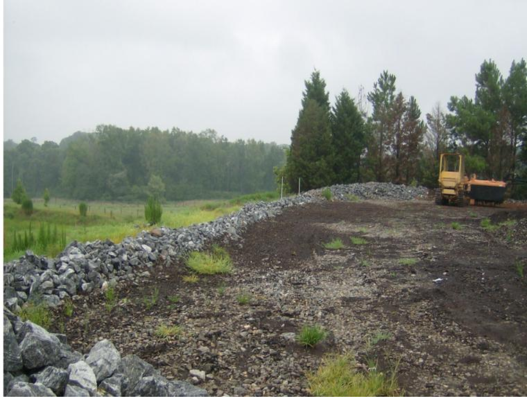
Figure B.3: Image of the lower section of the compost pad with gravel embankment (left) where water has been found to pool as surface storage. This section is represented by compartment two in the compartmentalized model.
