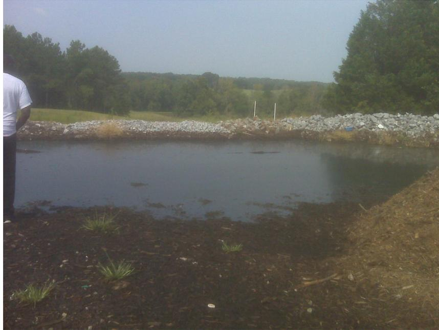
Figure A.2: Surface storage that can occur at the lower section of the compost pad due to the embankment.
