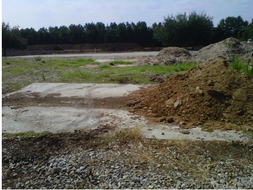
Figure A.8: There are six concrete pads that contain small volumes of compost material that drain directly to the collection pond.
