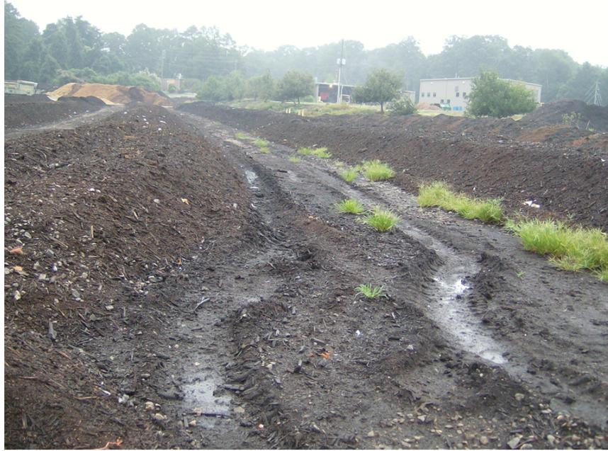
Figure A.3: Image of tire tracks that occur of compost pad. Storage shown in the depression of the tracks was found 6 hours after the previous storm.
