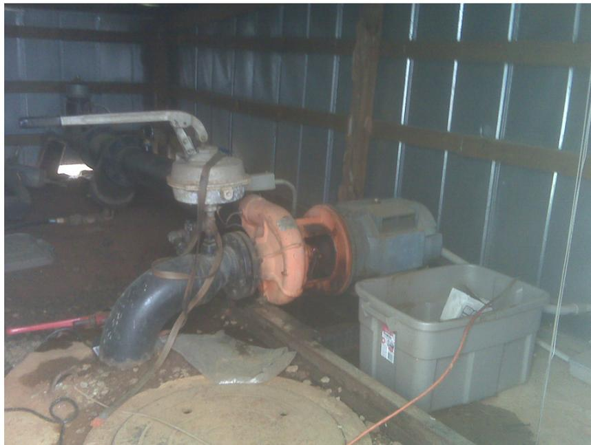
Figure A.7: Image of the pump that pumps water from the collection pond and uses it for spraying. The pump is rated to operate at 1516 L/min (400 gal/min).
