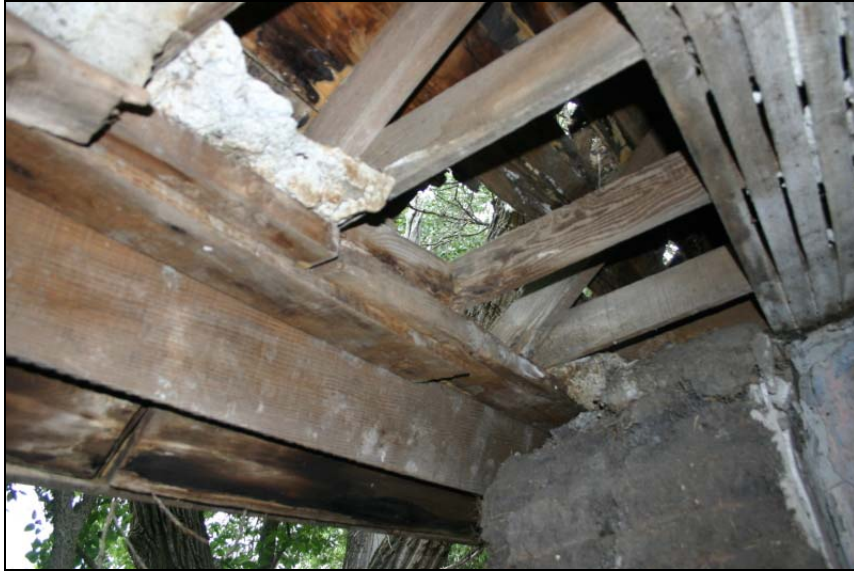
Figure 52. Sod – 04, Detail of Wonch Sod House built up top plate
