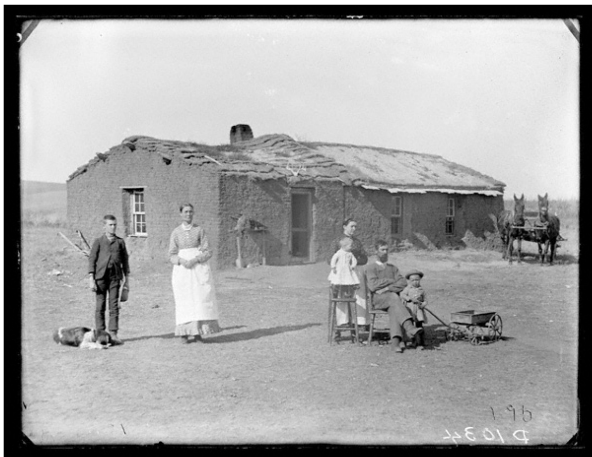
Figure 30. Three beam gable roof using a brush and pole method on the left and using vertically placed wood planks on the right, circa 1886
