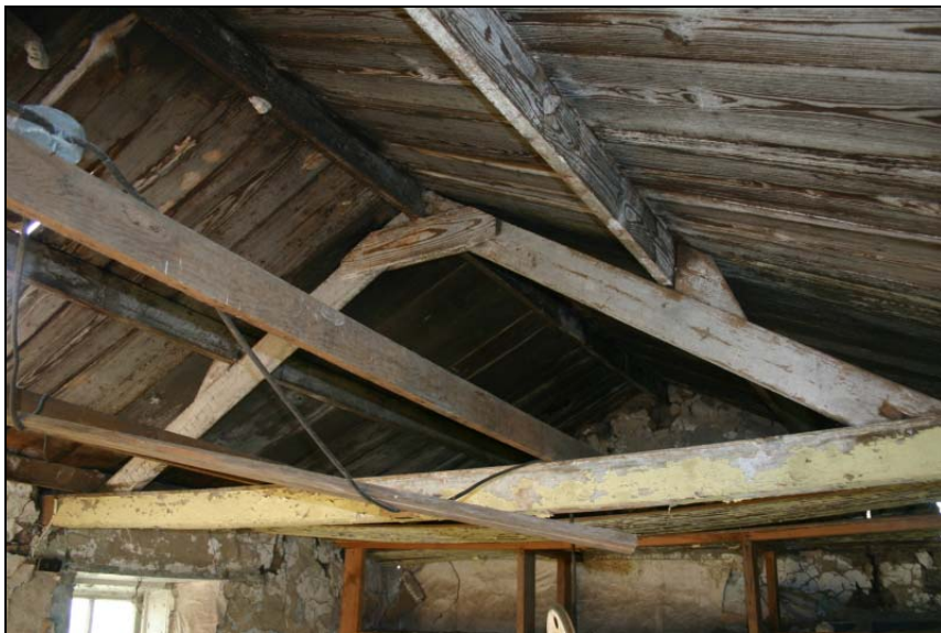
Figure 53. Sod – 17, Detail of McNulty Sod House roof framing
