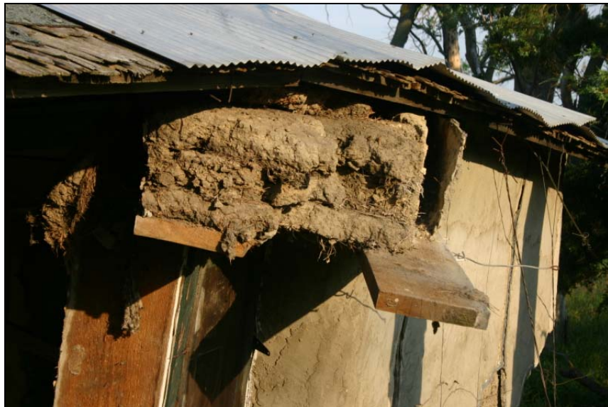
Figure 51. Sod – 17, Detail of McNulty Sod House window lintels and sod
