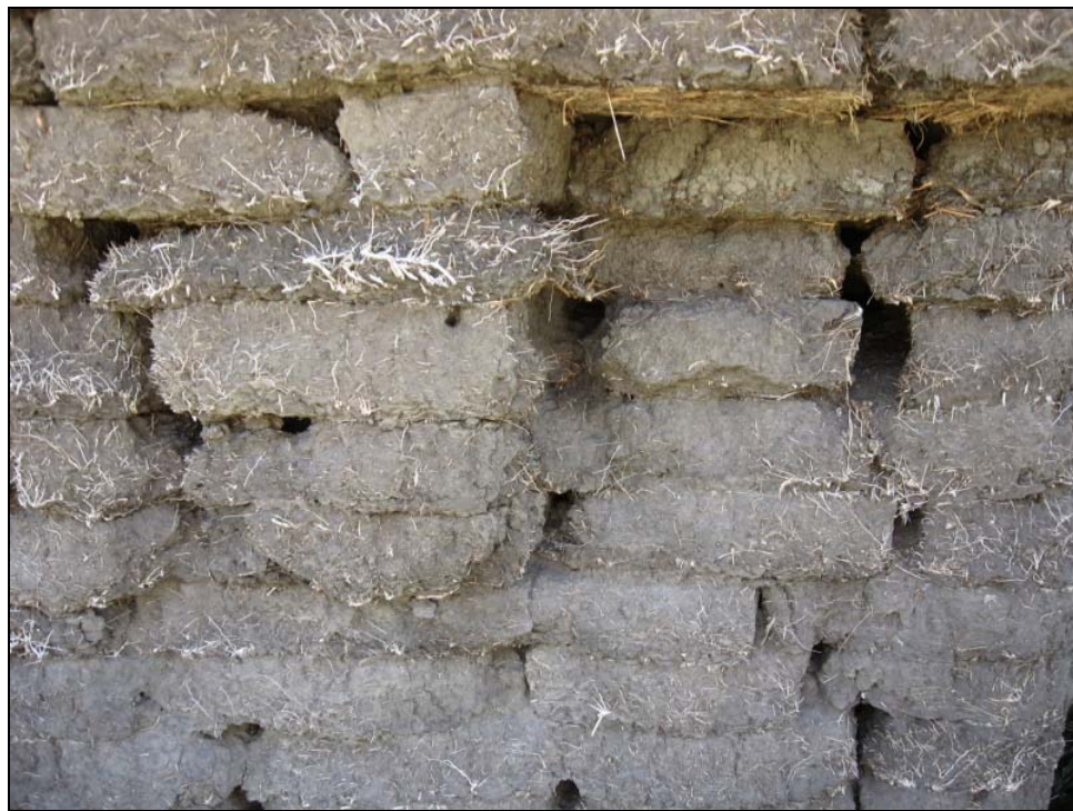
Figure 10. Wall construction: blocks laid two wythes deep with alternating headers and stretchers
