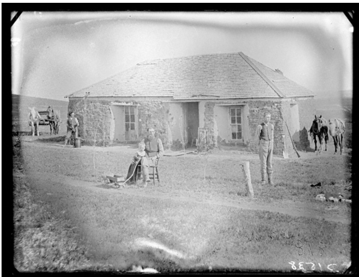
Figure 27. Photograph showing plaster on portions of exterior walls, circa 1890
