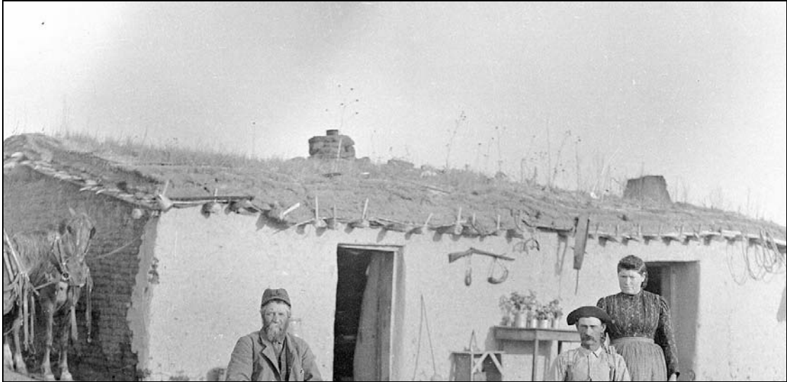
Figure 17. Roofs: To keep sod from slipping off roof, pegs were sometimes inserted into the ends of rafters
