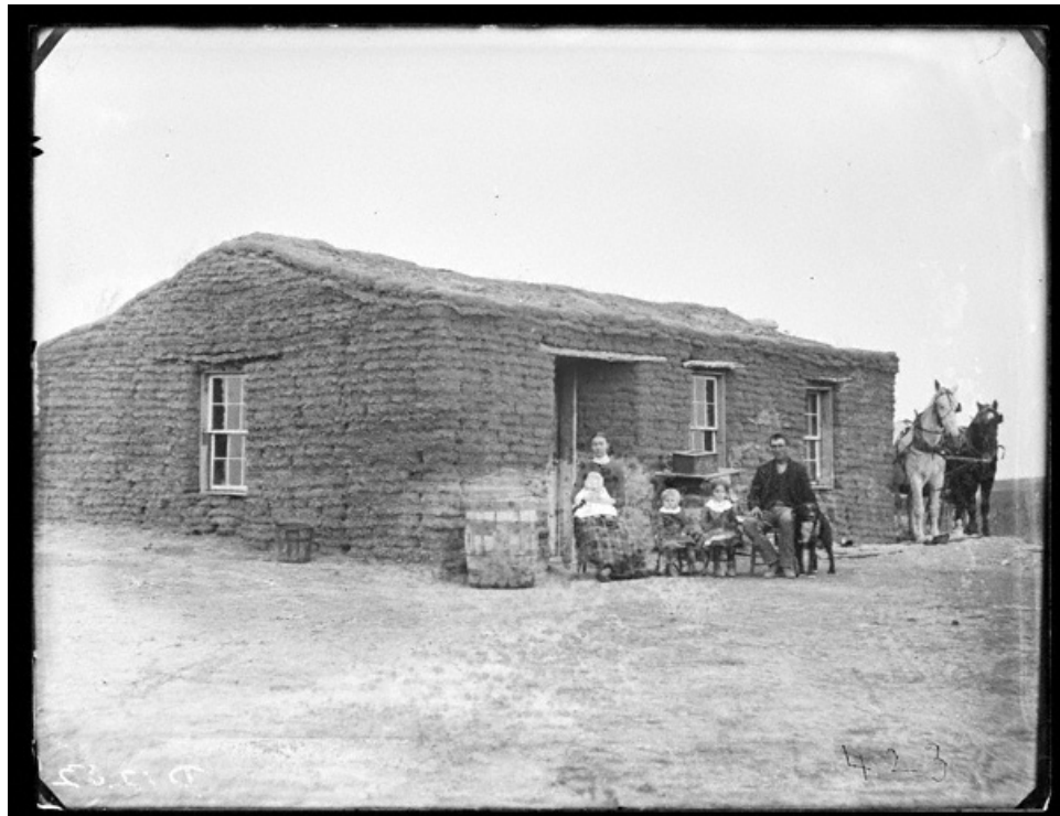
Figure 18. Roofs: Eaves eliminated and walls rounded up to the plane of the roof
