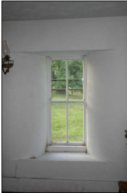
Figure 50. Sod – 11, Detail of Dowse Sod House arched beveled window wells
