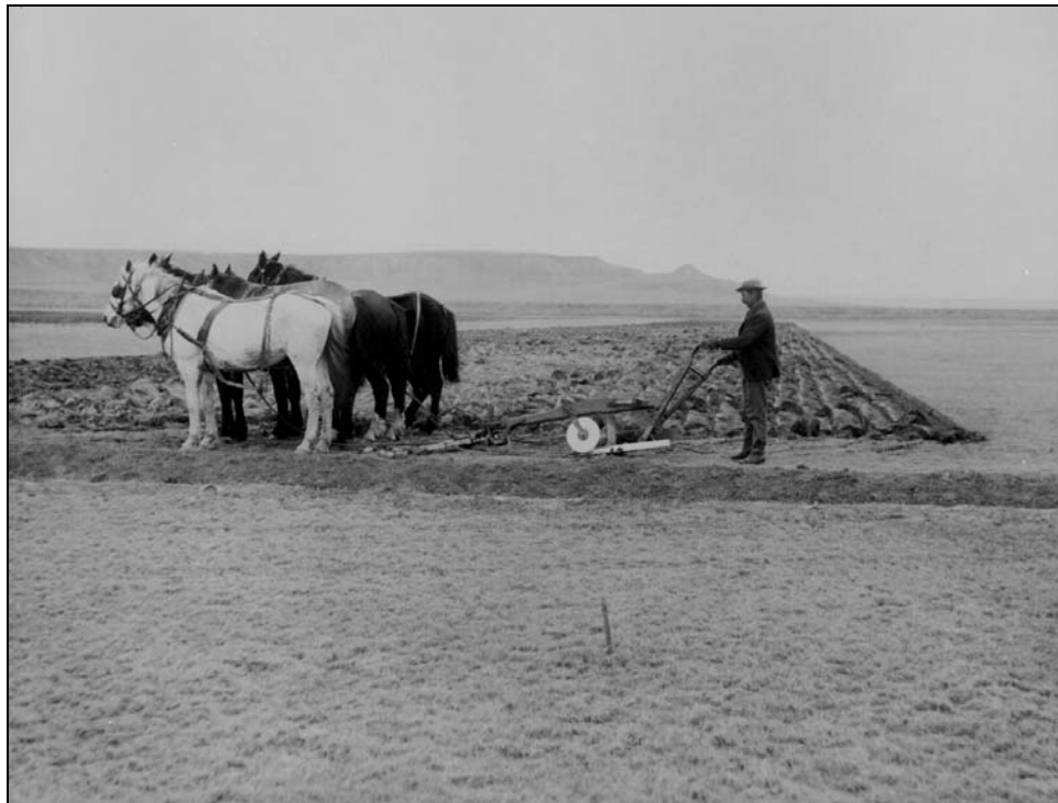
Figure 9. Material preparation: grasshopper plow and its use in cutting the sod by a team of horses
