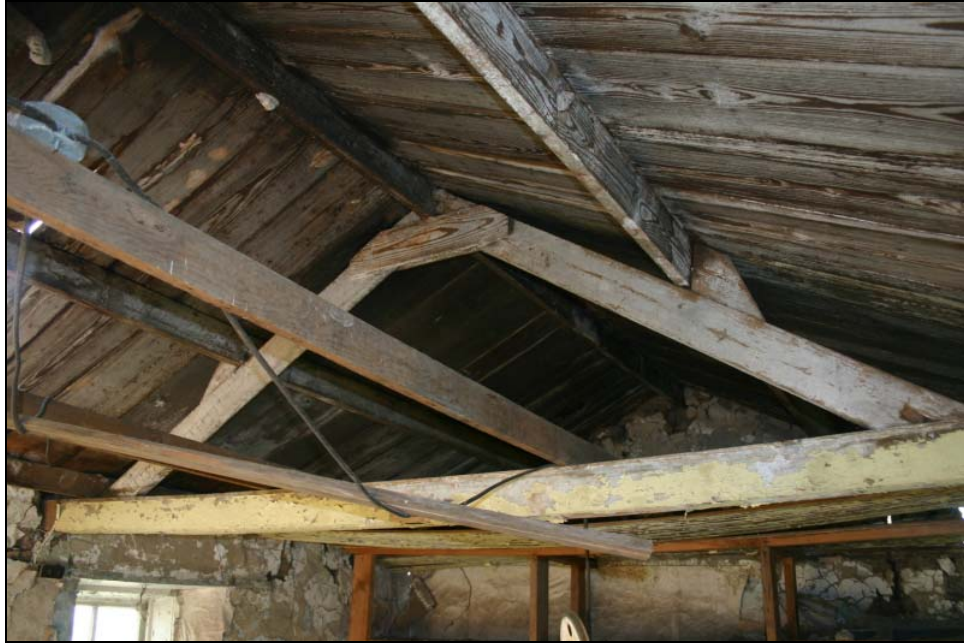
Five beam gable roof with frameless sheathing and later supported with principle rafter roof
