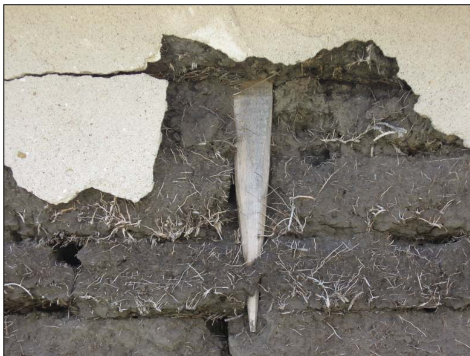
Figure 11. Wall construction: blocks laid grass side down, and sometimes included wooden stakes driven through the blocks
