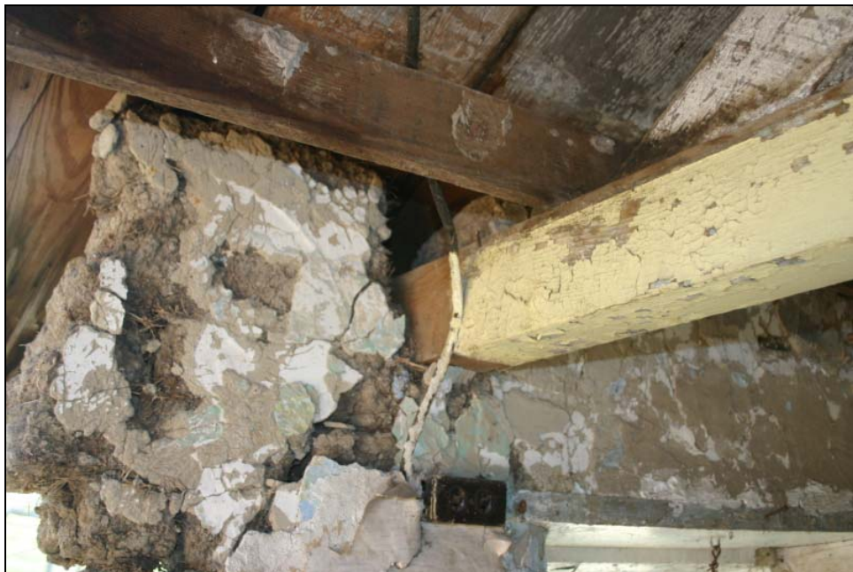
Attic joist placed directly into the sod
