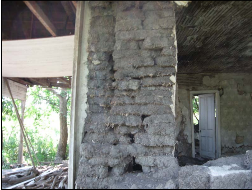
Figure 48. Sod – 12, Detail of Murray Sod House walls laid three wythes deep
