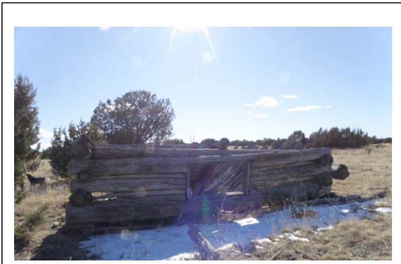
IMAGE A: Dugout with Log Superstructure
