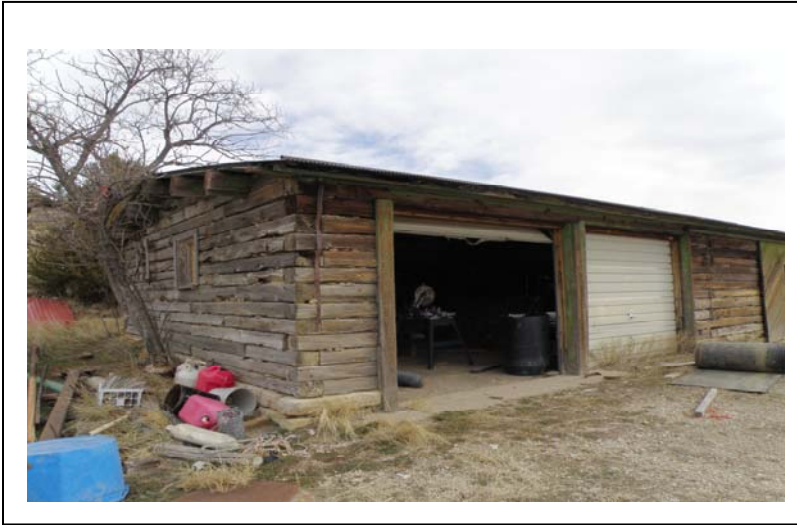
IMAGE E: Shed Constructed of Railroad Ties
