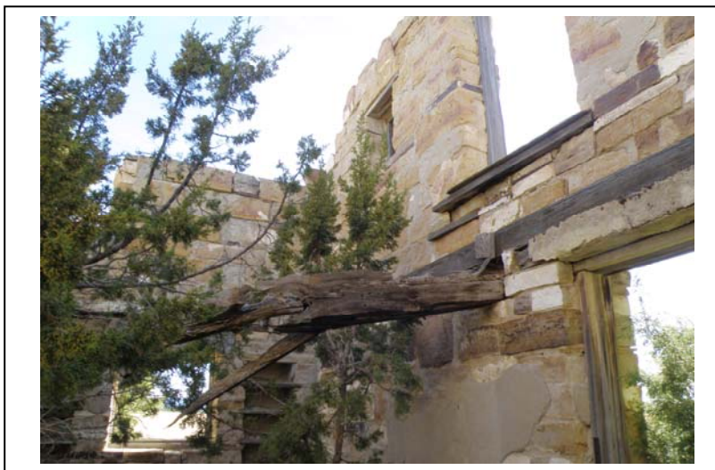
IMAGE C: Second Story Floor Beams
