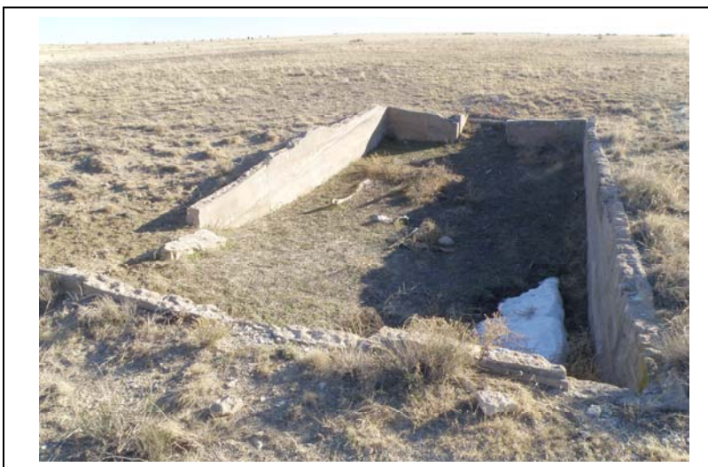
IMAGE D: Concrete-Lined Dugout
