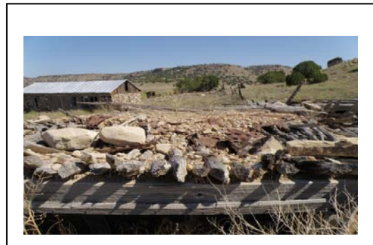
IMAGE D: Flat Roof of Vigas and Latillas
