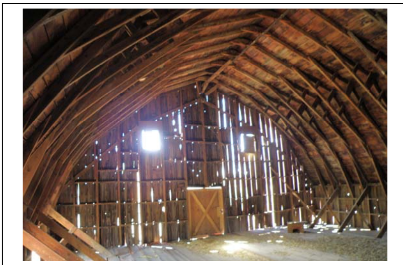
IMAGE E: Roof Truss System
