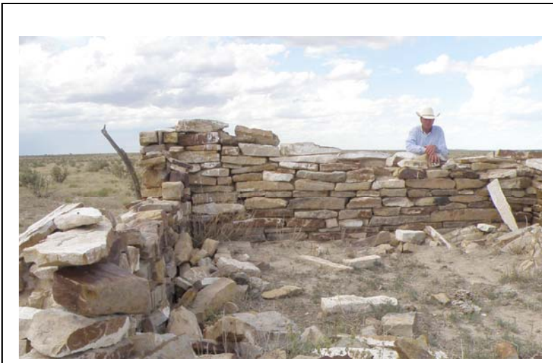
IMAGE B: Sandstone Masonry
