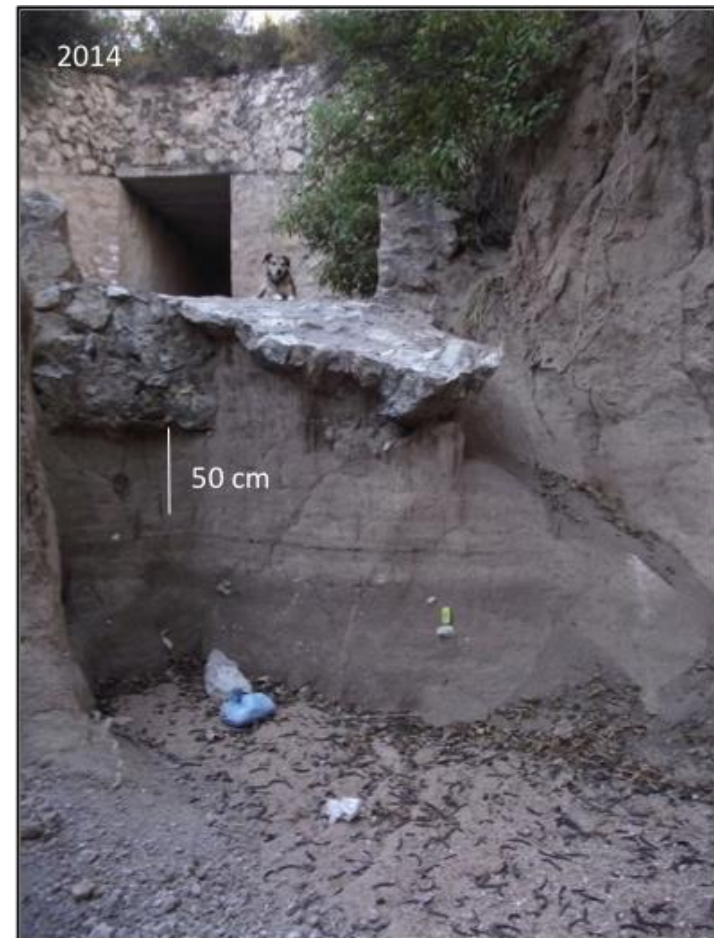
Figure 2.7. Artificial knickpoint created by a bridge on Barranca Sandage. The bridge and associated knickpoint are located immediately downstream from the basin outlet at Sandage. Figure 2.7a shows the incision depth in 2011, while Figure 2.7b demonstrates the amount of incision that occurred between 2011 and 2014.
