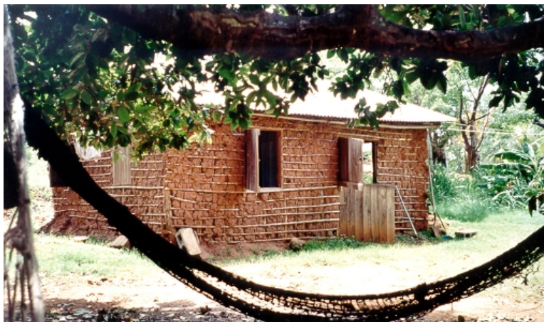
Figure 4.4 Garifuna house of traditional construction, but with metal roof
