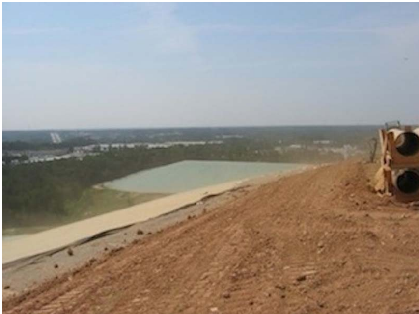
Figure 33-It is very windy on top of the landfills. This shows dust blowing off the top. You can see the non-solar TPO closure in the distance.
