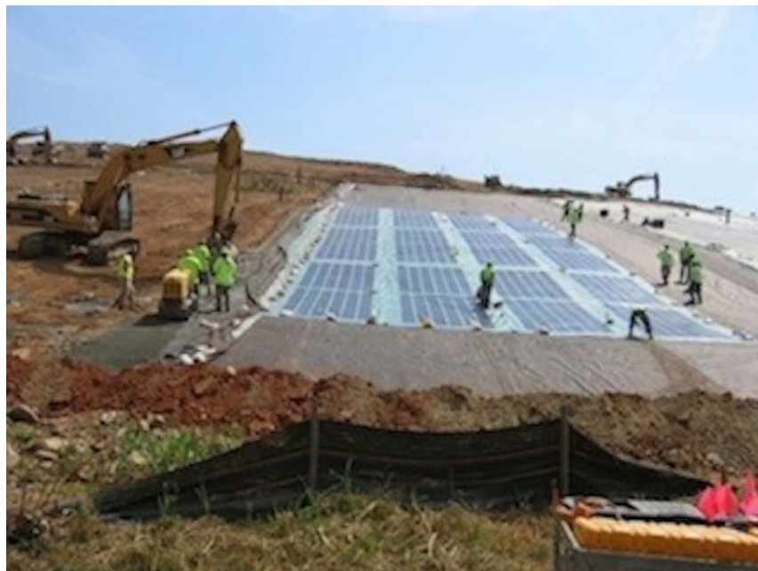
Figure 27-Workers installing the solar TPO. The machine to the left is digging a trench to tuck in the TPO so it is wind resistant.
