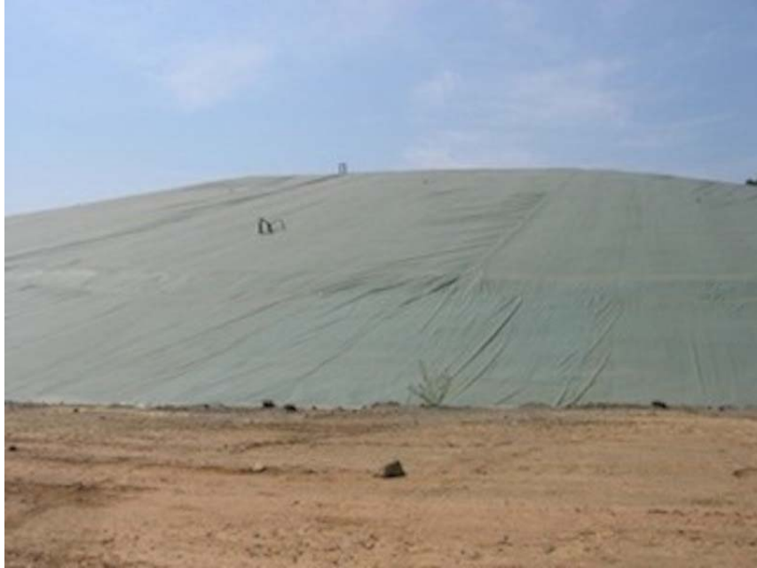
Figure 24-Another TPO closure at Hickory Ridge without solar panels. This landfill has some shading from surrounding trees making it not ideal for solar.
