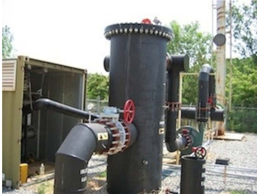
Figure 38-The LFG set-up at Hickory Ridge. The gas is currently not being used for energy. It is flared off through the flare at the rear of the photo.
