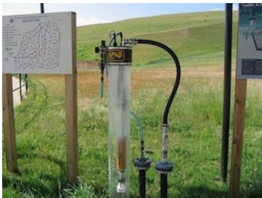
Figure 5-Example of a LFG well-head
