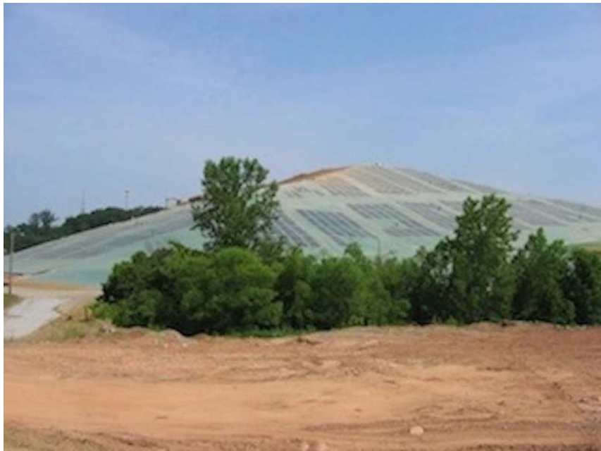
Figure 23-The installed TPO and solar panels on Hickory Ridge
