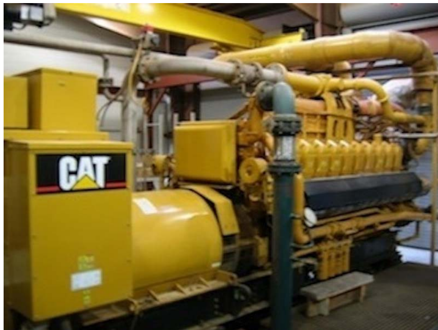
Figure 13-One of the two Caterpillar generators.
