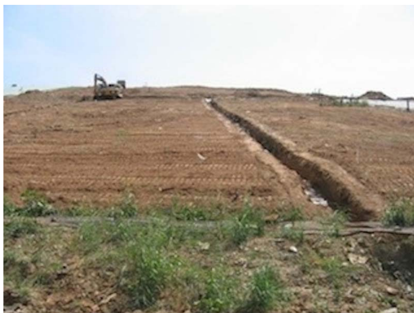
Figure 29-A trench waiting to tuck in its TPO
