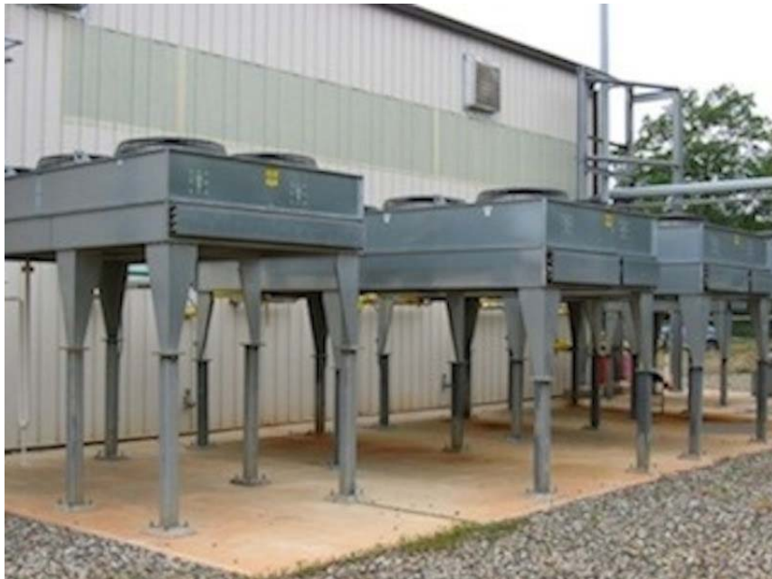
Figure 60-Cooling for the compressors
