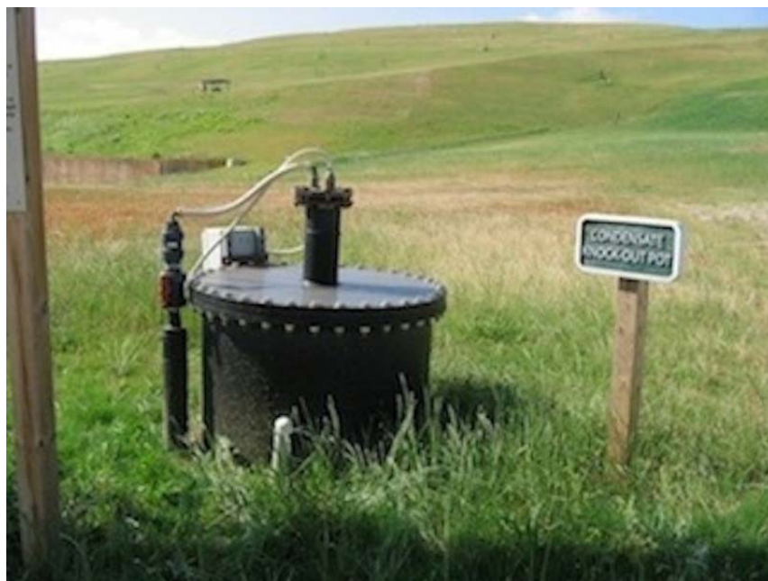
Figure 4-Example of a knockout pot where condensate is removed
