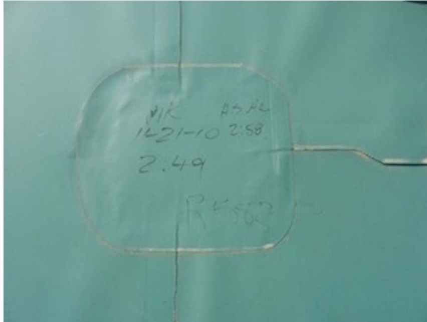
Figure 26-Each seam is signed by the installer and then signed by the person that inspects the seam.
