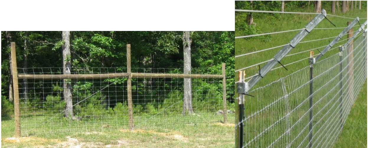
Figure 1.1. The 2.4-m woven-wire fence treatment (left) and outrigger fence treatment (right) constructed on Berry College, Floyd County, Georgia.
