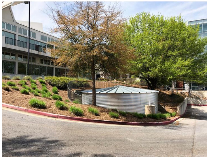
Figure 15: Jackson Street Building Above-ground Cistern
