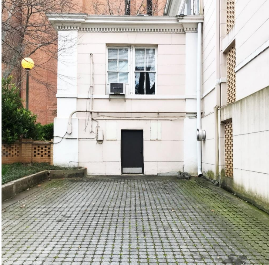
Figure 28: Site M, Pervious pavement and disconnected downspout, at Denmark Hall.
