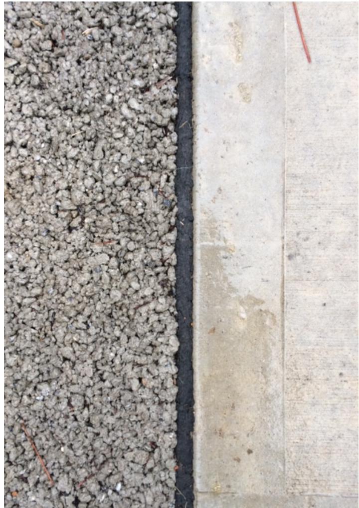
Figure 3.2: Pervious Concrete next to Traditional Concrete, Photo by Author .
