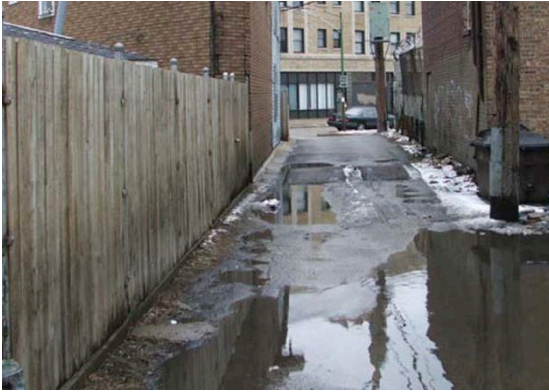
Figure 2.3: Alley with impervious pavement and poor drainage, Photo courtesy of Chicago's Green Alley Handbook
