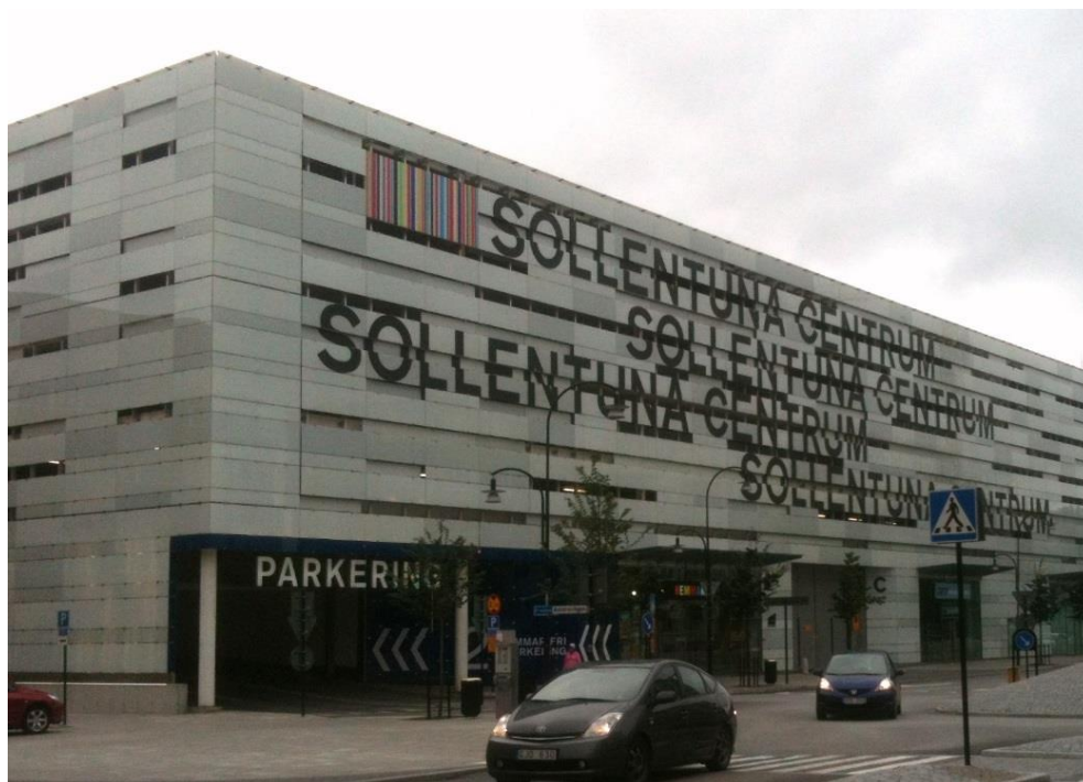
Figure 8.4 Exterior of Sollentuna Centrum. (Source: By Einarspetz - Own work, CC BY-SA 3.0, https://commons.wikimedia.org/w/index.php?curid=22790605 >).
