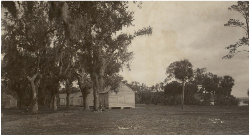
Slave cabins arranged in a double row were built at the edge of the plantation's work and wild spaces, roughly halfway between the estate house and the historic fort. The slave quarters bordered the marsh of the Skidaway River. 3
