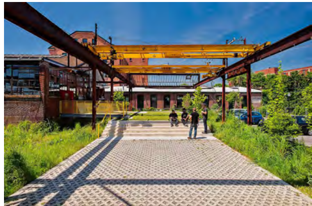
Figure 3.2: Porous Pavement (KMDG 2011)
