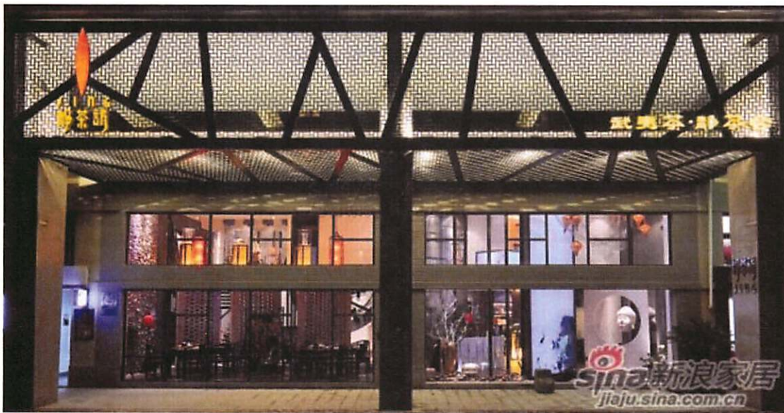
Figure40. Facade of Tranquil Tea House
