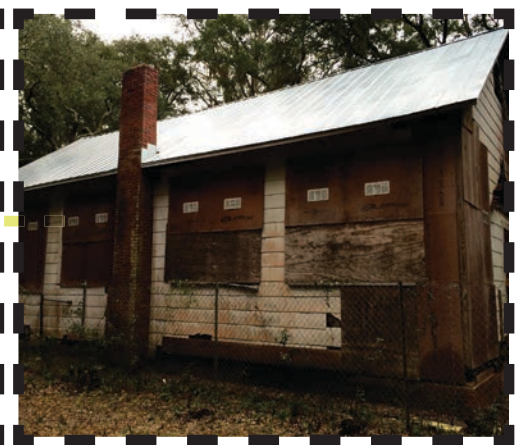
Side of Schoolhouse
