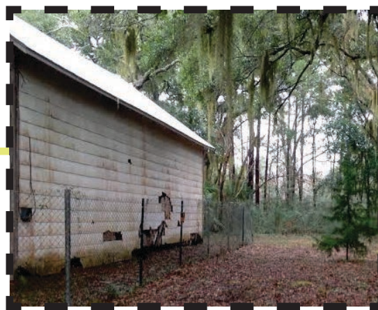
Side of Schoolhouse
