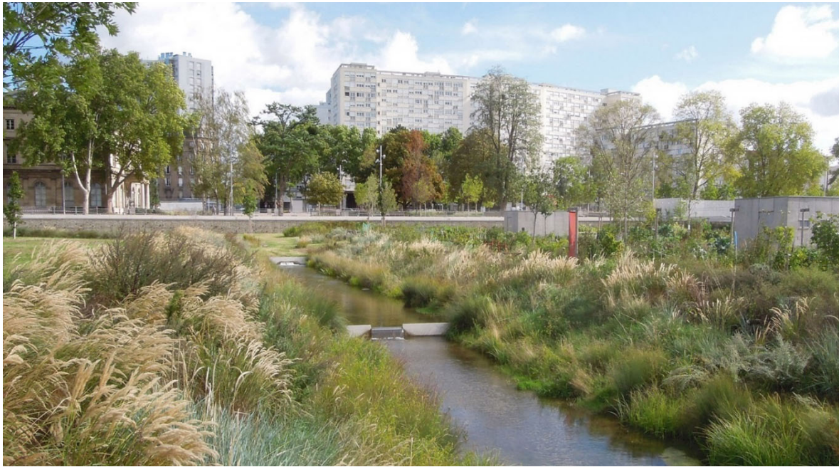
Figure 20: Vegetated bioswale for treating and storing stormwater runoff (Agence Ter)
