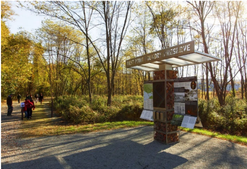
Figure 16: Gabion structure filled with bricks recovered on site (MNLA)
