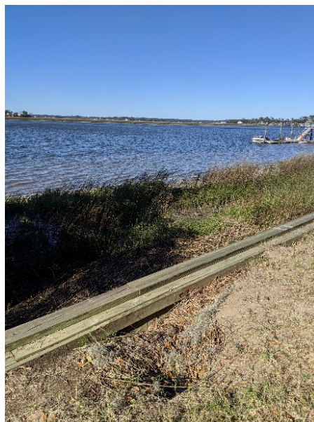
Figure 14: One of a few washout locations behind bulkhead (Jon Calabria, 02/27/2020).
