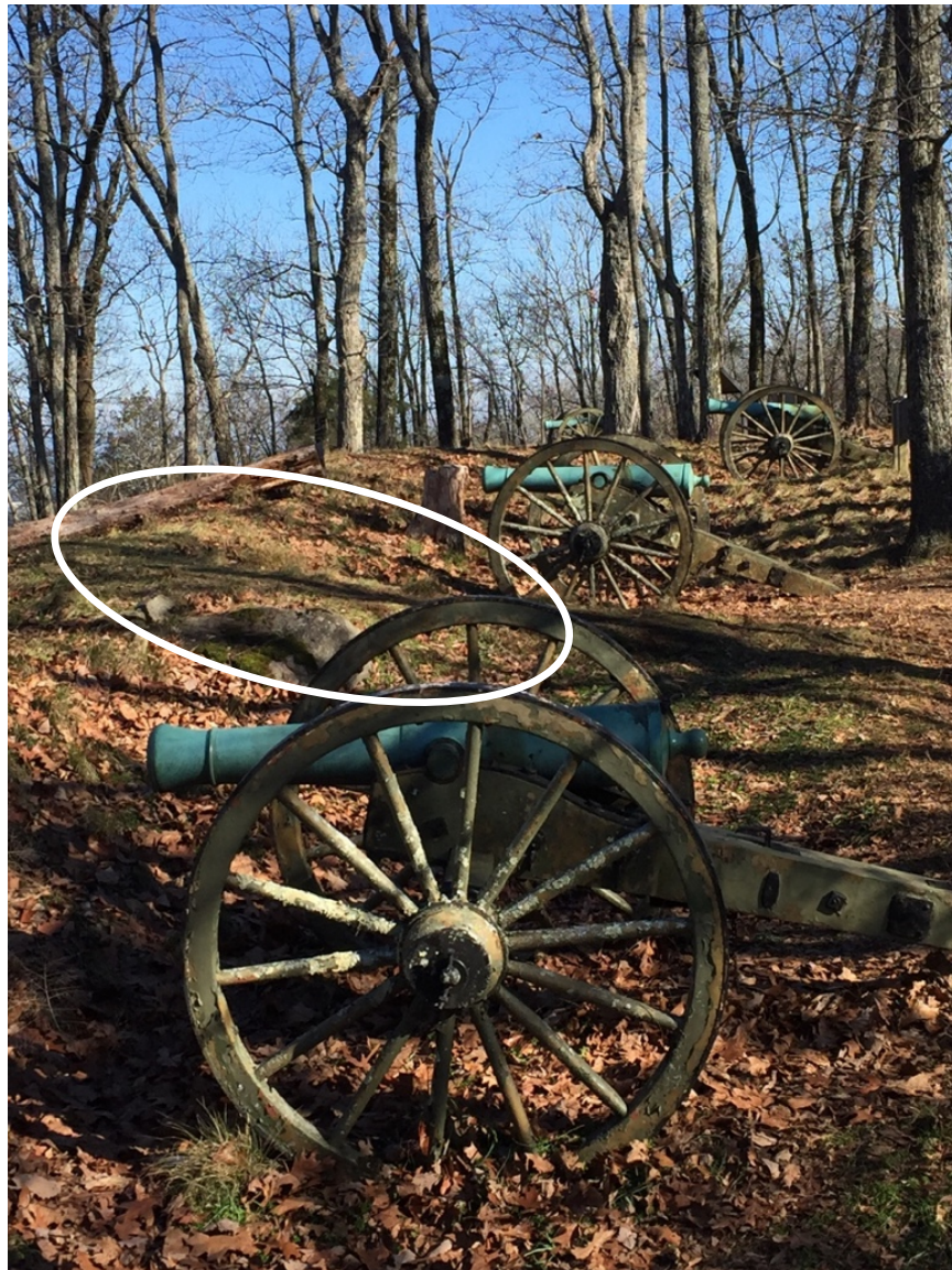
Figure 5.11. A view of the earthworks looking north. Notice the lack of leaf litter on the top of the parapet and traverse that separates the two cannons closest to the camera. Visitors are using this traverse for a walking path (Photo by Author January 2020).
