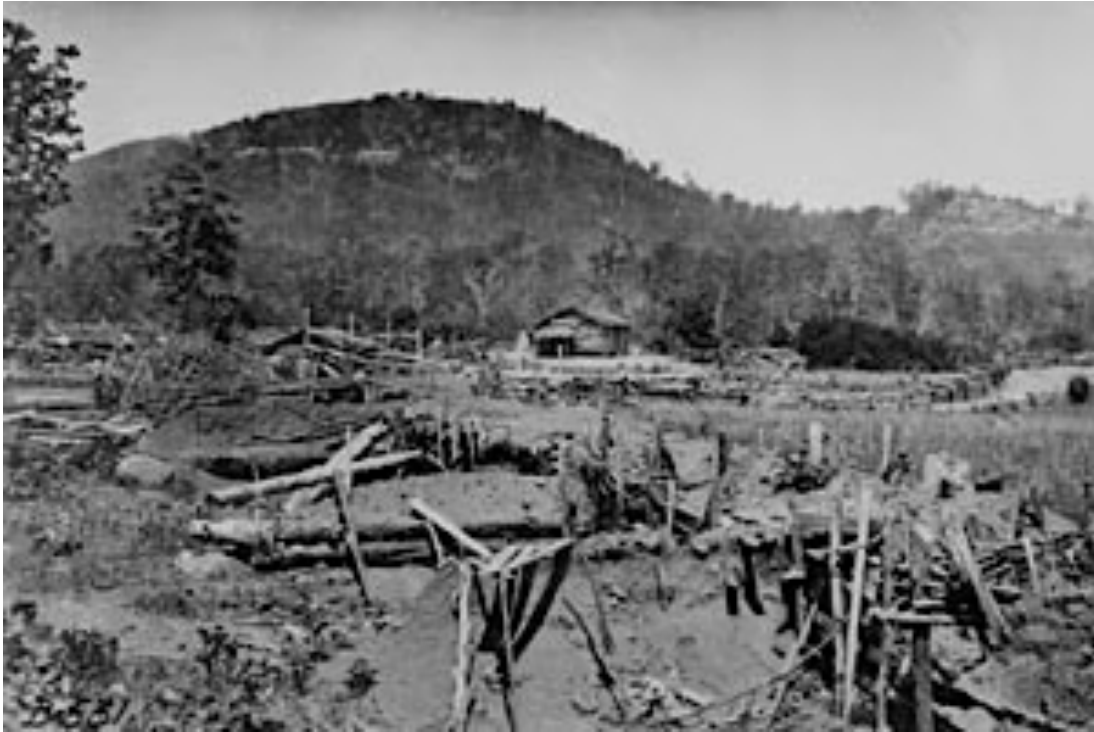
Figure 2.4. Union earthworks facing Big Kennesaw Mountain (Digital Library of Georgia).
