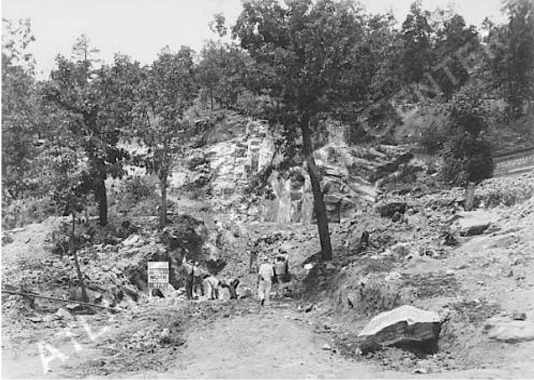
Figure 3.3. Works Progress Administration Workers quarrying rocks on Big Kennesaw Mountain for use in road construction at the park in 1935 (Digital Library of Georgia).
