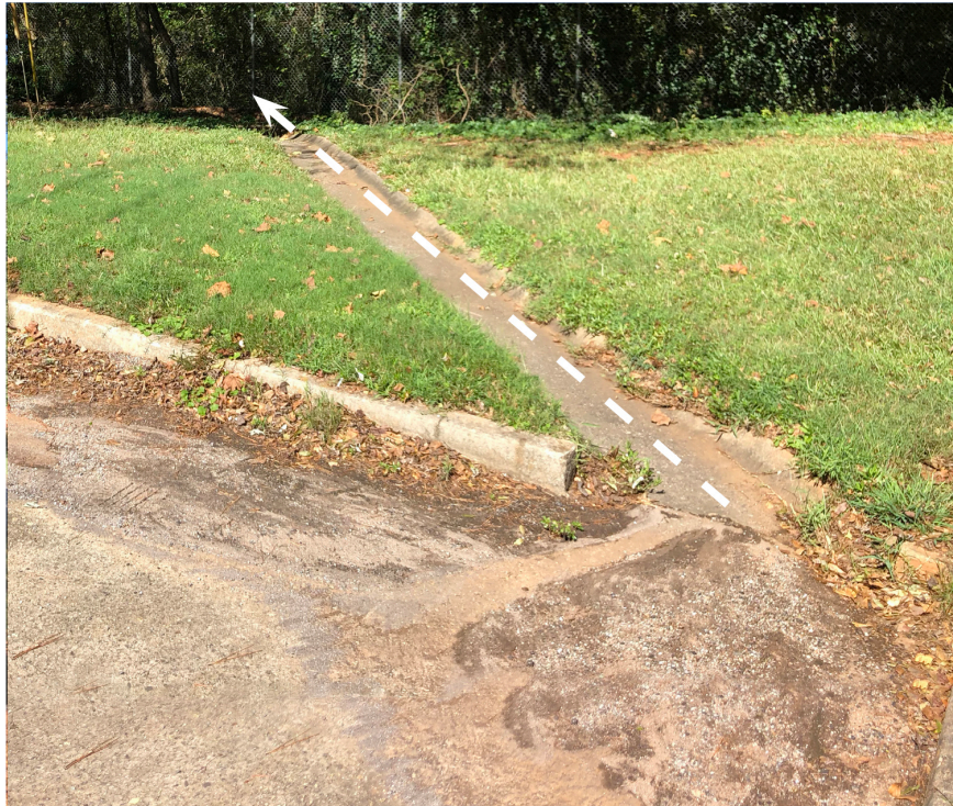
Figure 5.28. Looking toward concrete flume at Vine Circle Community. (2018)
