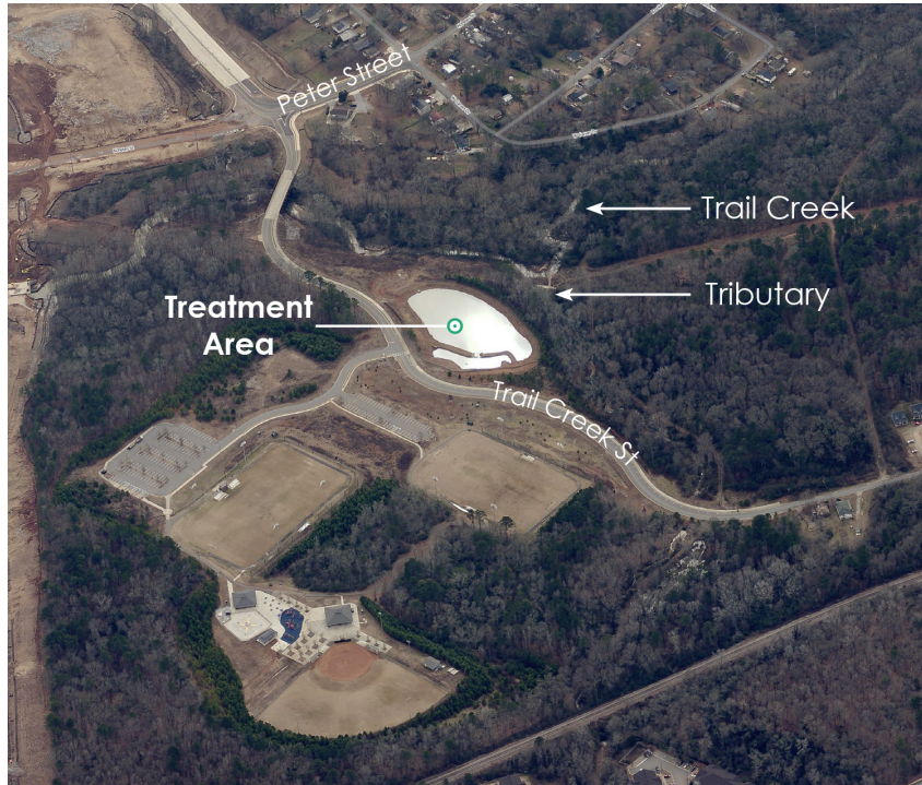
Figure 5.22. View looking south toward Trail Creek Park, Potential GI Area. Source: Pictometry 2014
