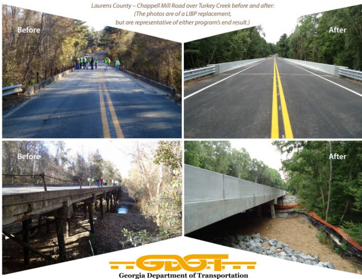
Figure 2: Results of LIBR & LOCBR in Laurens County Reprinted from Low Impact Bridge Program Manual, 2019
