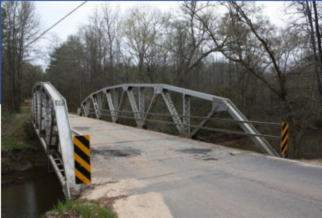
BR 25550200: Jenkinsburg Road Bridge
