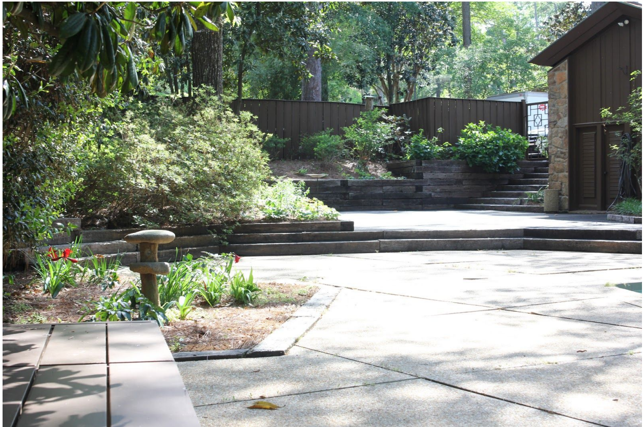
FIGURE 7 Saadia Rais, Railroad Ties Used As Steps and Retaining Wall at the Averett House , 2018, photograph.
