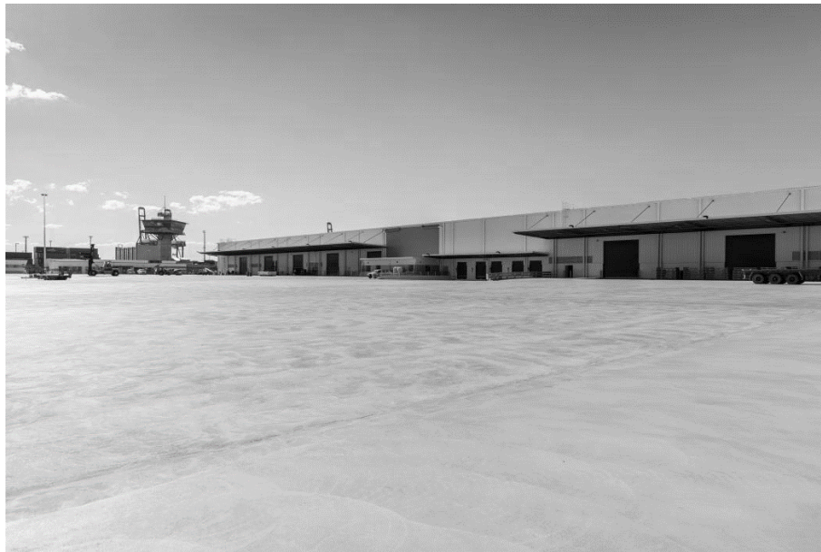
Figure 5: Seamless SFRC Slab at Port of Brisbane, Australia (ACI, 2018)
