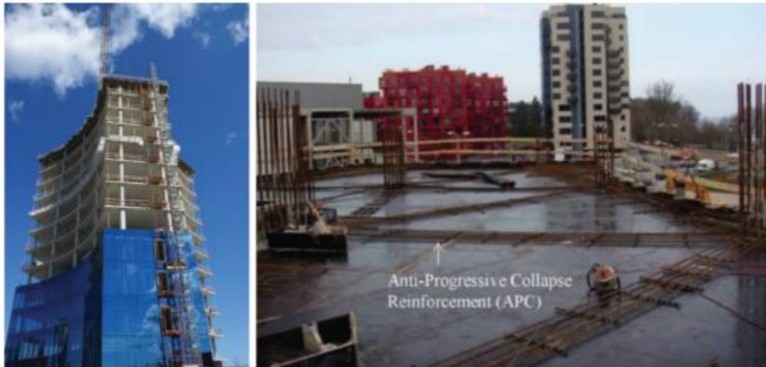
Figure 6: SFRC Elevated Slab in Highrise Construction (ACI, 2018)
