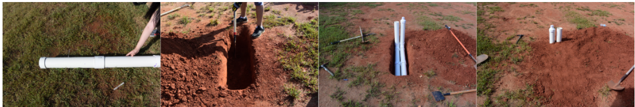
Figure 3.15: Buried Pipeline at Watkinsville, GA area.
