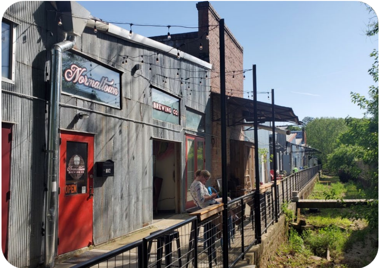
Fig. 7.6. Entrance of Normaltown Brewing Co. at Chase Park Warehouse
