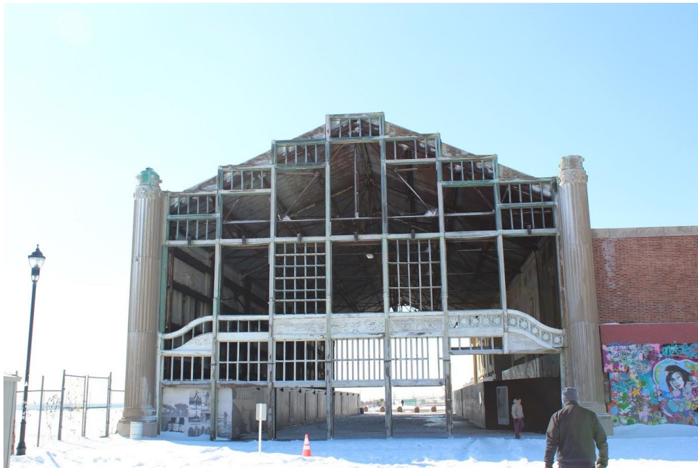
Figure 18: The Casino building, a vacant but defining, structure of the Asbury Park Boardwalk (photo by author)
