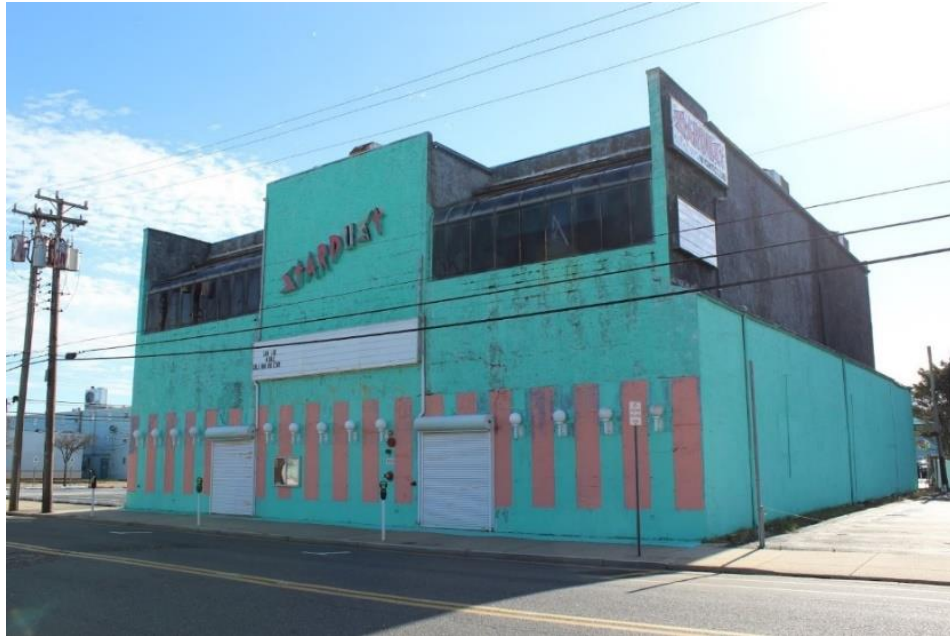
Figure 44: Known as one of the Wildwoods’ most famous night clubs, the Stardust is going to be demolished and replaced with a Comfort Inn (photo by author)
