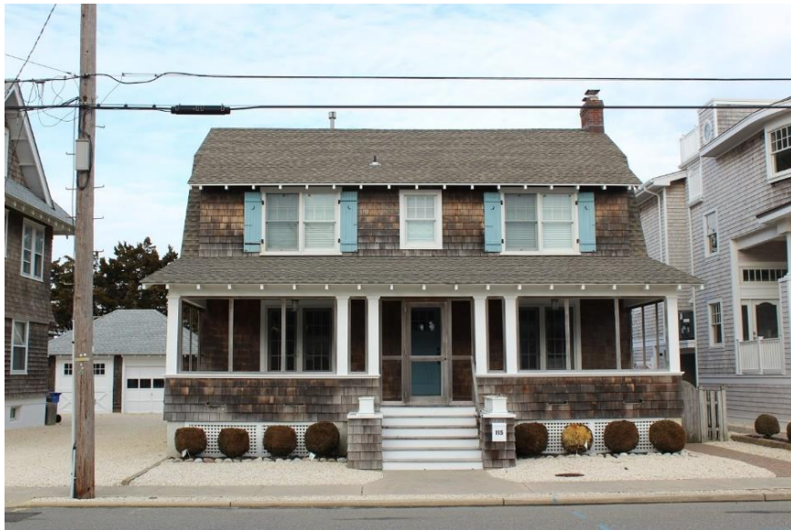
Figure 35: Shingles are frequently used on a variety of styles within the historic district, like on this Dutch Colonial house on Belvoir Avenue (photo by author)
