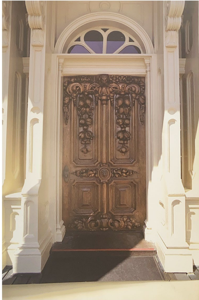
Figure 29. Woodruff House later door. Photograph 58 from Mercer University accessed March 18, 2021. https://gallery.mercer.edu/Gallery/Buildings/Macon/Woodruff-House/i-6Xbc4nM .
