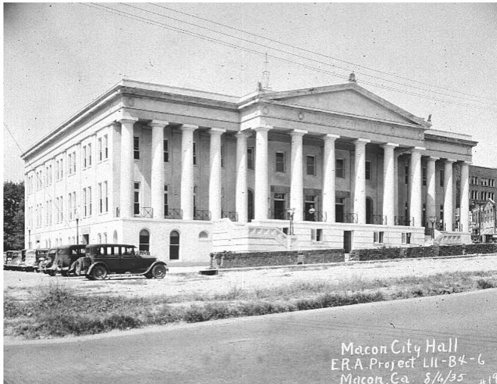
Figure 17. City Hall after 1920s renovation. Photograph from “Miscellaneous Projects.” collection file from WPA Photographs: Hargrett Rare Book & Manuscript Library. University of Georgia Libraries. Accessed March 19, 2021 at https://www.libs.uga.edu/hargrett/selections/wpa/misc/macon.html .
