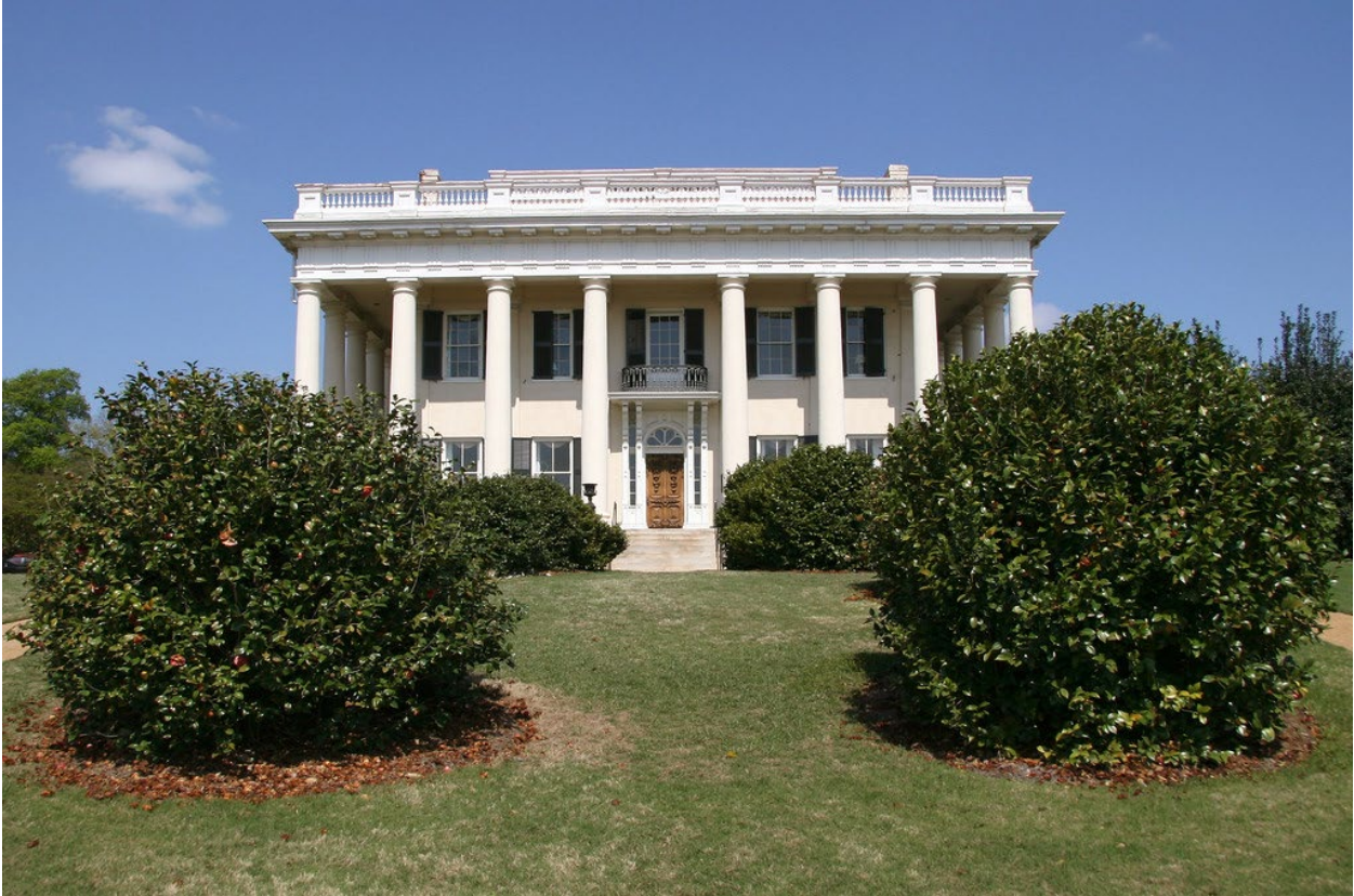
Figure 30. Woodruff House today. Photograph 56 from Mercer University accessed March 18, 2021. https://gallery.mercer.edu/Gallery/Buildings/Macon/Woodruff-House/i-6Xbc4nM .
