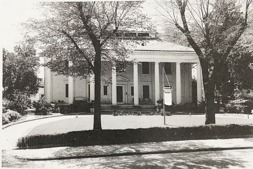
Figure 57. Nesbit House. Image 1034 Georgia Avenue, 1953 Nesbit-Wise-Winship House (demolished 1972). located at Washington Memorial Library Historical and Genealogical Room.
