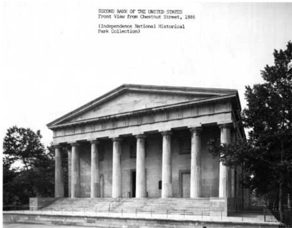
Figure 13. Second Bank of the United States. Photograph of the National Park Service entitled Second Bank of the United States, Philadelphia, Pennsylvania . Accessed at https://www.nps.gov/parkhistory/online_books/butowsky2/constitution7.htm .
