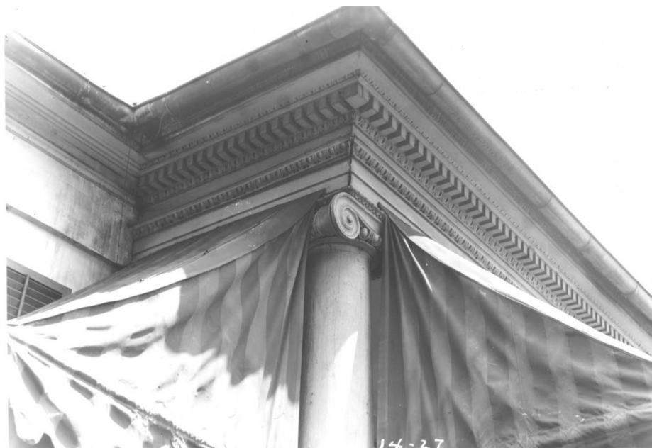
Figure 25. Portico detail on Cowles cottage. Image from National Register of Historic Places Inventory - Nomination Form. Home of Alfred Sam by John McKay Jr. United States Department of the Interior National Park Service, March 22, 1971, 9.
