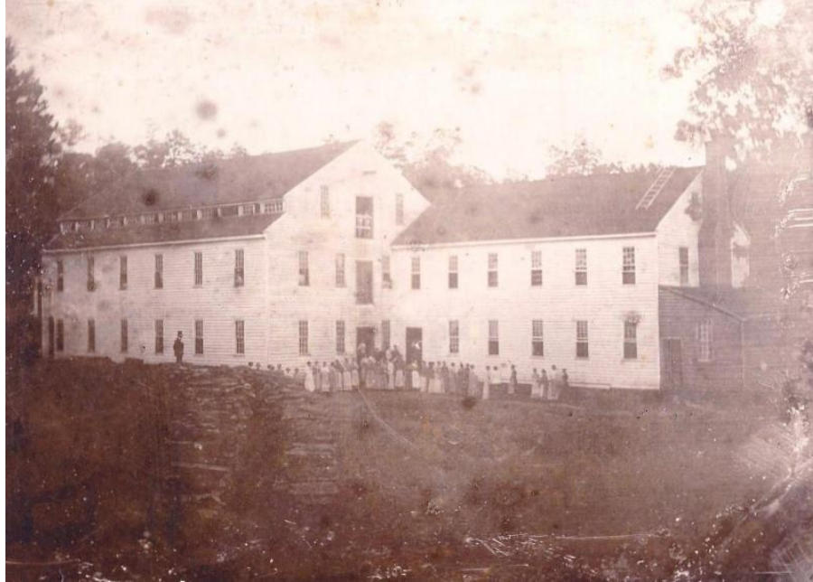
Figure 2.16. Photograph of the Alamance Cotton Mill taken shortly after its construction in 1837. Source, NCpedia.org, https://www.ncpedia.org/anchor/alamance-cotton-mill .
