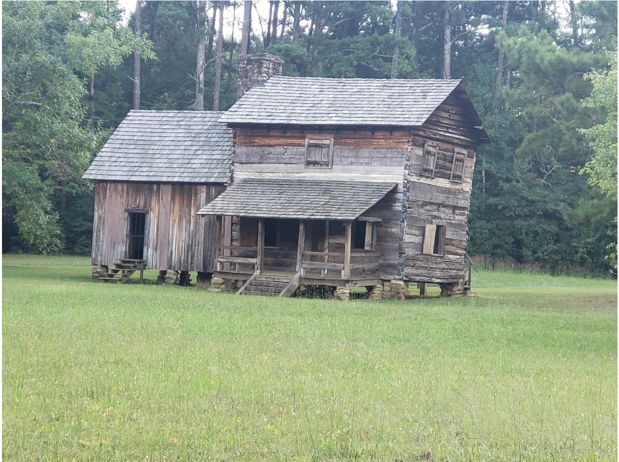
Figure 2 Relocated and Restored Vann Tavern (photo by the author)
