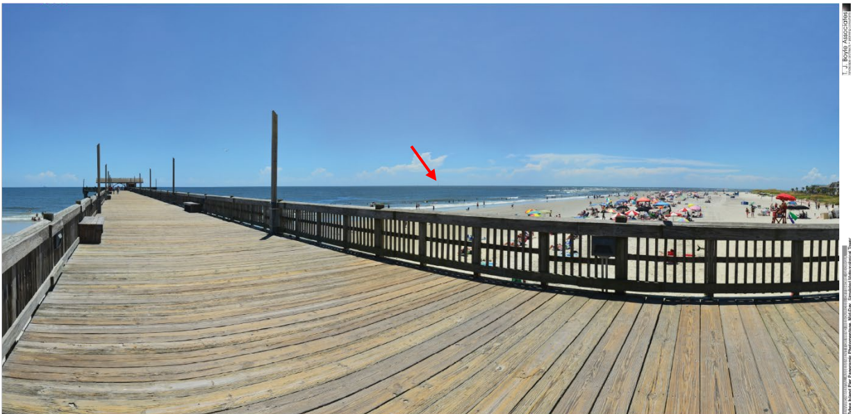
Figure 4.3. Poster of the meteorological tower as seen from Tybee Island shown during BOEM’s open house sessions in 2014. The red arrow is added to indicate the tower’s location.
