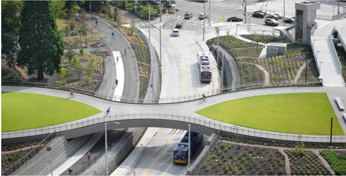
Figure 3.19 Land Bridge supports intermodal transportation
