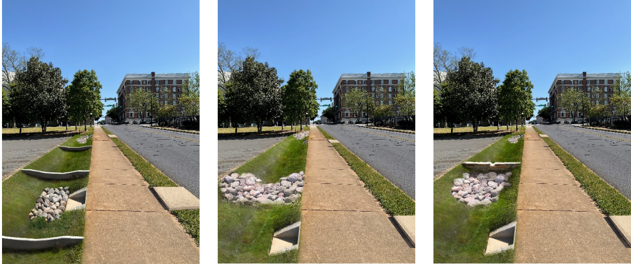
Figure 5. Images with Concrete, Stone, and Masonry Check dam, respectively
