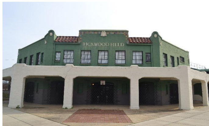
Fig. #67 – Photo of front entry portal 222
