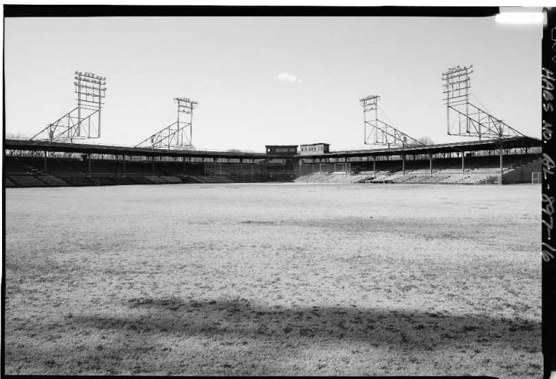
Fig. #68 - View from the outfield in 1993 from HABS documentation: 223
