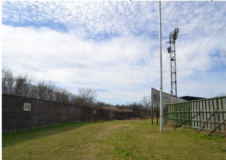
Fig. #52 – Fencing, billboards, light stanchion, and flagpole 193
