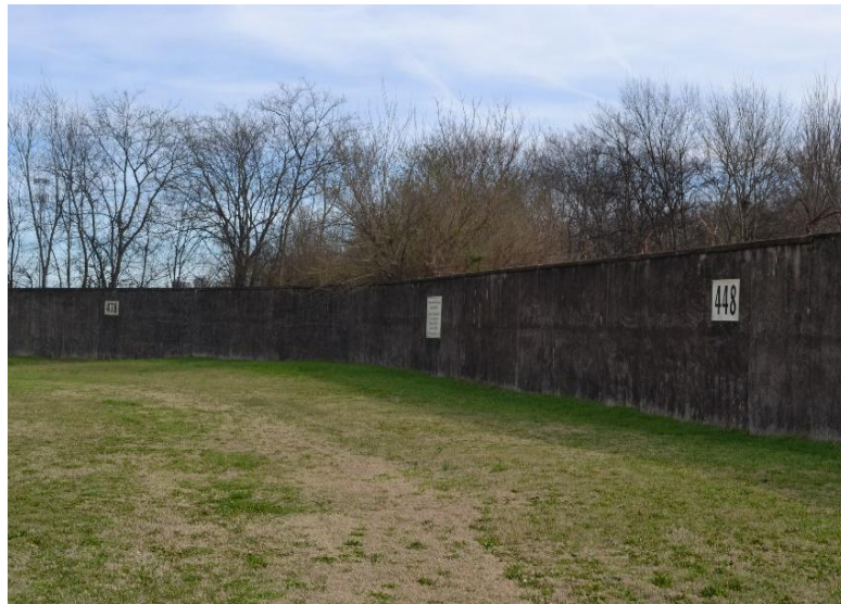
Fig. #61 – Original outfield wall 203
