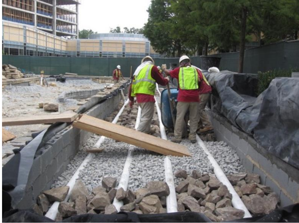
Figure 11. Installation of Filter Media (Photo taken by Reid Ferrero 2013)
