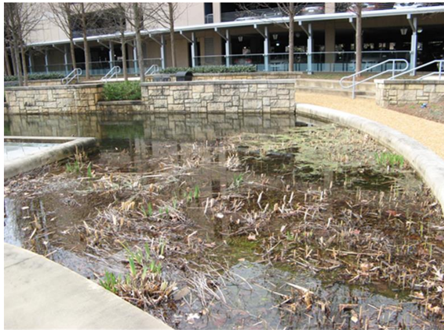
Figure 4. Photo of Existing Conditions (HGOR 2012)
