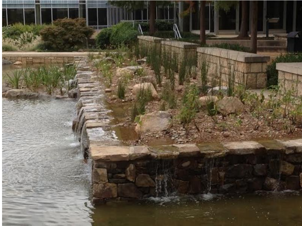
Figure 15. Photo of Pump Start Up (Photo taken by Reid Ferrero 2013)
