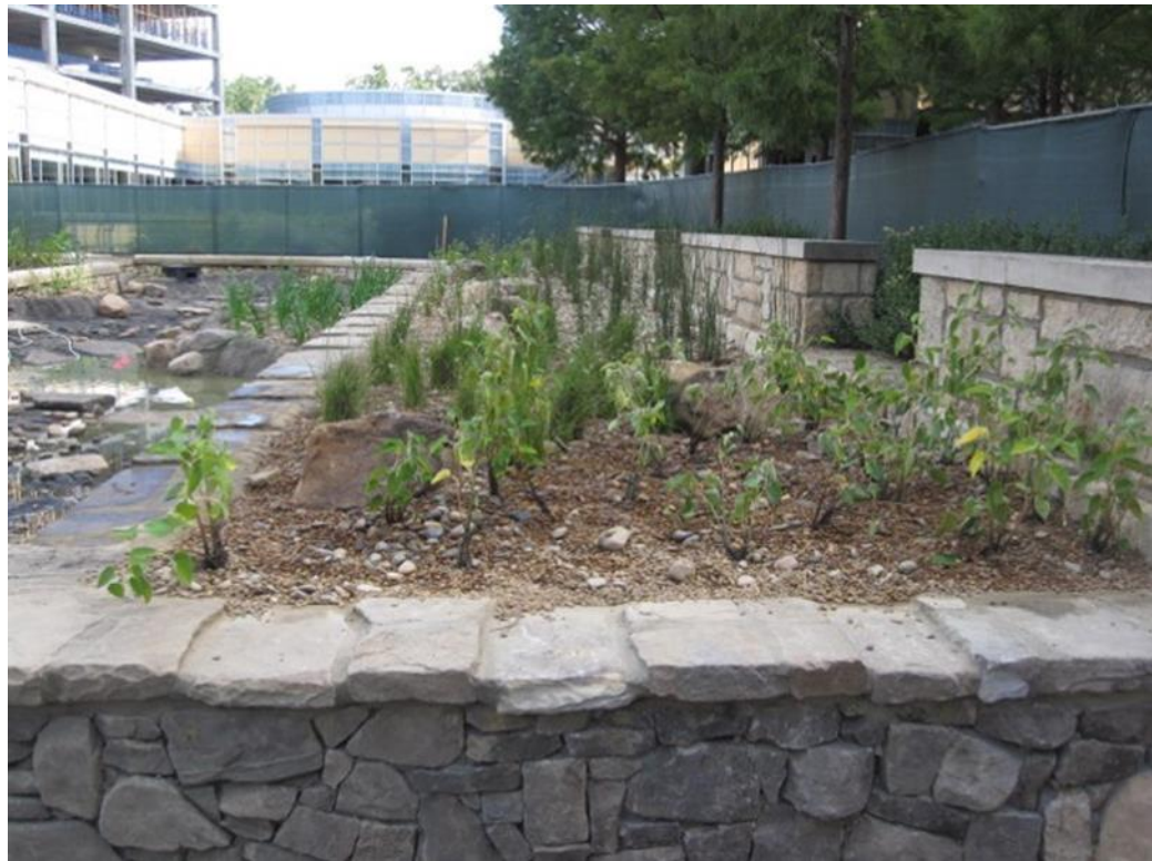
Figure 14. Installation of Plant Material (Photo taken by Reid Ferrero 2013)
