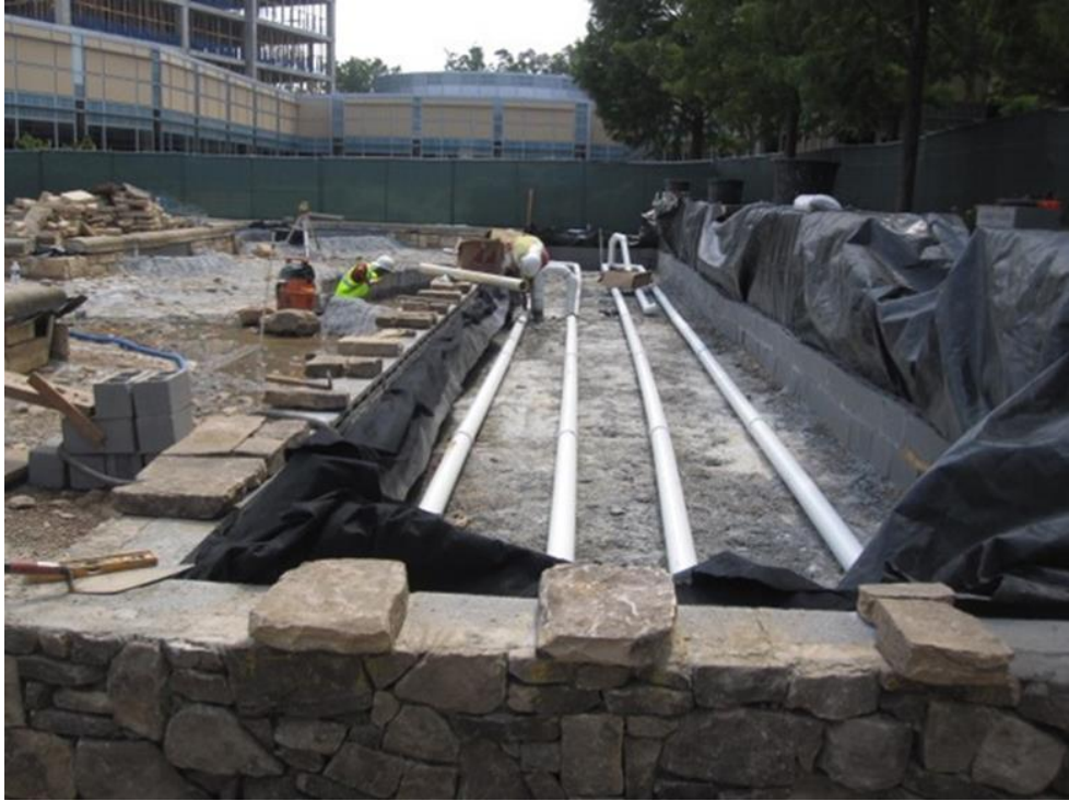
Figure 10. Installation of Dispersion Pipe (Photo taken by Reid Ferrero 2013)
