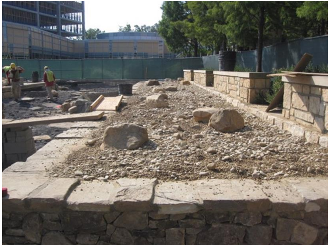
Figure 13. Installation of Filter Top Dressing (Photo by Reid Ferrero 2013)
