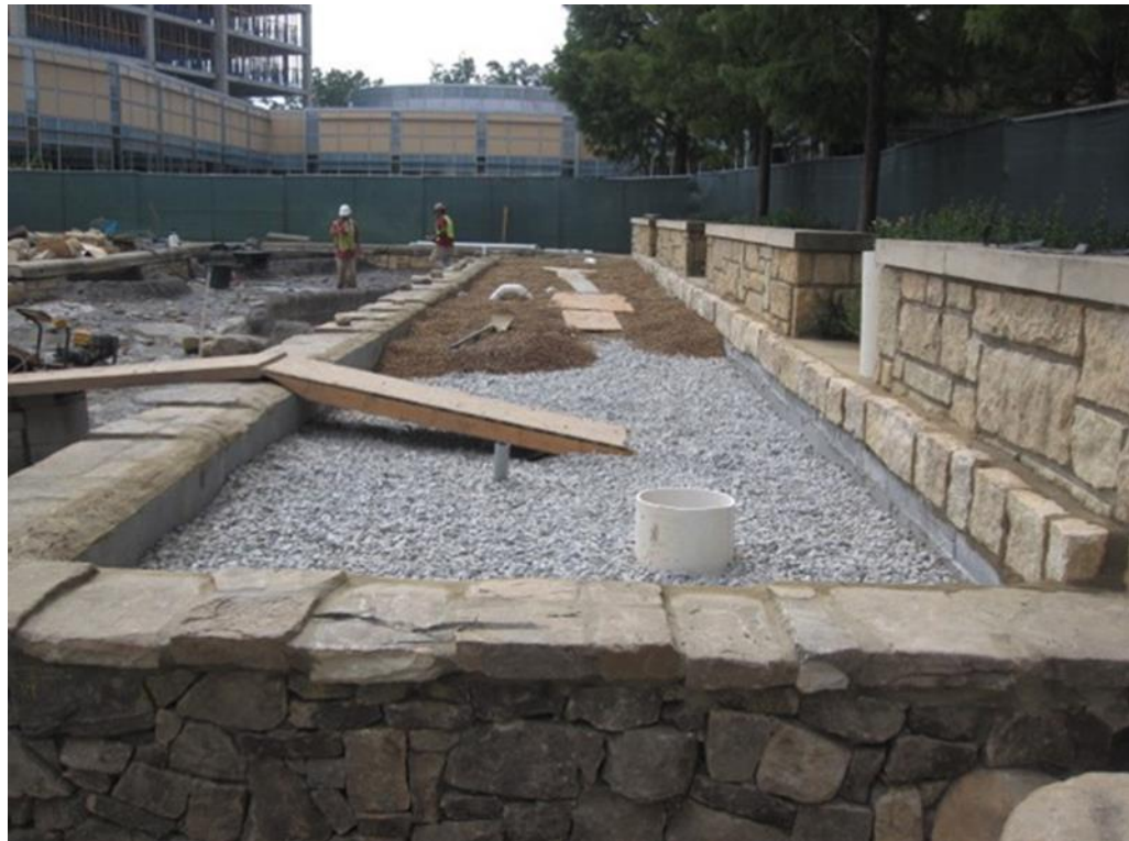
Figure 12. Installation of Filter Media (Photo taken by Reid Ferrero 2013)
