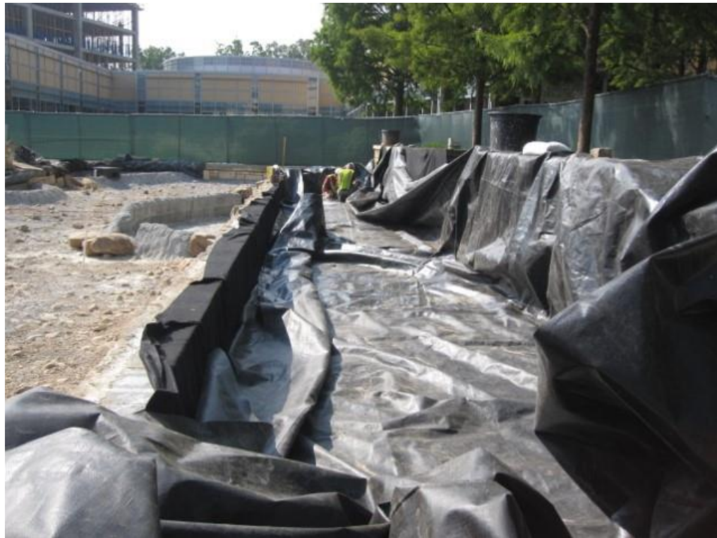
Figure 8. Waterproofing installation (Photo taken by Reid Ferrero 2013)
