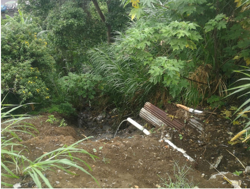
Figure 3.12: Sewage falling directly into LC GPS. Source: Felipe Barrantes.
