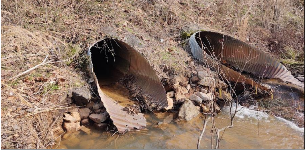
Figure 44 – Outlet of Voyles Road Double Barrel Culvert
