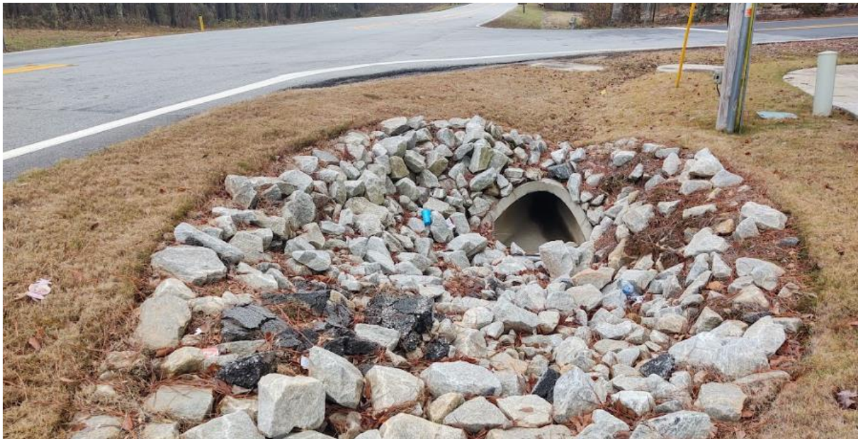
Figure 67 - Asset #3 Flair-End Concrete Culvert with Corrugated Pipe Barrel Under Major Road
