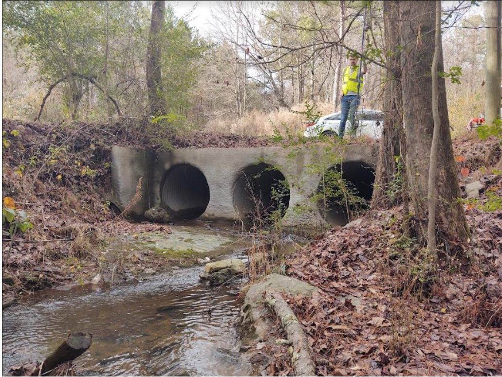
Figure 66 - Asset #2 Culvert Box Containing Three Lined Corrugated Pipes over Creek
