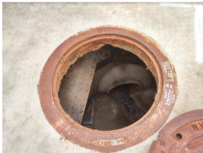
Figure 65 - Asset #1 Reinforced Concrete Stormwater Drainage Pipe in Residential Subdivision
