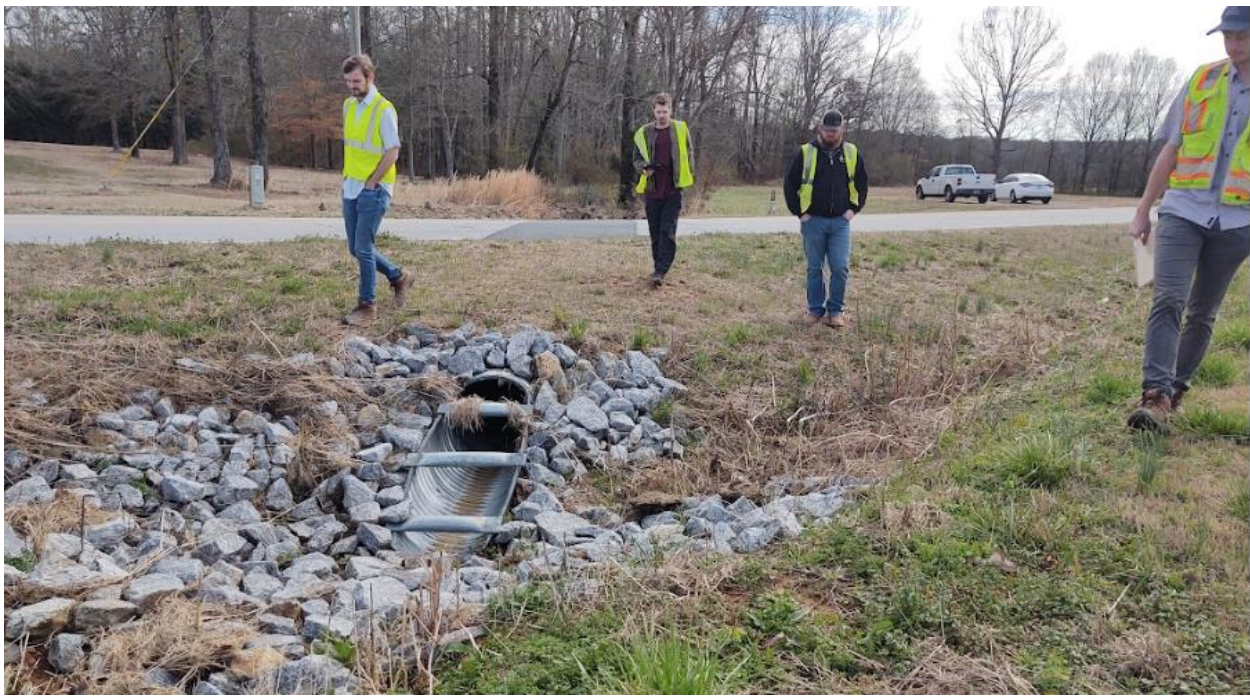
Figure 46 – Newly Installed Plastic Cross-Road Pipe Asset
