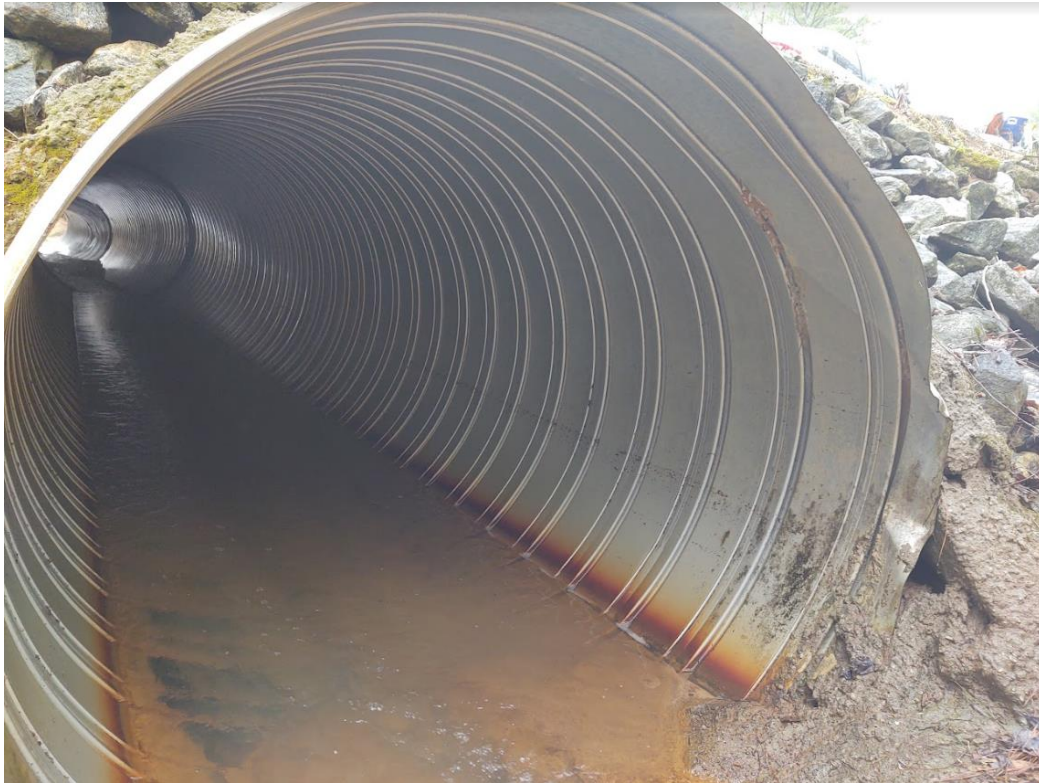
Figure 33 – Interior of Asset #4 with Sealant Holding Sleeve in Place
