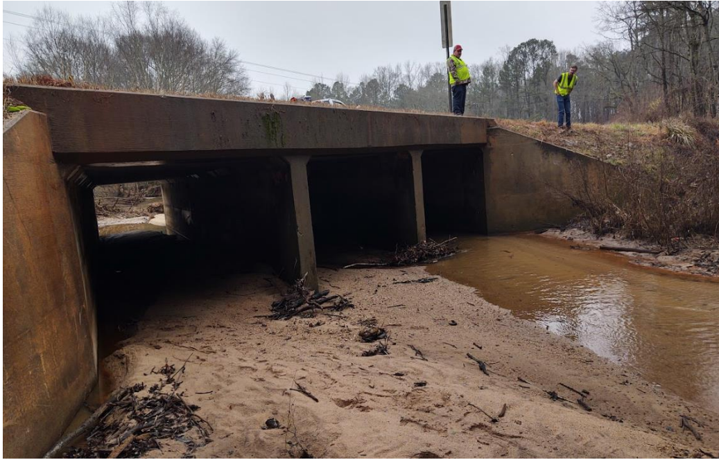
Figure 31 – Asset #3: Large Reinforced Concrete Box Culvert
