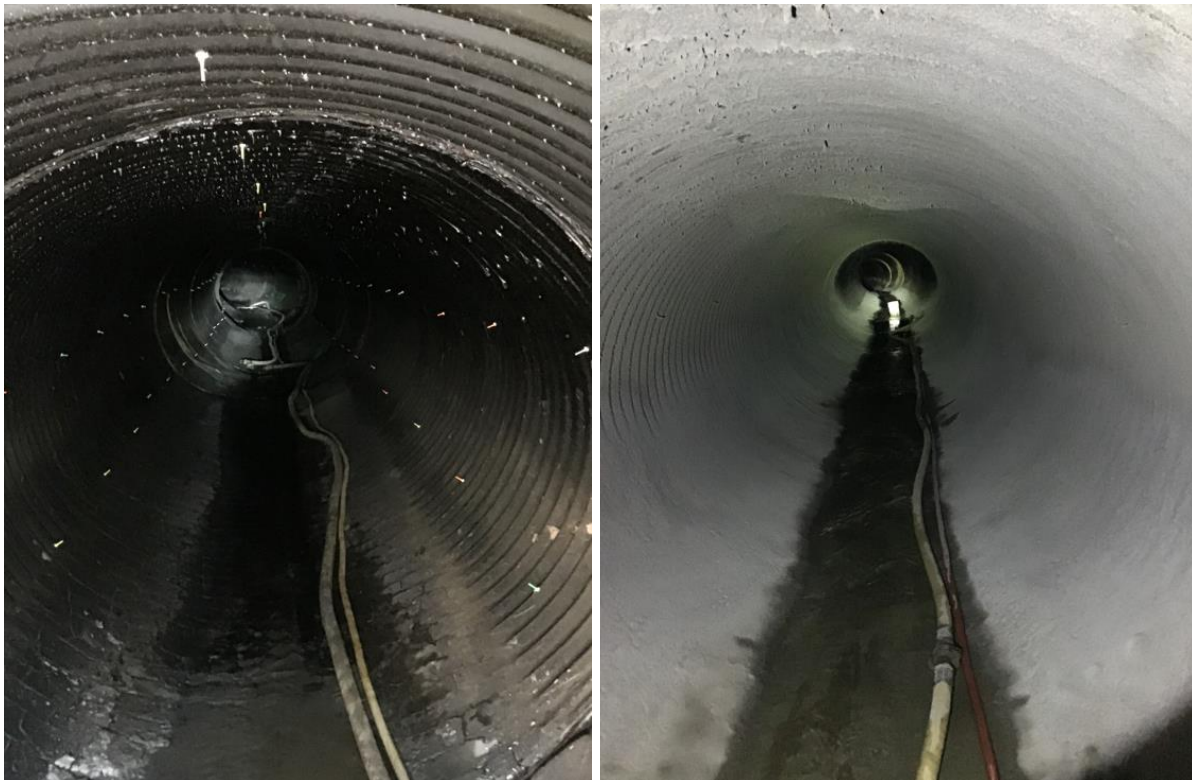
Figure 40 – Before and After of Geopolymer Lining Pipe Rehabilitation.
