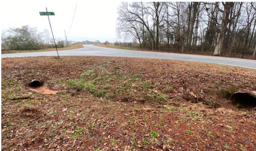
Figure 27 – Asset #1 Prior to Earthwork Maintenance
