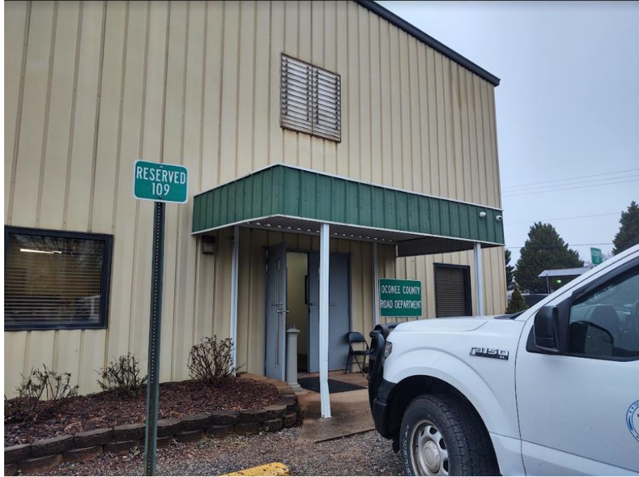
Figure 19 - Front Face of the Oconee County Road Department Building
