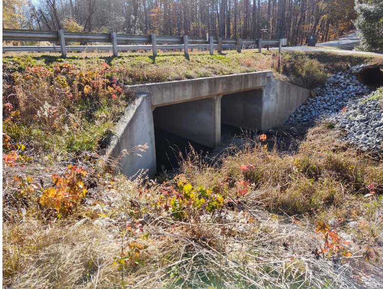
Figure 52 - Large Concrete Culvert Located on Lees Mill Road
