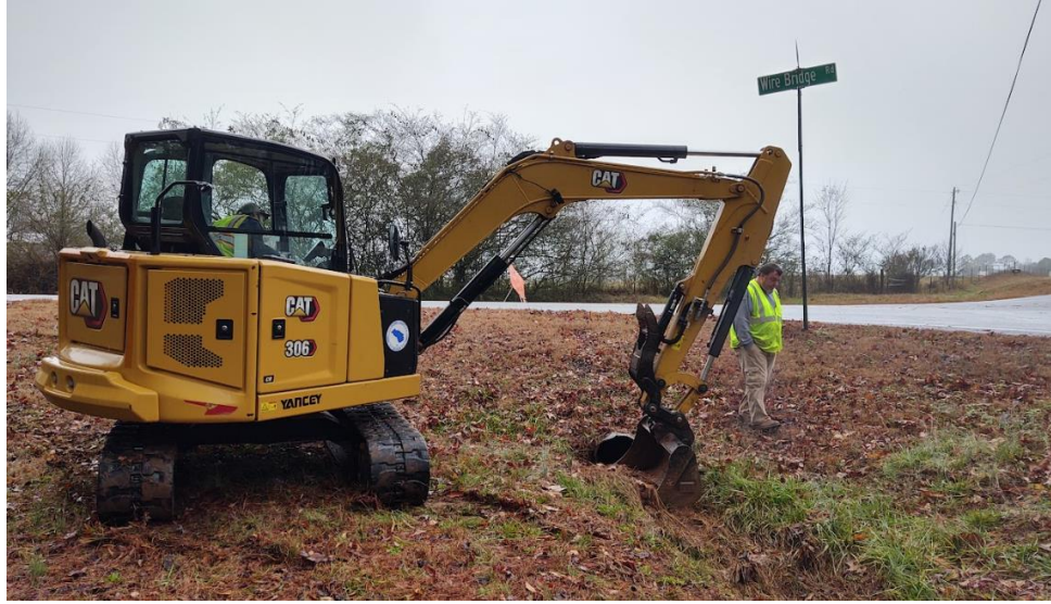
Figure 25 – Excavator Used for Earthwork Necessary in Asset Maintenance
