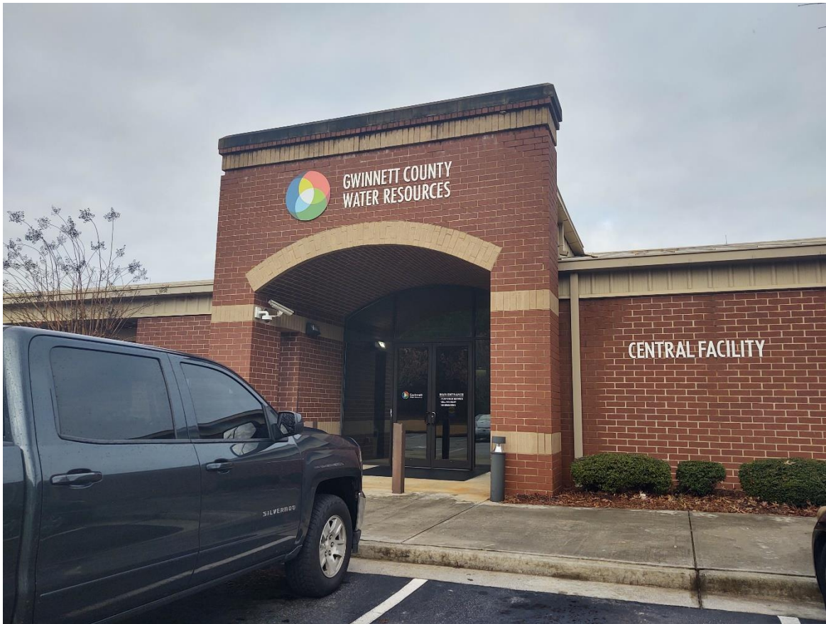
Figure 55 - Front Face of the Gwinnett County Water Resources Department Building
