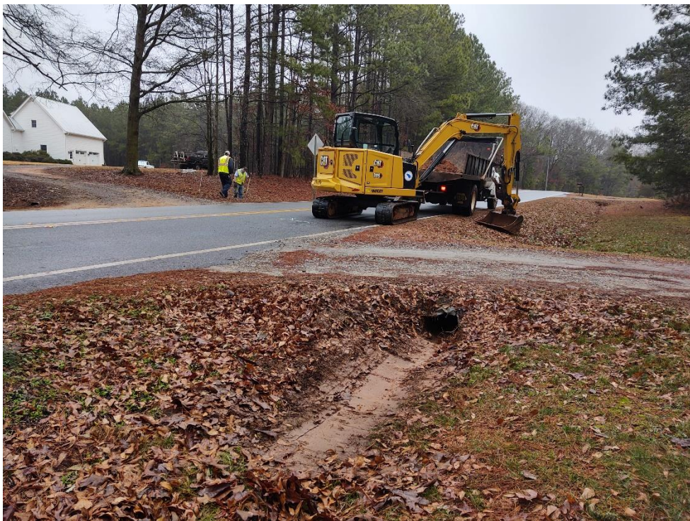
Figure 29 – Maintenance on Driveway Culverts
