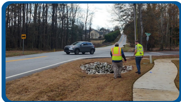
Figure 6 - Inspectors Minding Traffic Hazards and Standing a Safe Distance Away.
