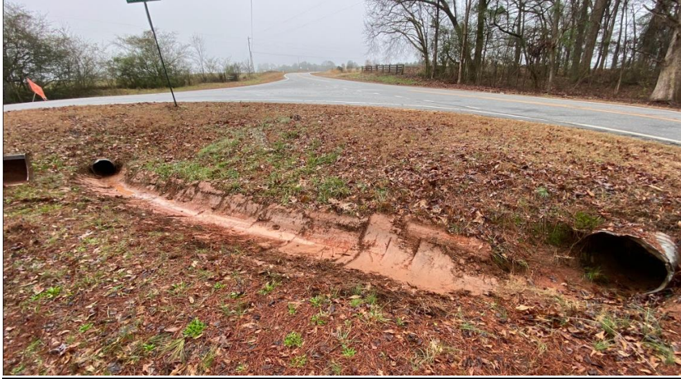
Figure 28 – Asset #1 After Earthwork Maintenance
