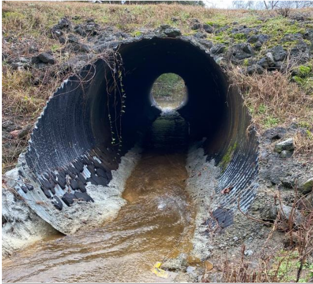
Figure 30 – Asset #2: Large Corrugated Metal Pipe Asset with Concrete Bottom Lining
