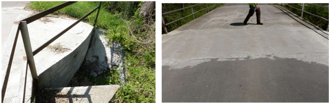
Figure 45: Bridge 055-5009-0 Void Repair Side View(Left) and Top View (Right)
