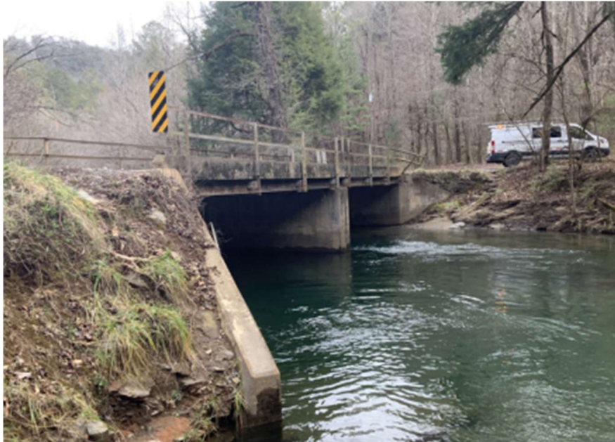
Figure 193 – Bridge 213-0048-0 Side View (GDOT, 2022)
