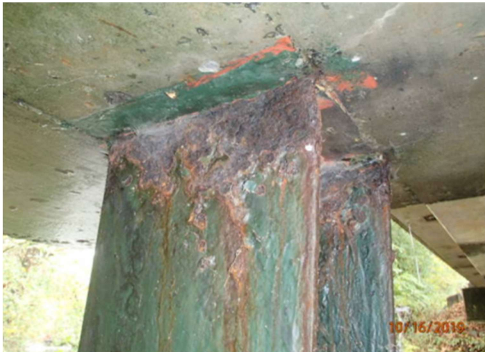
Figure 177 – Bridge 111-5002-0 Typical Steel Pile Condition (GDOT, 2019)
