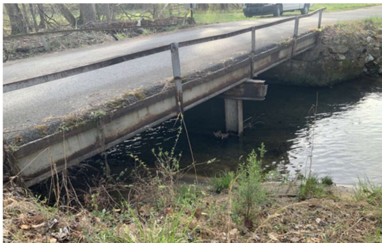
Figure 51: Bridge 055-5045-0 Right Side View (GDOT, 2020)
