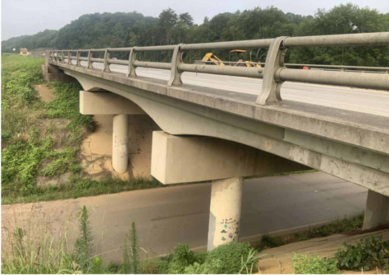
Figure 107 – Bridge 083-0027-0 Side View (GDOT, 2022)
