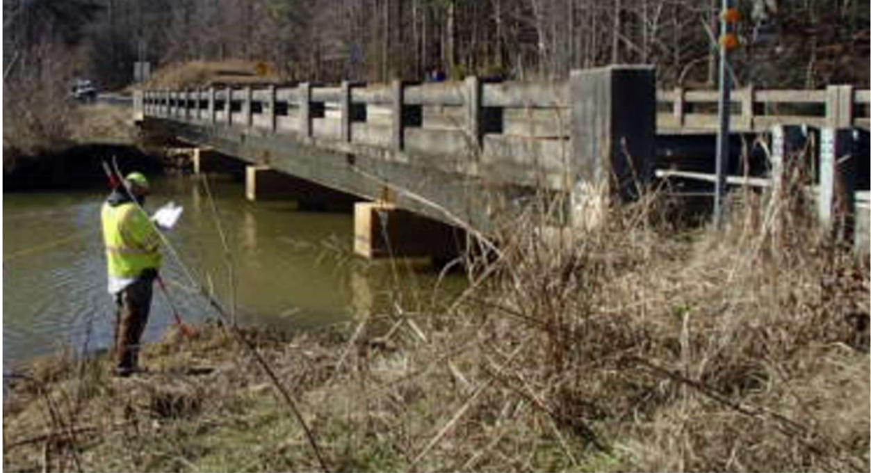
Figure 132 – Bridge 311-5001-0 Side View (GDOT, 2021)
