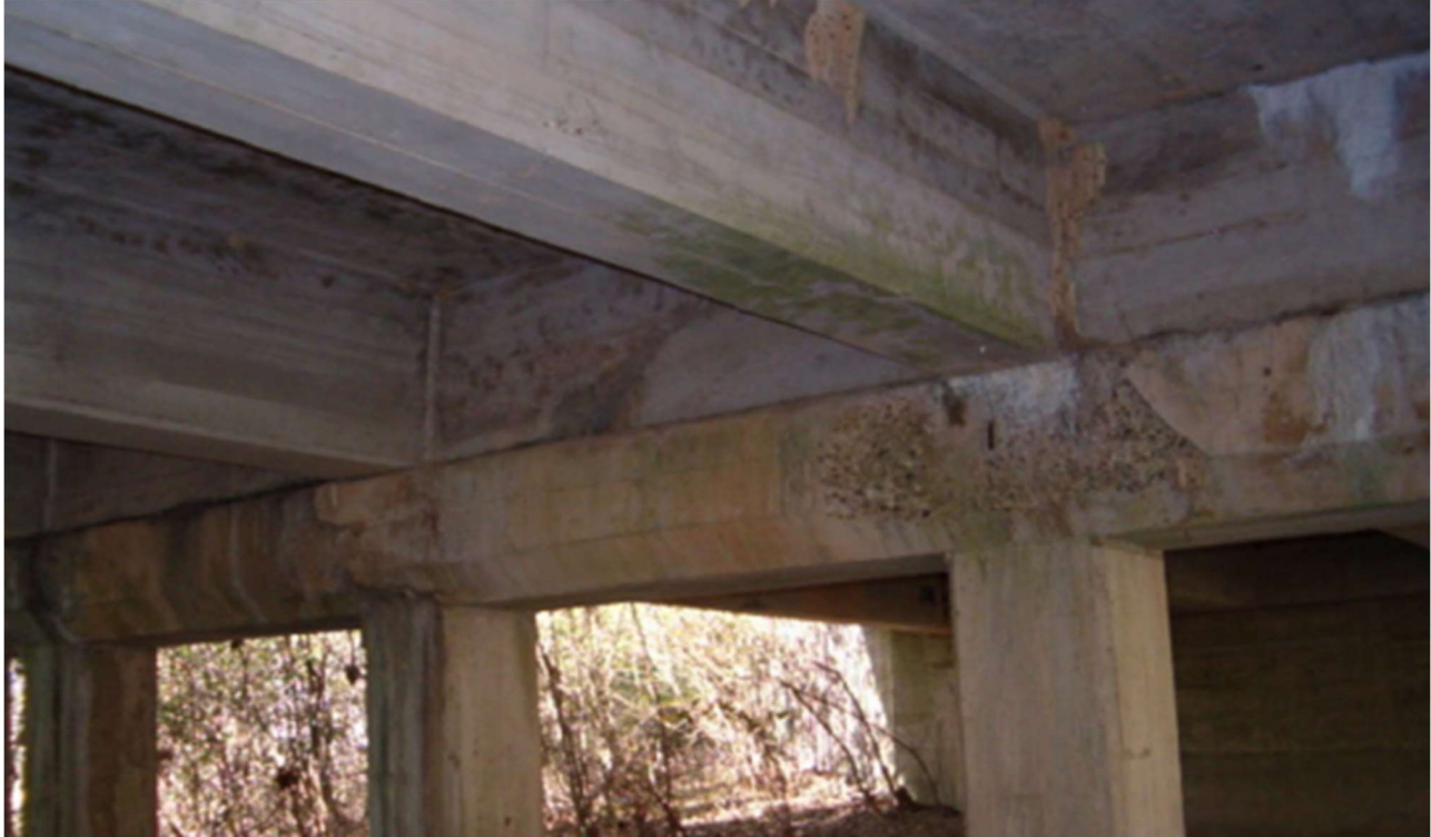
Figure 100 – Bridge 295-0041-0 Reinforced Concrete Pier Cap (GDOT, 2021)
