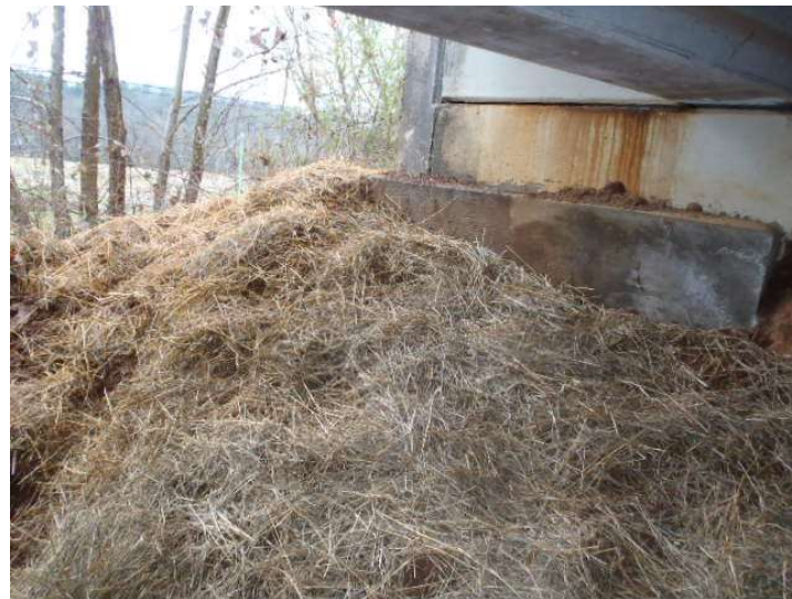
Figure 205 – Bridge 311-0040-0 Abutment Repair (GDOT, 2020)
