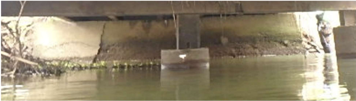
Figure 66: Reinforced Concrete Abutment on Bridge 055-5026-0 (GDOT, 2020)
