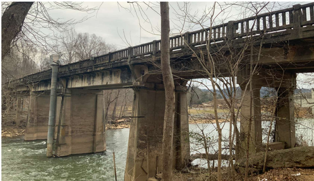
Figure 184 – Bridge 213-0044-0 Sideview (GDOT, 2022)
