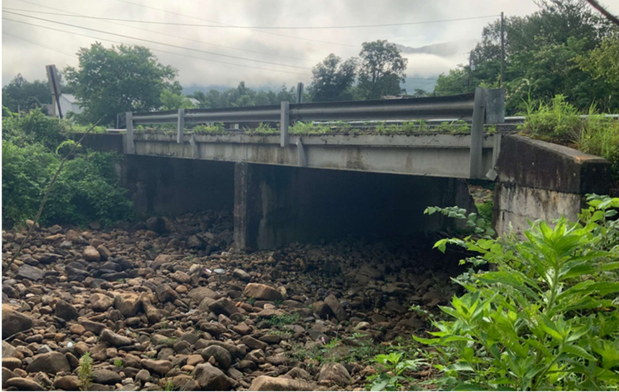
Figure 199 – Bridge 083-0046-0 Side View (GDOT, 2022)
