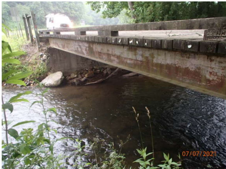
Figure 39: Bridge 291-5028-0 Side View (GDOT, 2021)
