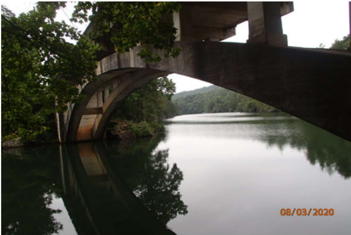
Figure 70: Side View of Bridge 241-5024-0 (GDOT, 2020)
