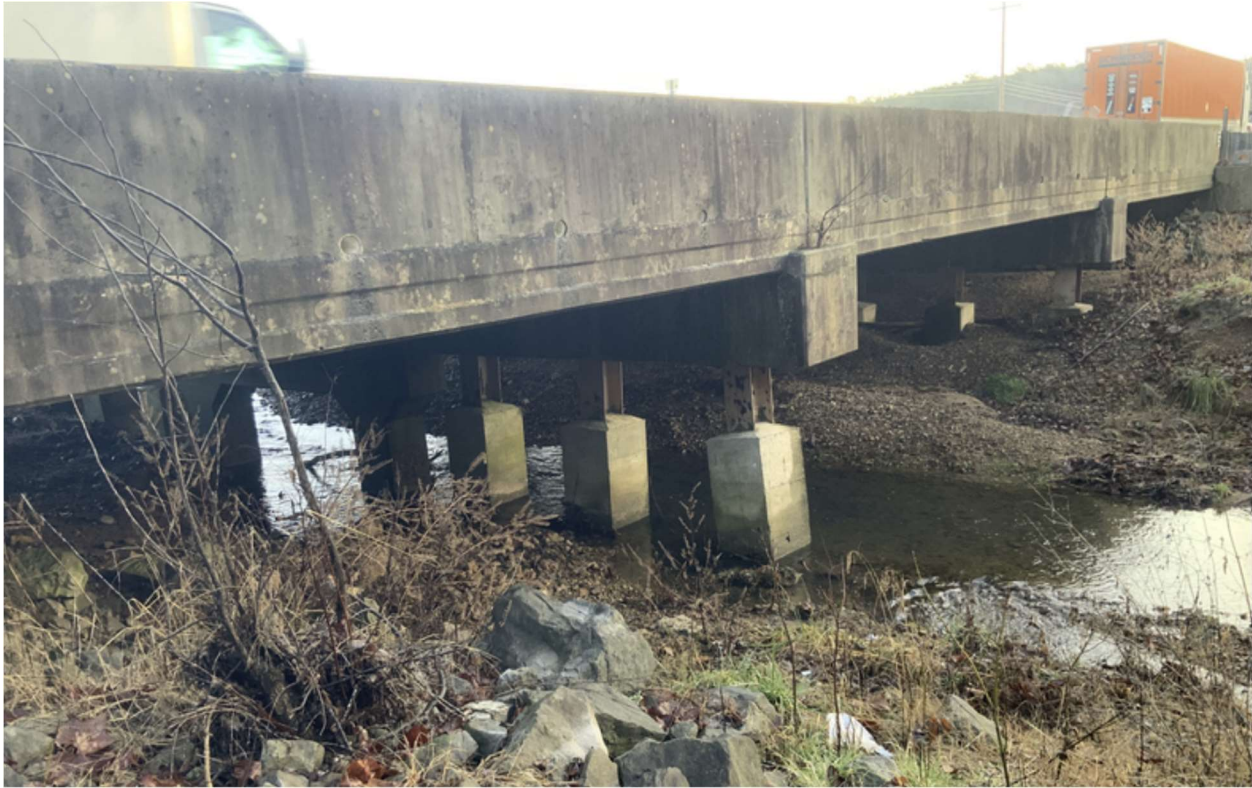
Figure 91 – Bridge 295-0015-0 Side View (GDOT, 2021)
