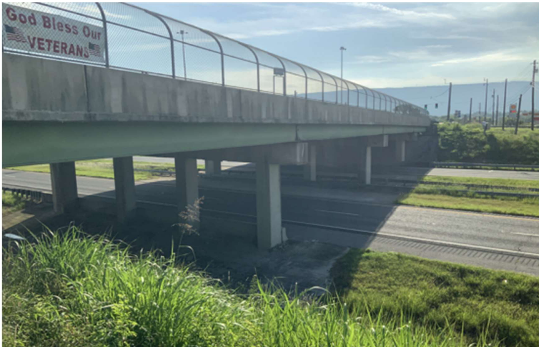
Figure 123 – Bridge 083-0012-0 Side View (GDOT, 2021)
