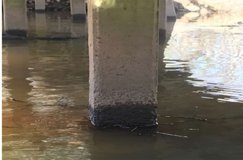
Figure 234 – Bridge 231-5024-0 Typical Reinforced Concrete Pile Condition (GDOT, 2021)
