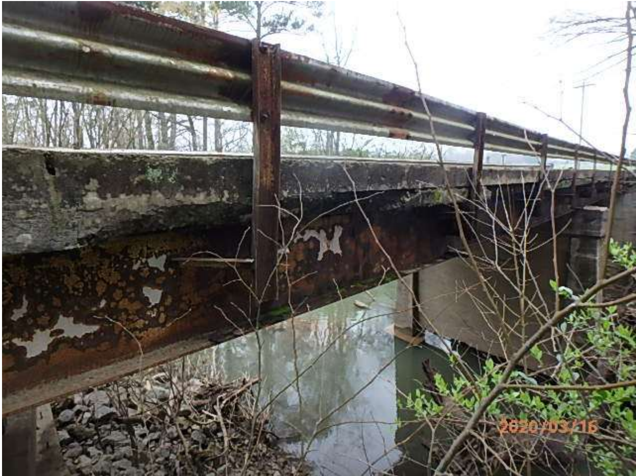
Figure 165 – Bridge 055-5030-0 Steel Girder Condition (GDOT, 2020)
