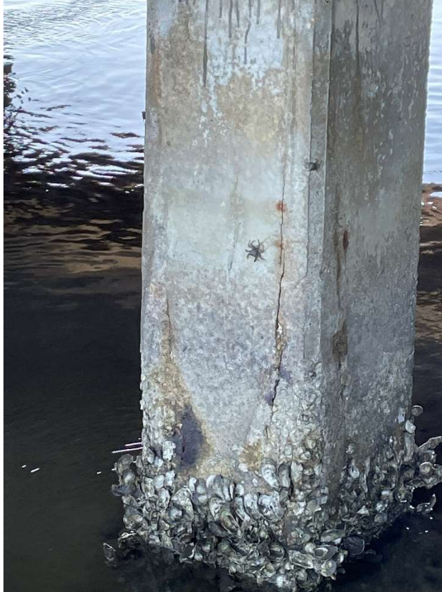
Figure 288 – Bridge 039-0049-0 Prestressed Concrete Piles Typical Condition (GDOT, 2021)
