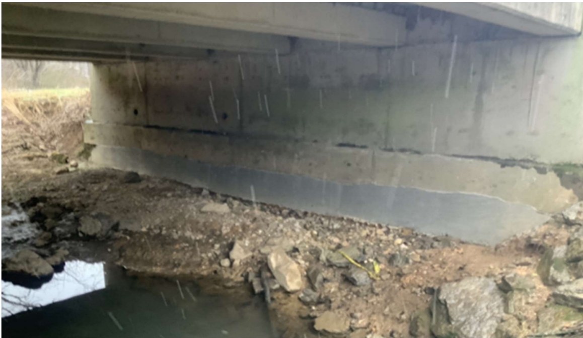
Figure 97 – Bridge 295-0039-0 Reinforced Concrete Abutment 2015 (Top) vs 2021 (Bottom)
