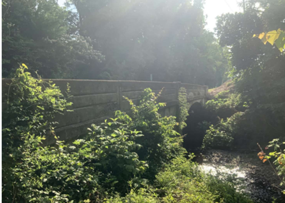
Figure 191 – Bridge 313-5002-0 Side View (GDOT, 2022)
