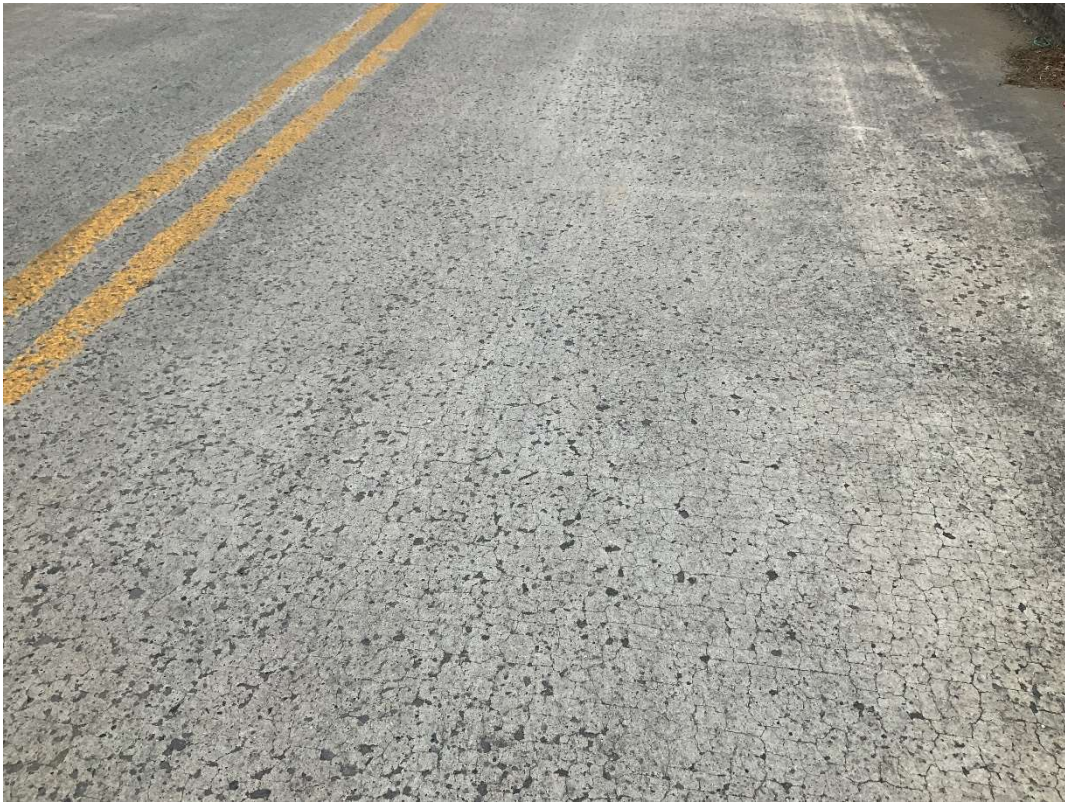
Figure 166 – Bridge 055-5030-0 Deck Topside Condition (GDOT, 2022)
