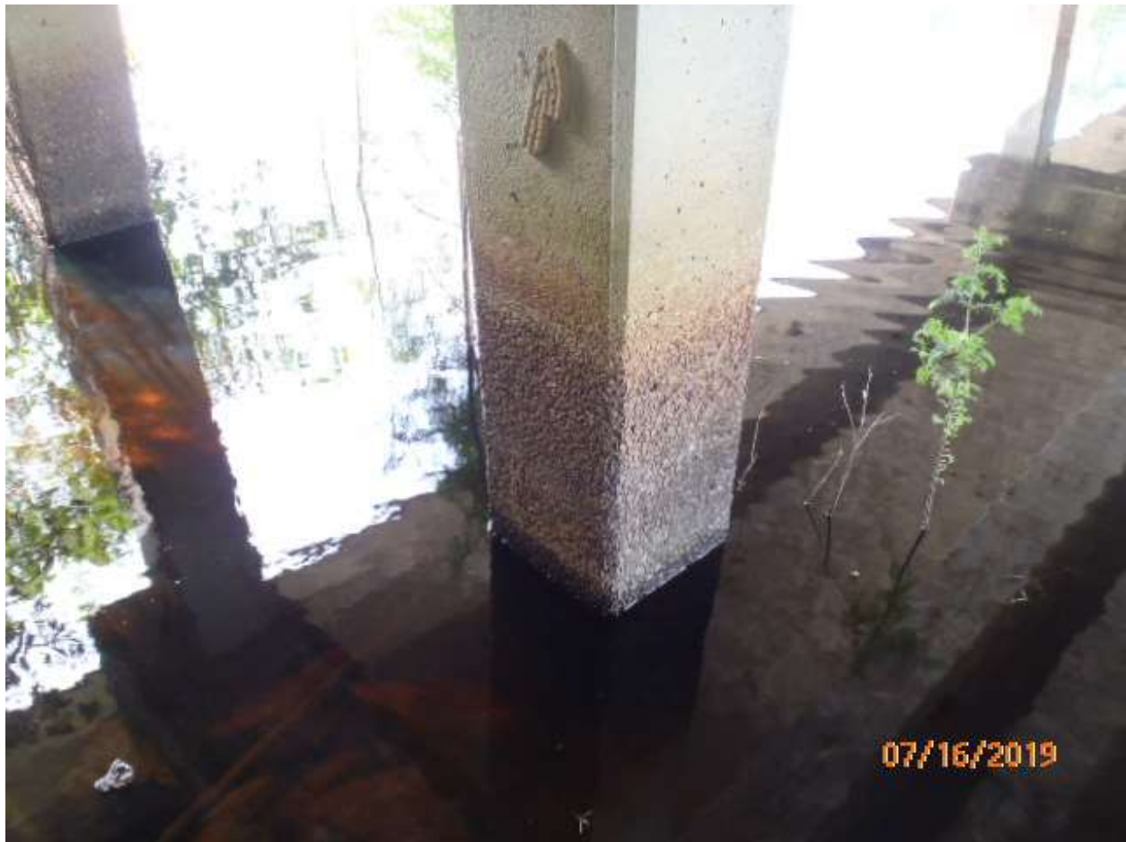
Figure 231 – Bridge 283-5026-0 Typical Pile Condition (GDOT, 2019)
