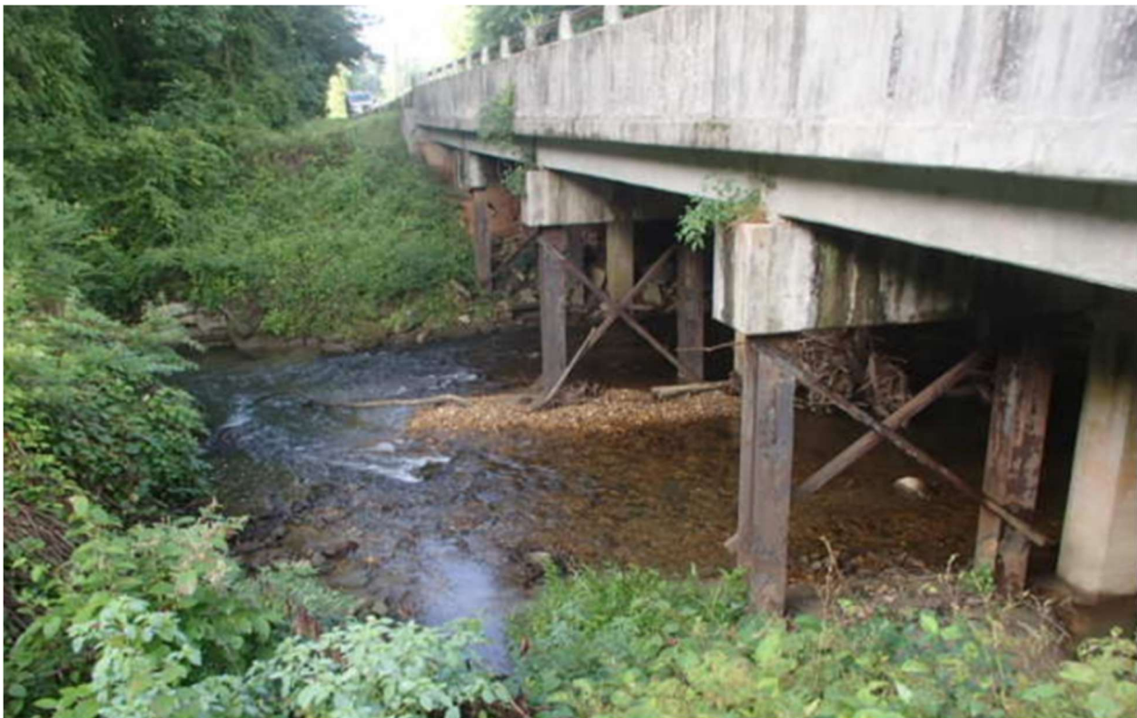
Figure 150 – Bridge 241-0016-0 Side View (GDOT, 2022)
