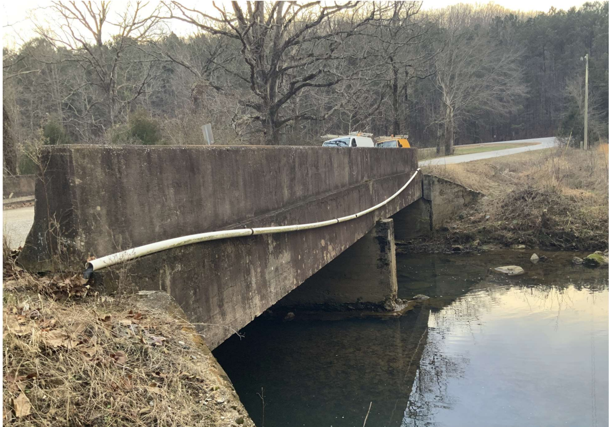
Figure 105 – Bridge 295-5011-0 Side View (GDOT, 2022)
