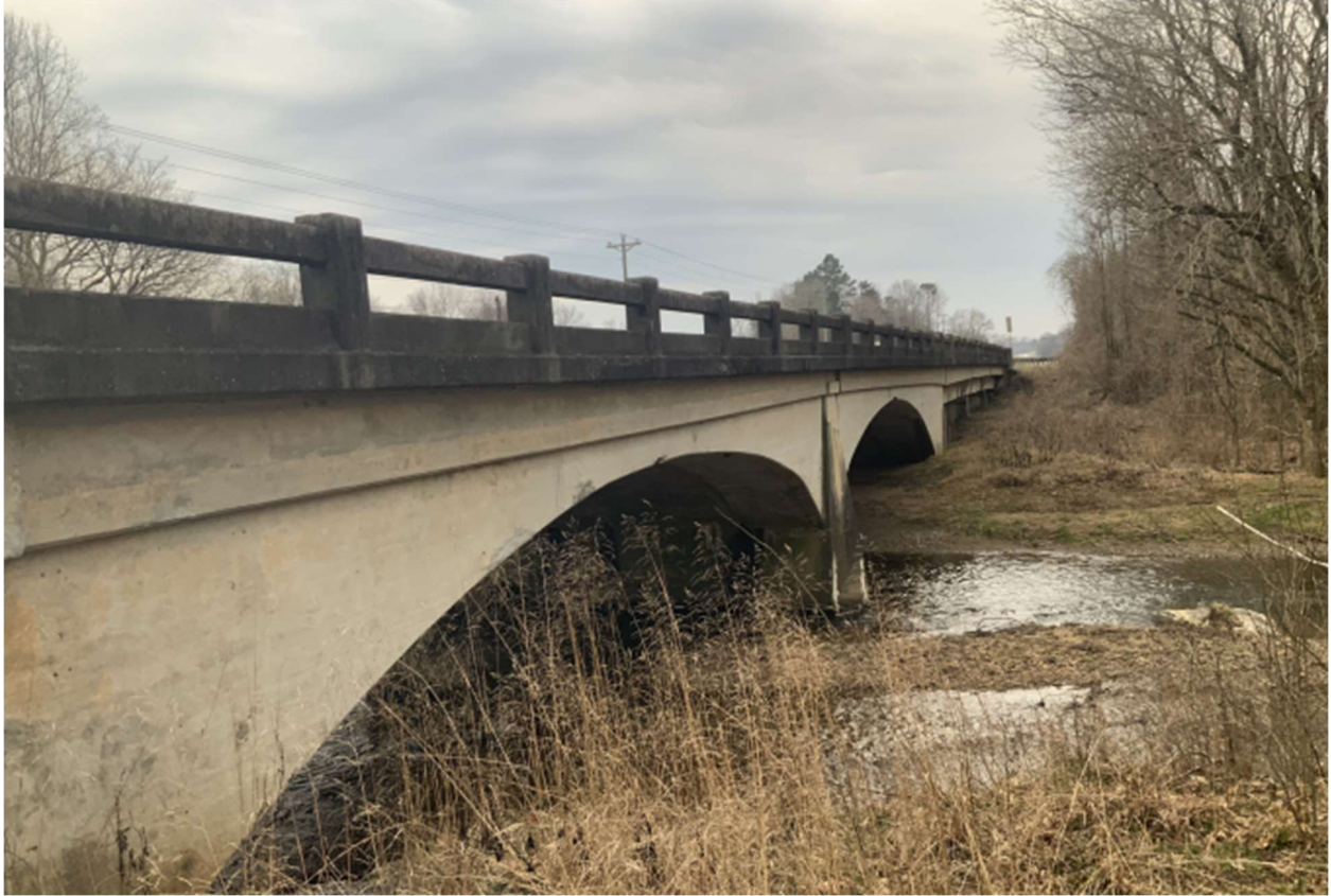
Figure 195 – 213-0017-0 Side View (GDOT, 2022)
