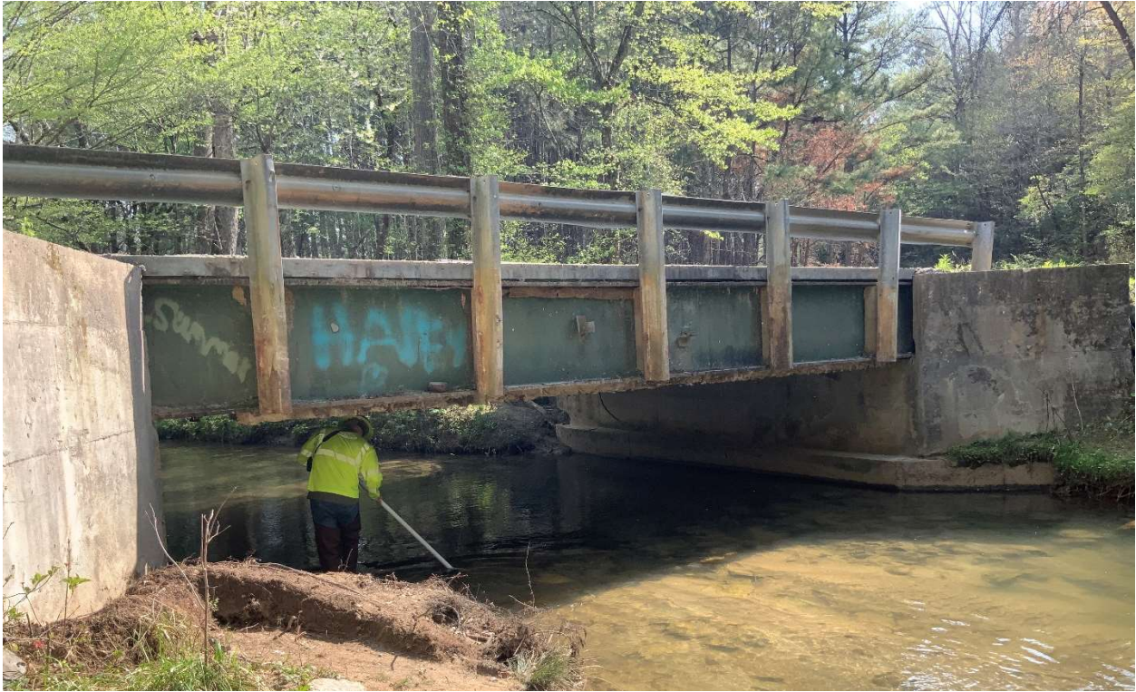
Figure 201 – Bridge 123-5060 Side View (GDOT, 2021)
