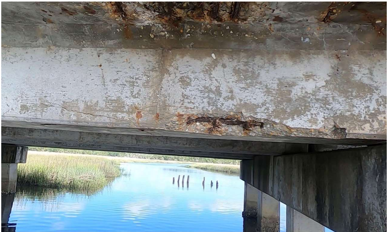
Figure 289 – Bridge 039-0049-0 Reinforced Concrete Girder Condition 2017 (Top) vs 2021 (Bottom)
