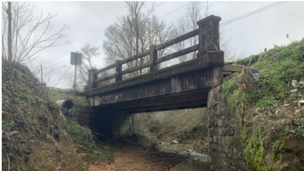
Figure 101 – Bridge 055-5037-0 Side View (GDOT, 2022)
