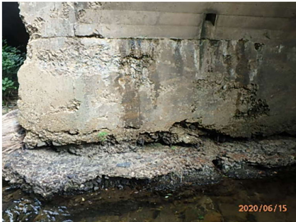
Figure 192 – Bridge 313-5002-0 Reinforced Concrete Pier Wall Condition (GDOT, 2020)
