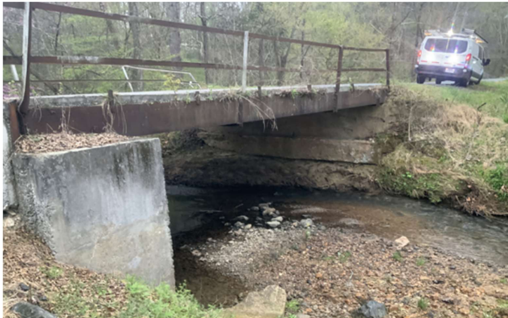
Figure 43: Bridge 055-5009-0 Side View (GDOT, 2022)
