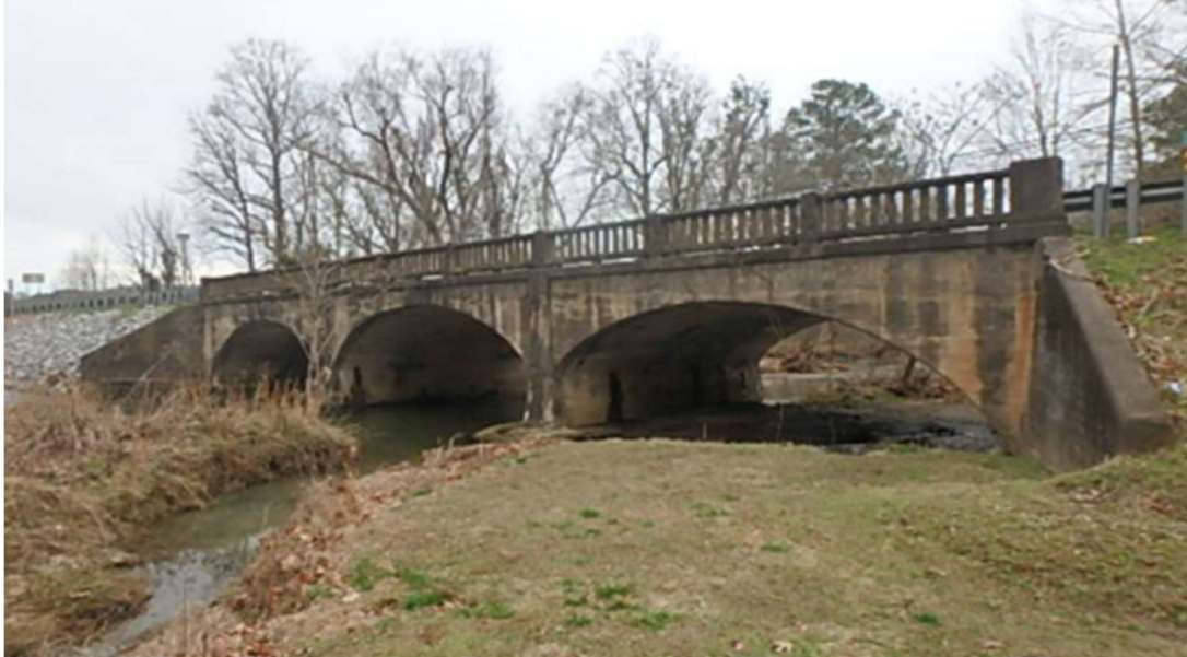
Figure 56: Bridge 213-0033-0 Left Side View (GDOT, 2020)
