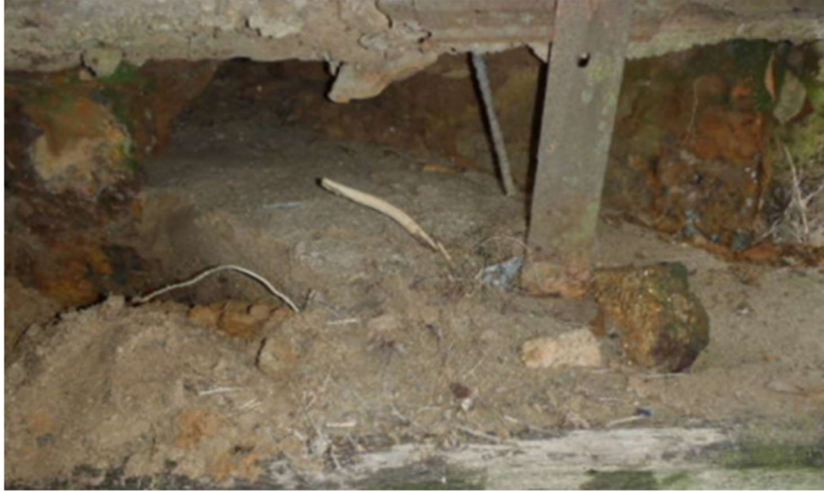
Figure 217 – Bridge 147-5080-0 Typical Abutment Condition (GDOT, 2021)
