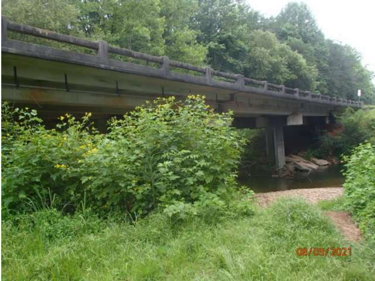
Figure 241 – Bridge 291-0018-0 Side View (GDOT, 2021)
