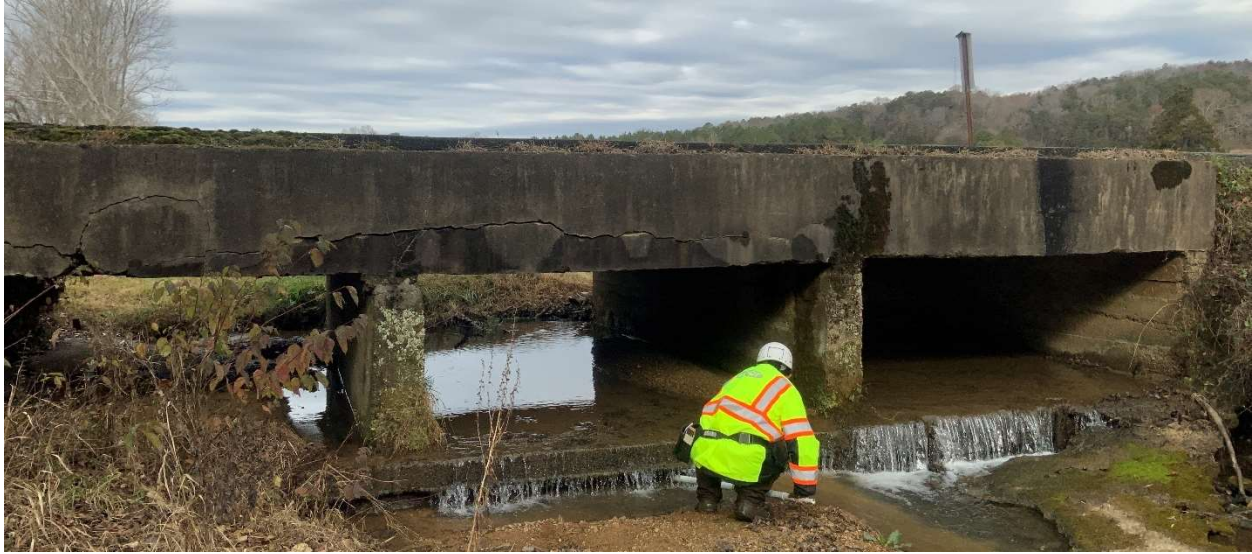
Figure 188 – Bridge 233-5026-0 Side View (GDOT, 2022)
