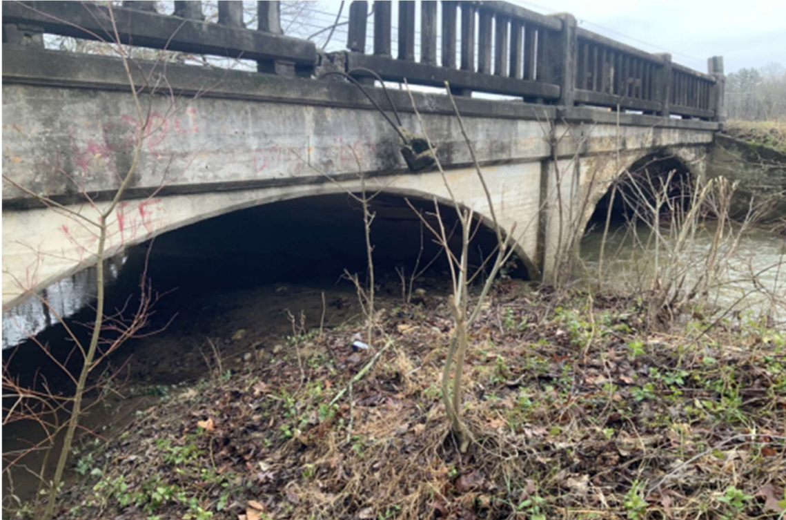
Figure 48: Left Side View of Bridge 213-0045-0 (GDOT, 2022)
