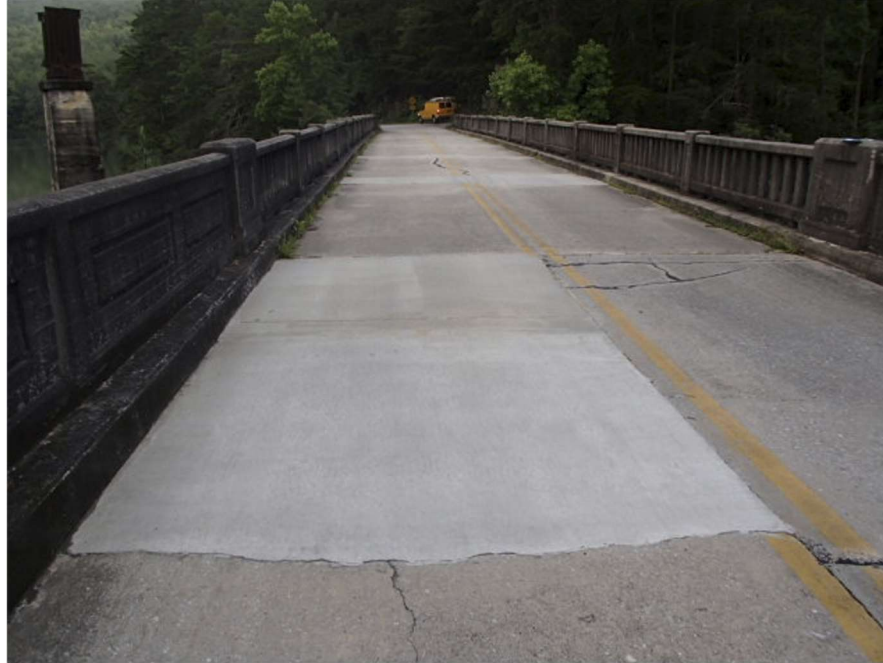
Figure 77: Reinforced Concrete Deck Patching on Bridge 241-5024-0 (GDOT, 2022)
