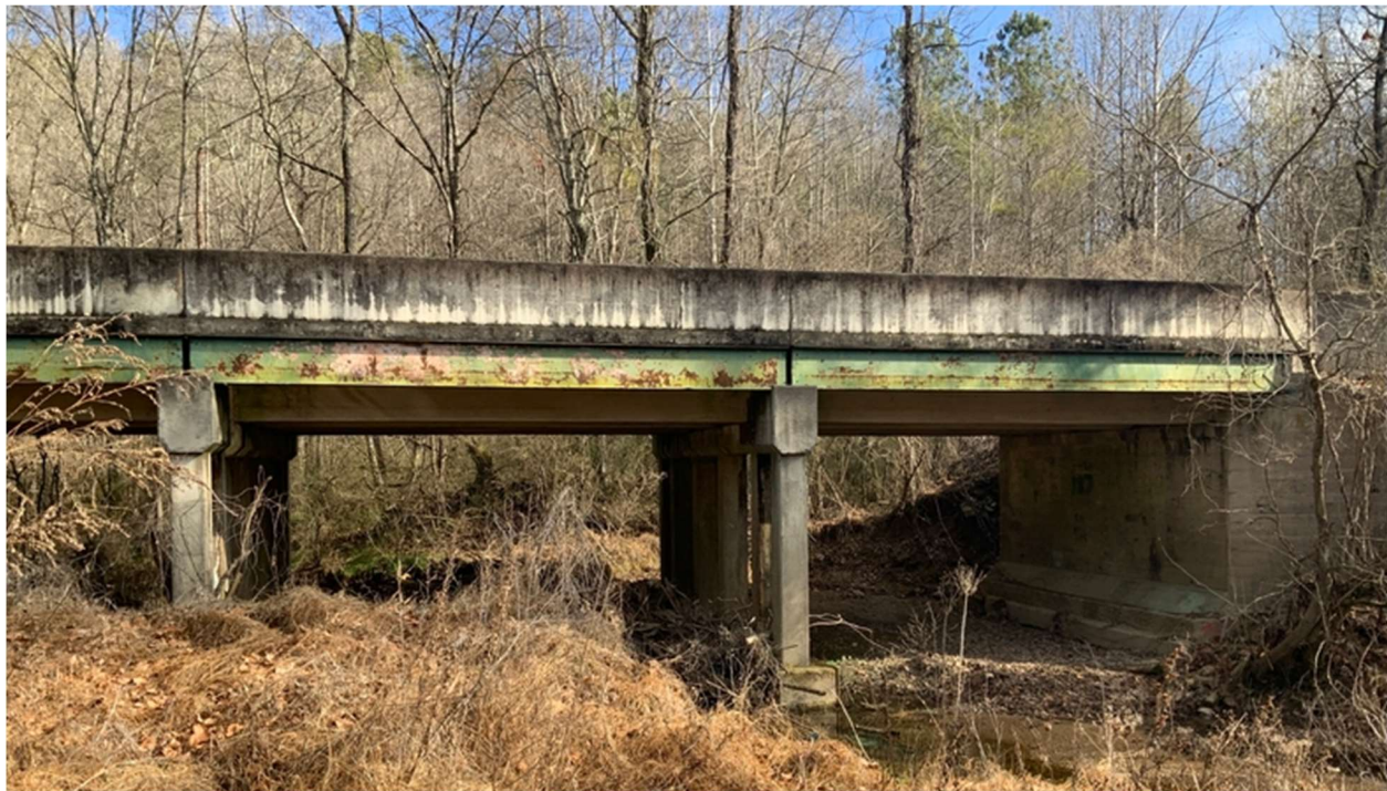
Figure 98 – Bridge 295-0041-0 Side View (GDOT, 2021)
