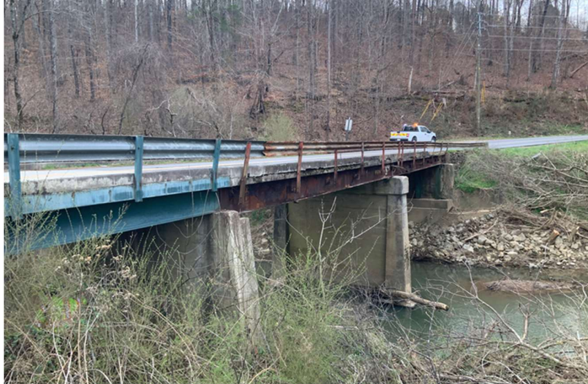
Figure 78 - Bridge 055-5030-0 Side View (GDOT, 2022)
