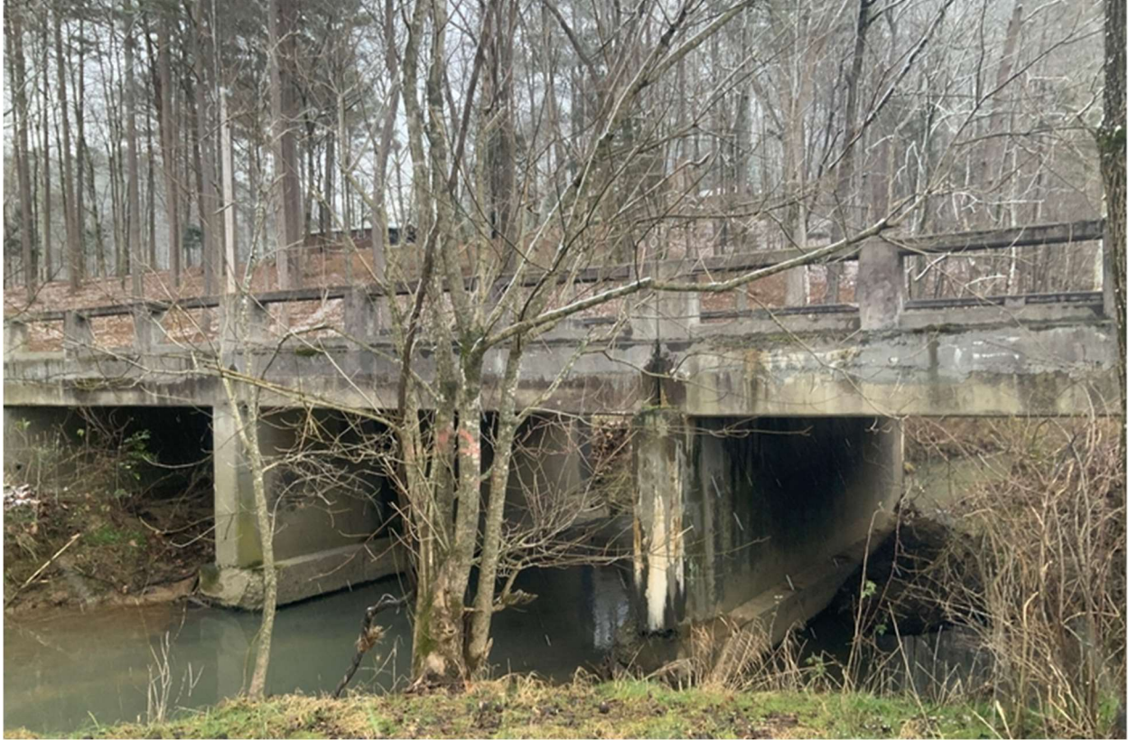
Figure 94 – Bridge 295-0039-0 Side View (GDOT, 2021)
