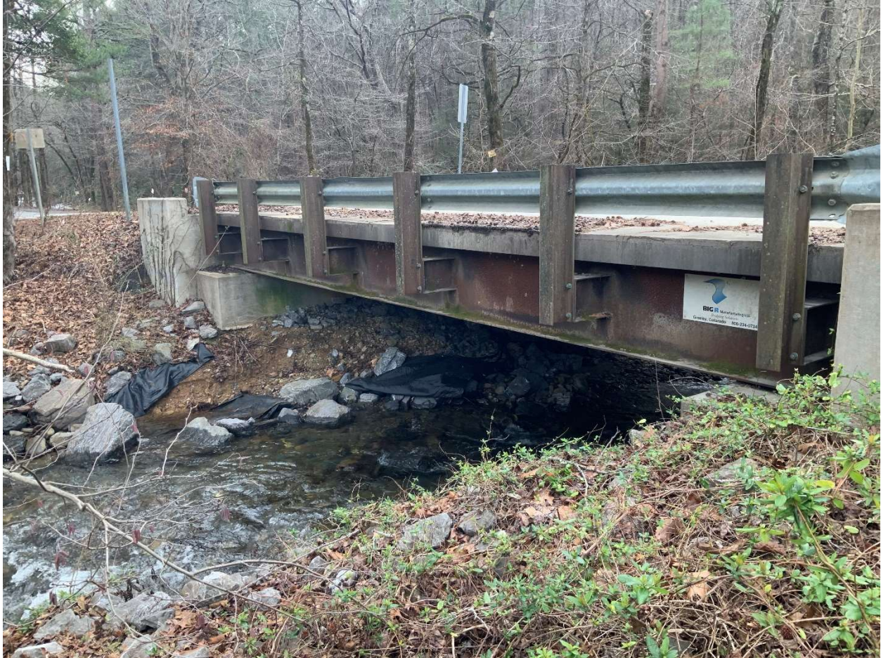
Figure 207 – Bridge 213-5044-0 Bridge Side View (GDOT, 2022)
