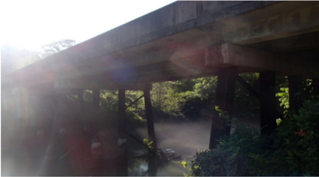
Figure 172 – Bridge 291-5035-0 Side View (GDOT, 2019)
