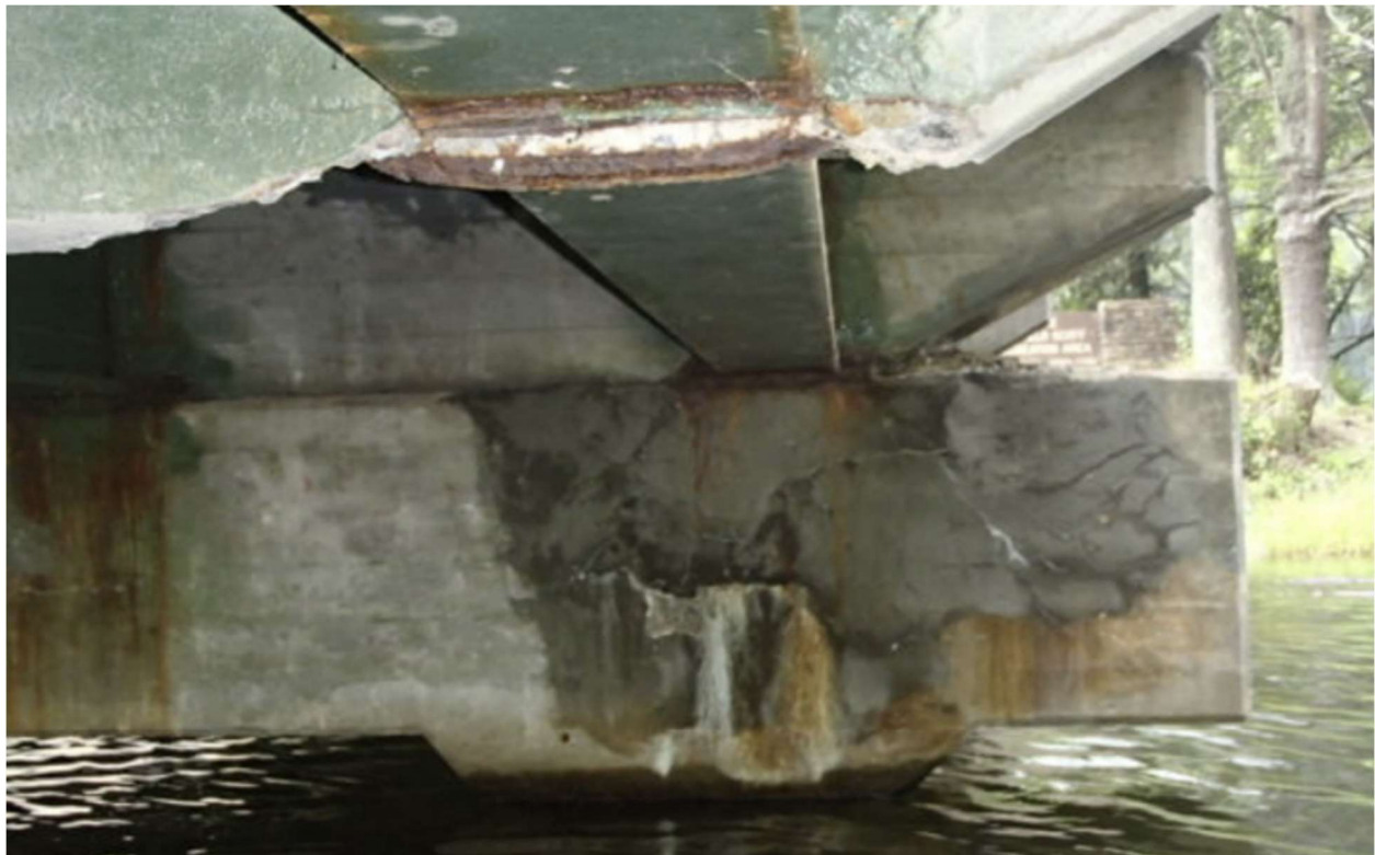
Figure 131 – Bridge 291-0017-0 Reinforced Concrete Pier Cap (GDOT, 2021)
