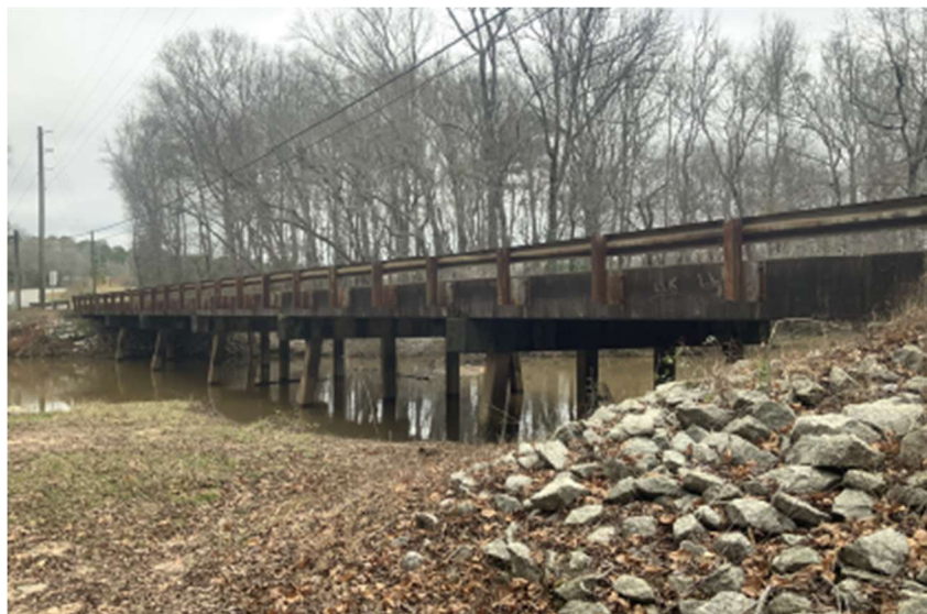
Figure 233 – Bridge 231-5024-0 Side View (GDOT, 2021)
