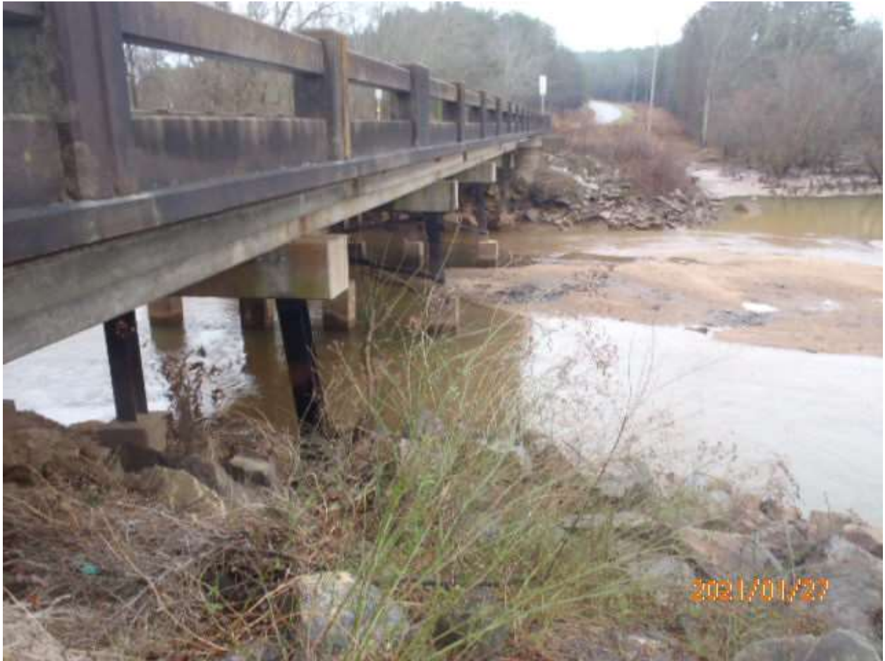
Figure 256 – Bridge 257-0012-0 Side View (GDOT, 2021)
