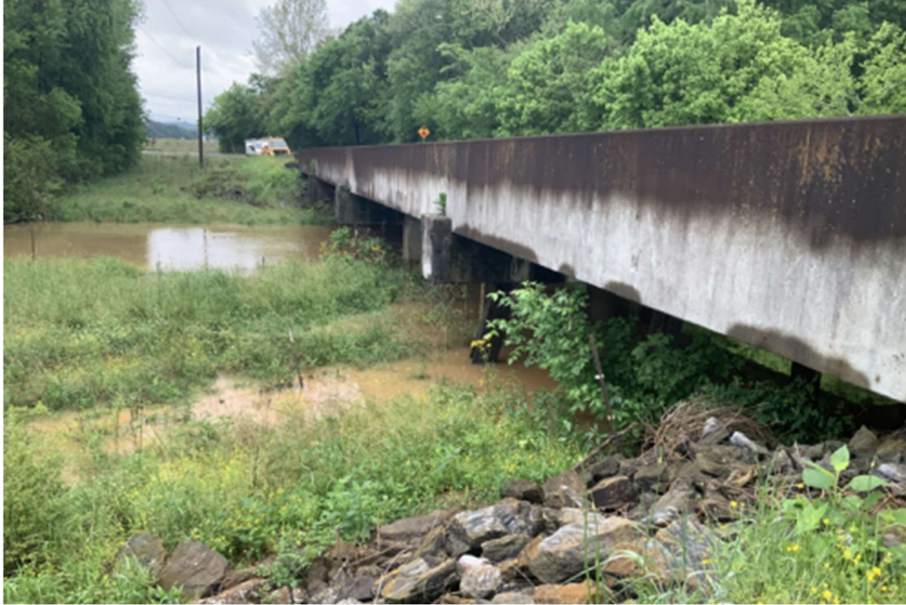
Figure 175 – Bridge 129-5003-0 Side View, 2022
