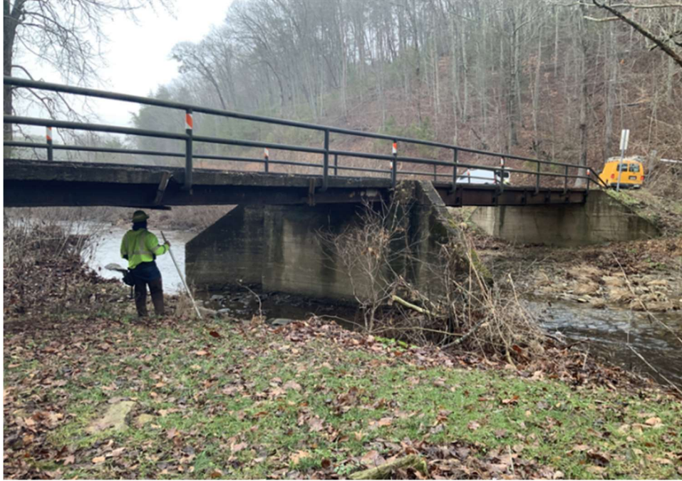
Figure 59 - Bridge 213-5004-0 Side View (GDOT, 2021)
