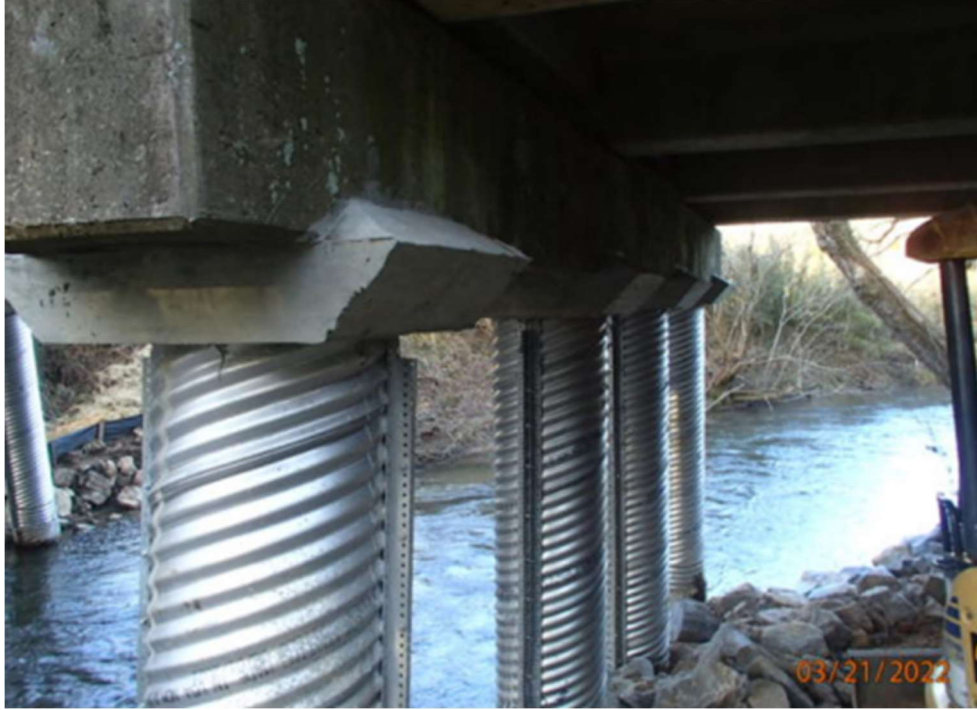
Figure 179 – Bridge 111-5002-0 Steel Pile Repair (GDOT, 2022)
