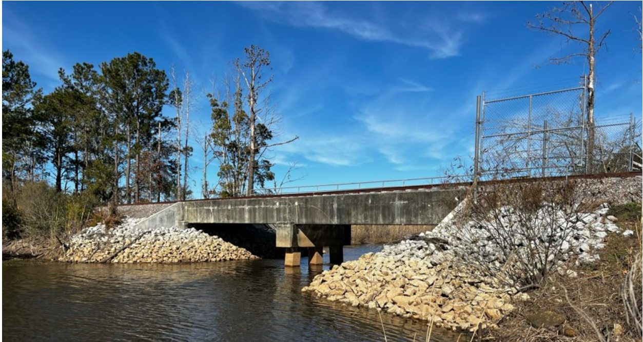
Figure 1.1: Armoring at the base of the railroad crossing at HAAF
