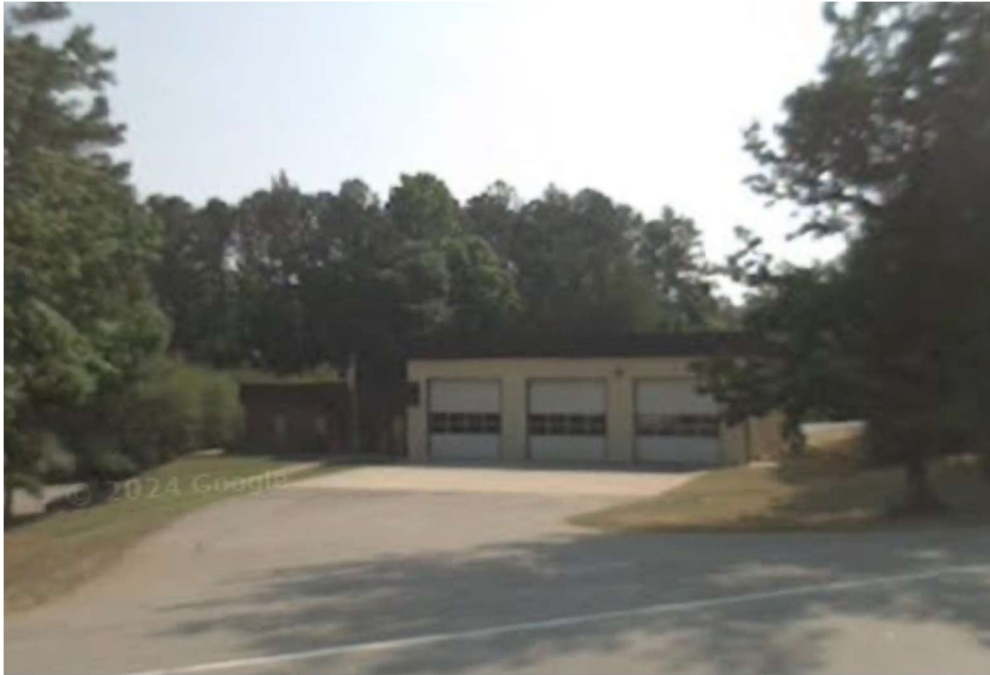
Figure 29- A 2008 Google Street View screenshot of the original appearance of Station No. 6 (Courtesy of Google Street View, image capture date June 2008).
