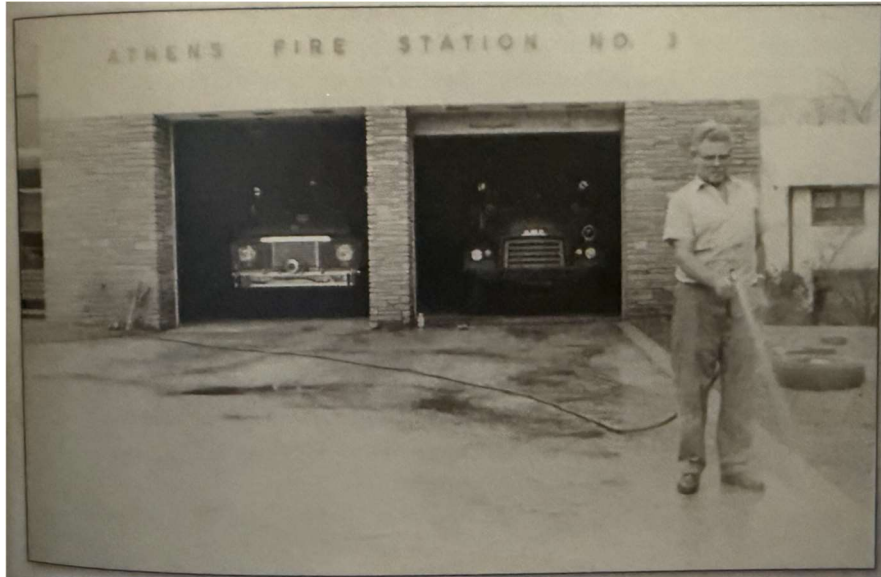
Figure 19- The original facade of Old No. 3 with stone accents (Courtesy of Athens-Clarke County Fire Department).
