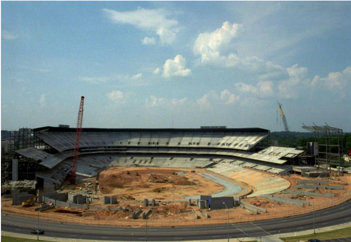
Figure Forty-Three: The Olympic Stadium under construction on June 28, 1995. Courtesy of WBUR and John Bazemore, Associated Press
