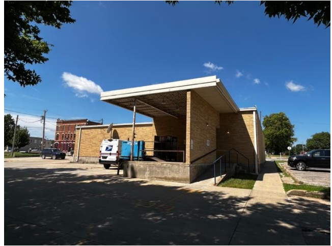
Figure B41: Rear and east elevations of the Garnett Post Office (Haylee Rose, 2025).
