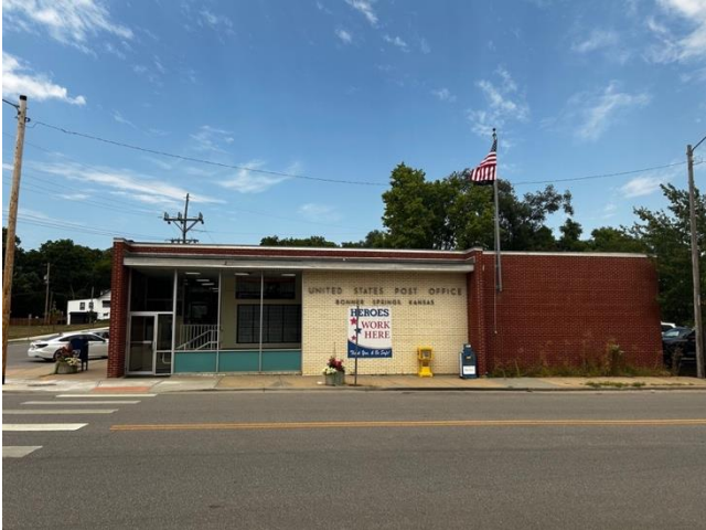
Figure B28: Front elevation of the Bonner Springs Post Office (Haylee Rose, 2024).
