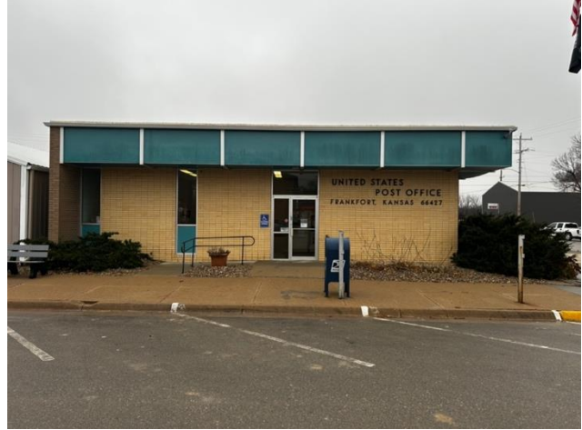
Figure 38: Frankfort Post Office built in 1967 illustrating a Thousand Series main post office with a traditional flat roof (Haylee Rose, 2025).
