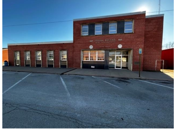
Figure 29: Sedan Post Office and Federal Building, constructed 1958. Character-defining features include asymmetrical massing with one section two stories or higher, a flat roof, granite window detailing, exterior dedication plaque, and federal seals ( Haylee Rose, 2025).
