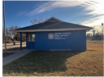
Figure 75: Elk City Post Office, despite having been constructed in 1991, still has many of the character-defining features of Thousand Series main post offices indicating smaller main post offices constructed post 1975 may still be eligible under the Thousand Series umbrella (2025, Haylee Rose).
