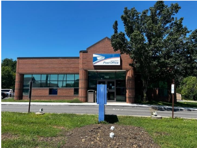
Figure B94: Front elevation of the Overland Park Post Office (Haylee Rose, 2024).
