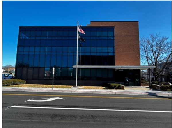
Figure 31: Leavenworth Post Office and Federal Building, constructed 1959. Character-defining features include asymmetrical massing with one section two stories or higher, a flat roof, granite window detailing, exterior dedication plaque, and federal seals (Haylee Rose, 2025).
