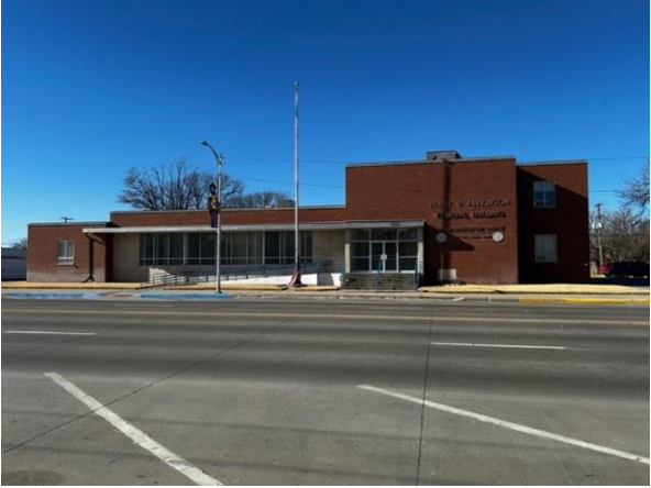
Figure 28: Scott City Post Office and Federal Building, constructed 1965. Character-defining features include asymmetrical massing with one section two stories or higher, a flat roof, picture windows, granite window detailing, and an exterior dedication plaque with federal seals (Haylee Rose, 2025).
