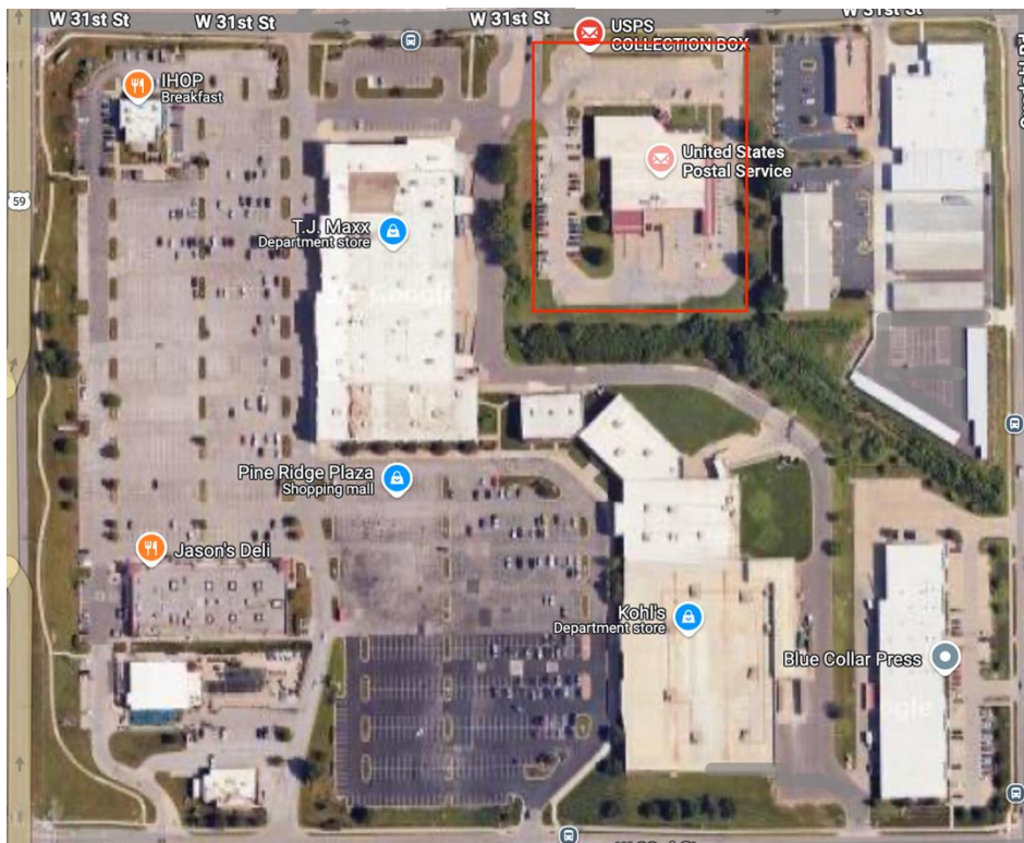
Figure B130: Aerial image of the Lawrence Jayhawk Station Post Office on a central lot of a large commercial block (Google Maps, 2024).
