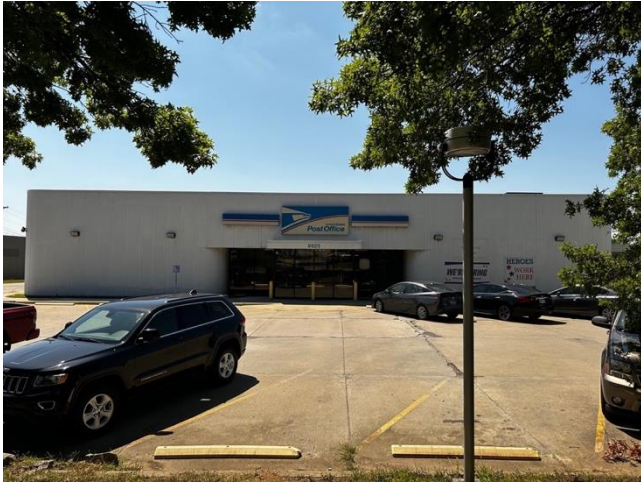
Figure B79: Front elevation of the Lenexa Post Office (Haylee Rose, 2025).
