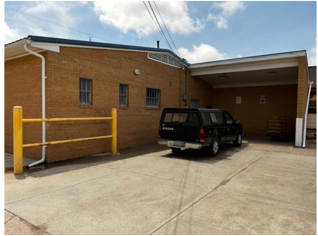
Figure B38: Rear elevation of the Burrton Post Office (Haylee Rose, 2024).
