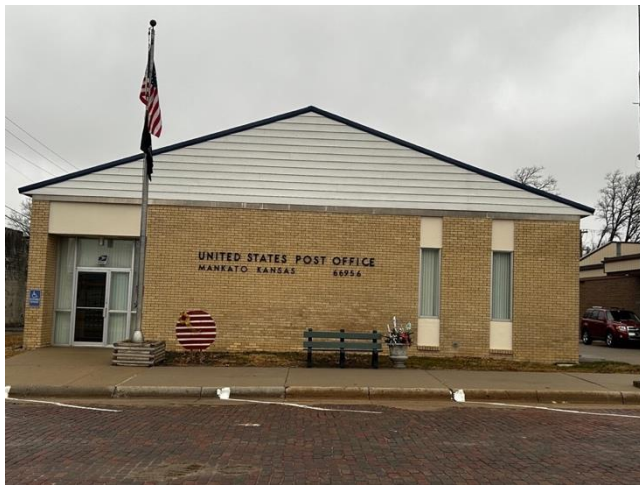
Figure B61: Front elevation of the Mankato Post Office (Haylee Rose, 2025).
