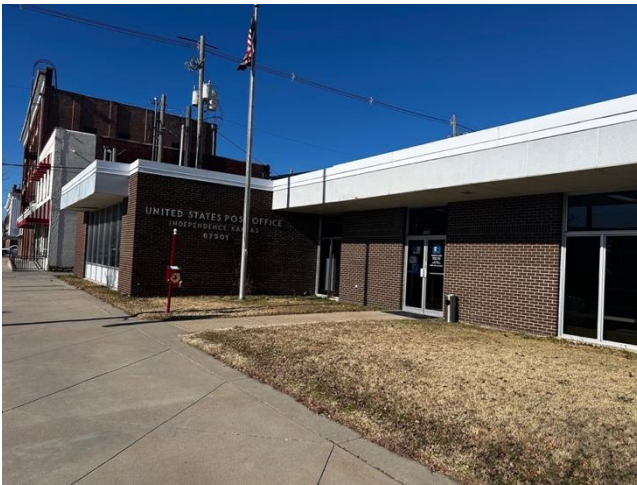
Figure B103: Front elevation of the Independence Post Office looking east (Haylee Rose, 2025).
