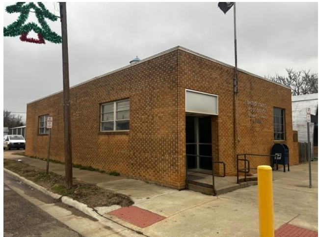
Figure B35: East oblique of the Tescott Post Office (Haylee Rose, 2025).
