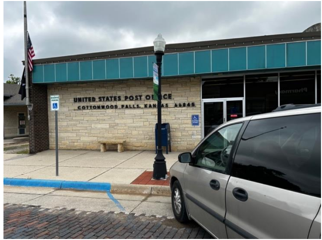
Figure B50: Front elevation of the Cottonwood Falls Post Office (Haylee Rose, 2024).
