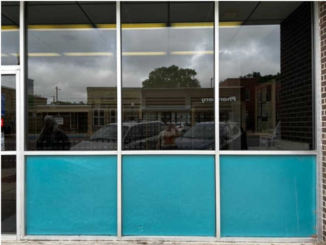
Figure 43: Aqua Window Paneling on the Cottonwood Falls Post Office (Haylee Rose, 2024).
