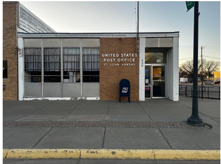
Figure 56: Similarly, to Design 27 the St. John Post Office constructed in 1960 has a bay on vertical tri-part picture windows with silver window paneling with a center section of blond running bond brick veneer separating the windows from the entrance bay (Haylee Rose, 2025).
