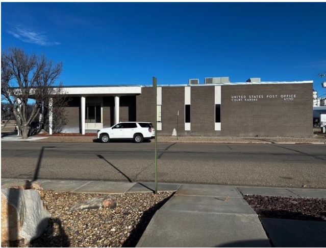
Figure B70: Front elevation of the Colby Post Office (Haylee Rose, 2025).
