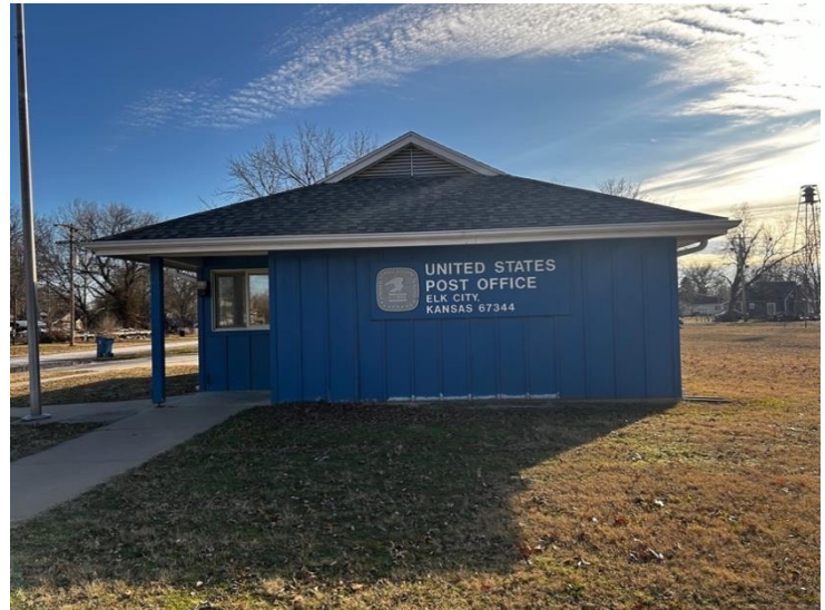
Figure 68: Similarly, to Design 103 the Elk City Post Office constructed in 1991 has the same Polynesian-hipped roof, rectangular massing, and recessed front entrance. (Haylee Rose, 2025).
