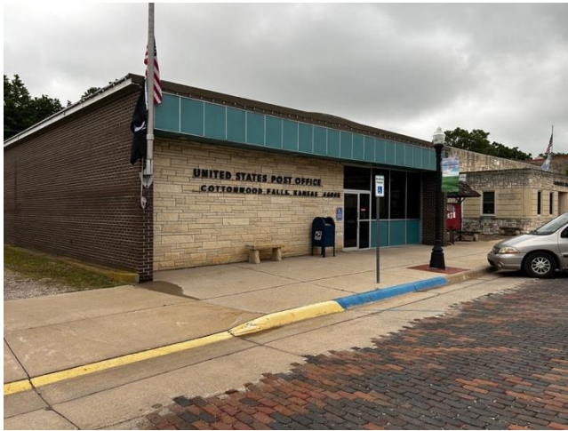
Figure B49: East oblique of the Cottonwood Falls Post Office (Haylee Rose, 2024).
