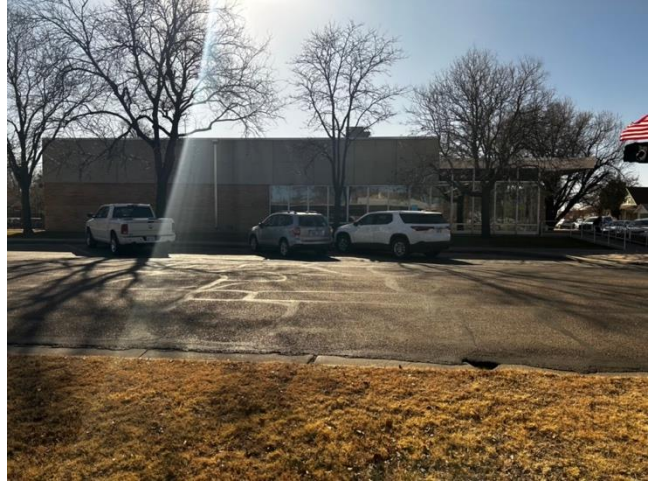
Figure B105: Front elevation of the Garden City Post Office (Haylee Rose, 2025).
