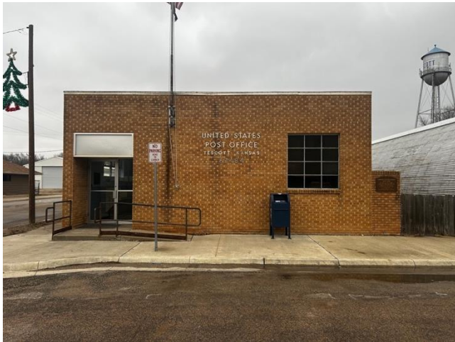
Figure B34: Front elevation of the Tescott Post Office (Haylee Rose, 2025).
