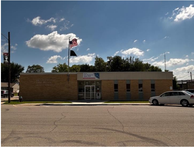
Figure B40: Front elevation of the Garnett Post Office (Haylee Rose, 2025).
