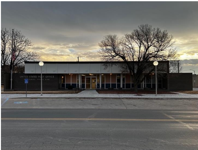
Figure B73: Front elevation of the Phillipsburg Post Office (Haylee Rose, 2025).
