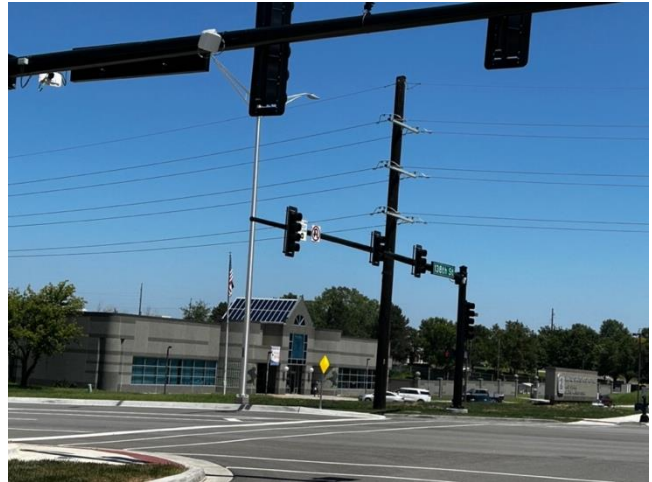
Figure B126: East Oblique of the Olathe East Station Post office (Haylee Rose, 2024).
