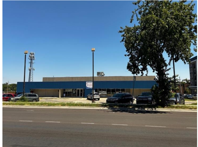
Figure B115: Front elevation of the Olathe Post Office (Haylee Rose, 2024).
