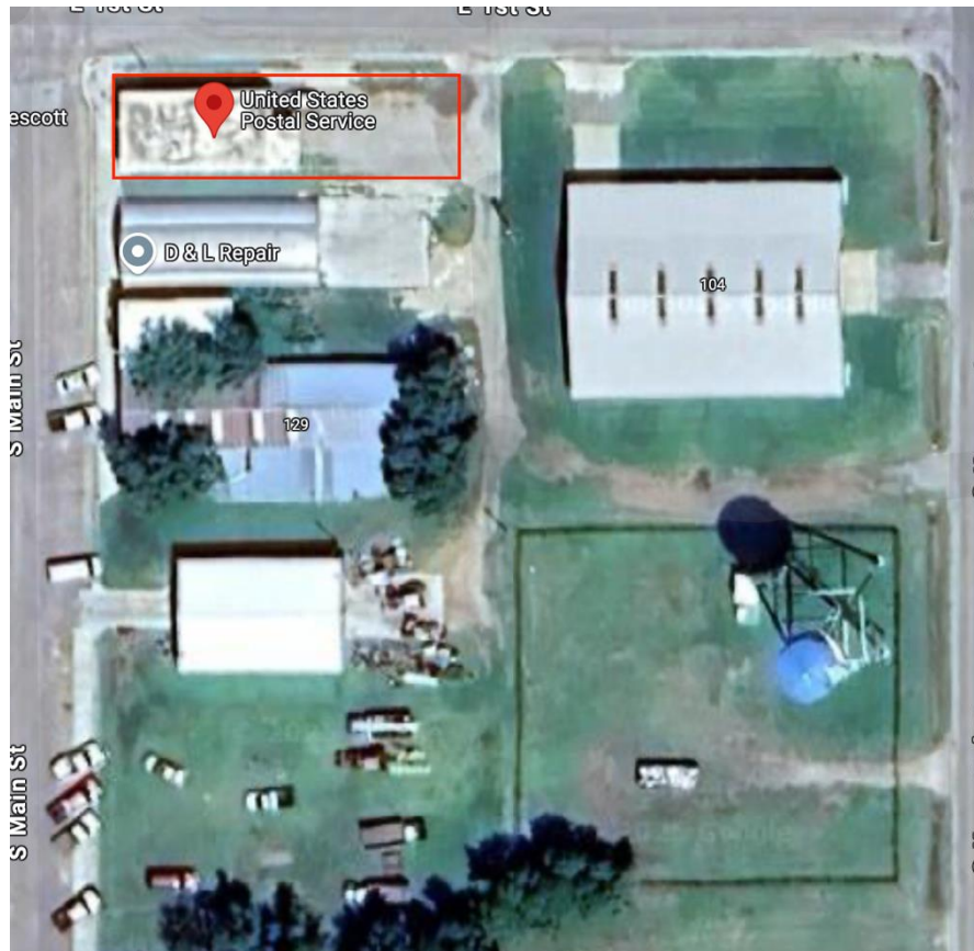
Figure B36: Aerial image of the Tescott Post Office located on the corner lot surrounded by contemporary commercial architecture like metal Quonset huts and prefabricated metal buildings (Google Maps, 2024).
