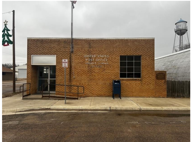
Figure 62: Similarly, to Design 32 the Tescott Post Office constructed in 1961 has a blond running bond brick veneer windows with an attached flagpole and entrance on the far east side of the front elevation. Unlike Design 32 the Tescott post office has only one large 3x4 window and the flagpole is attached in a different location (Haylee Rose, 2025).
