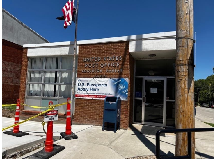
Figure 54: Edgerton Post Office constructed in 1961. Similarly, to the preliminary design the Edgerton facility has a strong horizontal axis with brick veneer and front door on the far western portion of the front elevation. The windows are the same fixed picture windows, but the Edgerton windows are 3x4 as compared to the preliminary design which is 4x4 (Haylee Rose, 2024).
