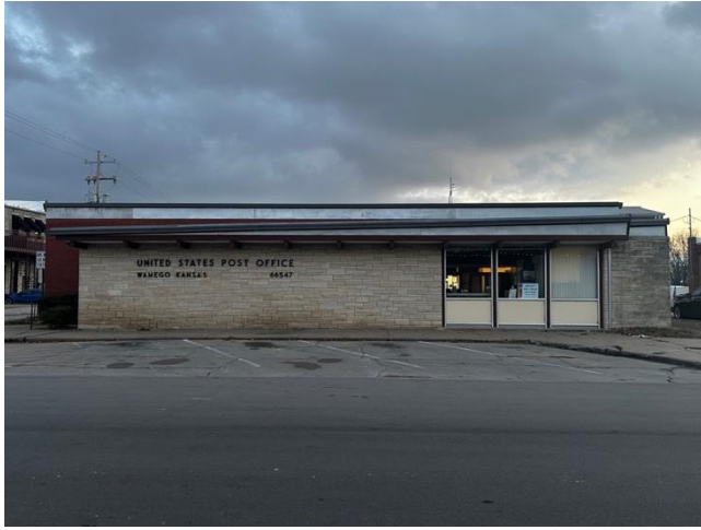
Figure B67: Front elevation of the Wamego Post Office (Haylee Rose, 2025).
