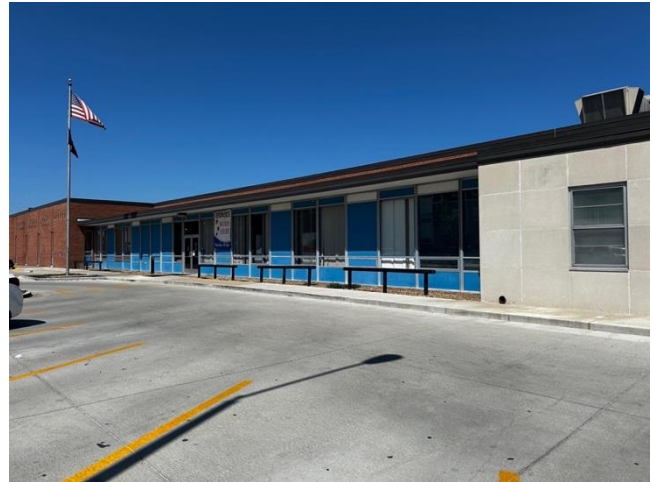
Figure B101: Front elevation of the Shawnee Post Office looking east (Haylee Rose, 2024).
