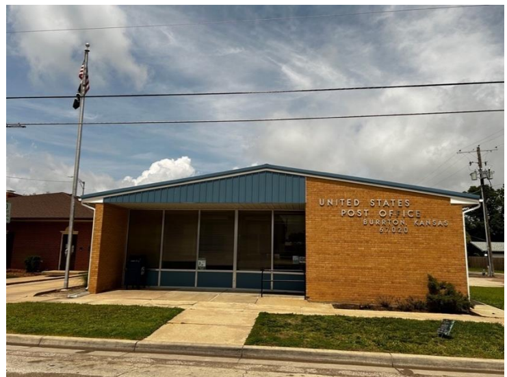
Figure 64: Similarly, to Design 53 the Burrton Post Office is a front gabled main post office constructed in 1961 and has a blond running bond brick veneer with vertical picture windows in the recessed entrance (Haylee Rose, 2024).
