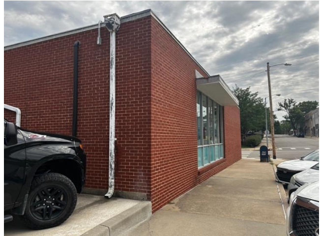
Figure B29: East and Rear of the Bonner Springs Post Office, this is one of the only examples of a main post office with windows on a side elevation (Haylee Rose, 2024).
