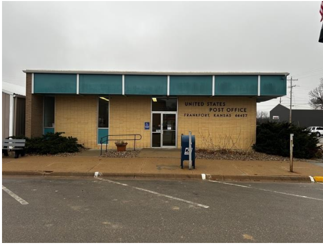
Figure B58: Front elevation of the Frankfort Post Office (Haylee Rose, 2025).
