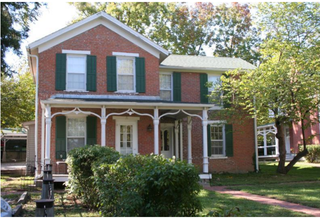
Figure 14: 1505 Kentucky St, Lawrence, Kansas. Greek Revival constructed in 1864. The house is considered a building as it houses human activity (KHRI, 2008).
