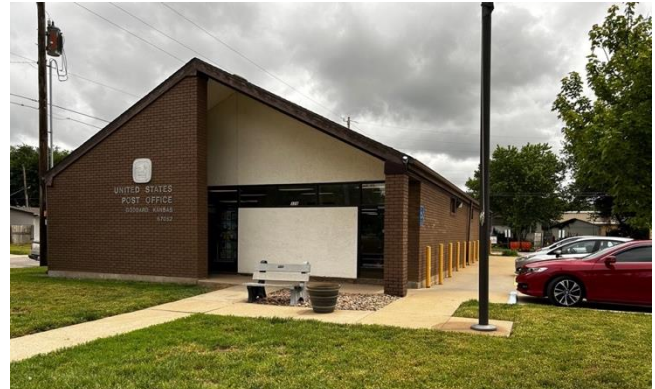
Figure 66: The Goddard Post Office constructed in 1985 is nearly identical to Residential design 24. The post office is constructed out of dark brown running bond brick veneer with stuccoed paneling under the recessed portion of the front gabled roofline. (Haylee Rose, 2024).
