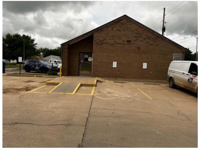
Figure B86: Rear elevation of the Goddard Post Office (Haylee Rose, 2025).
