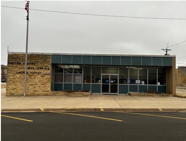
Figure B43: Front elevation of the Lincoln Post Office (Haylee Rose, 2025).
