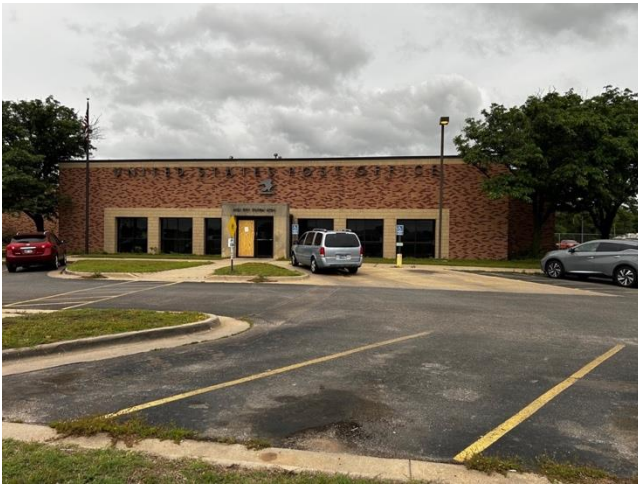
Figure B122: Front elevation of the Wichita River City Station (Haylee Rose, 2024).
