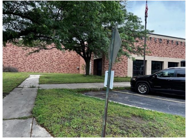
Figure B123: East oblique of the Wichita River City Station (Haylee Rose, 2024).
