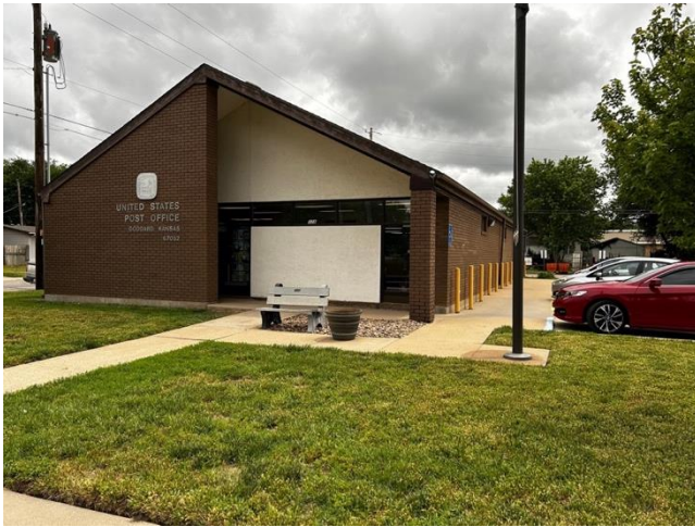
Figure B85: Front elevation of the Goddard Post Office (Haylee Rose, 2025).
