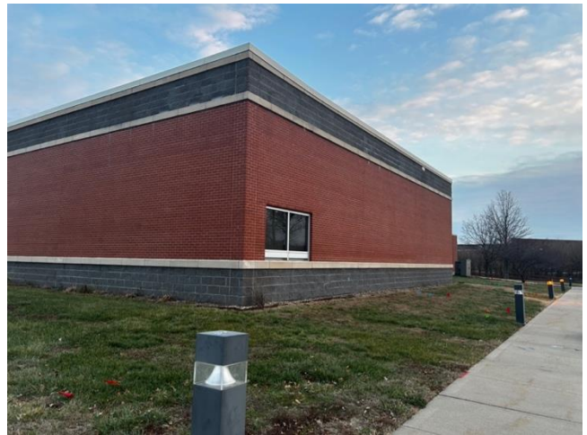
Figure B129: Front and east elevation of the Lawrence Jayhawk Station Post Office (Haylee Rose, 2024).
