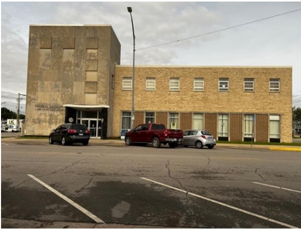
Figure 30: Emporia Post Office and Federal Building, constructed 1959. Character-defining features include asymmetrical massing with one section two stories or higher, a flat roof, a combination of brick patterns and colors with geometric concrete detailing, granite door detailing, exterior dedication plaque, and federal seals (Haylee Rose, 2025).
