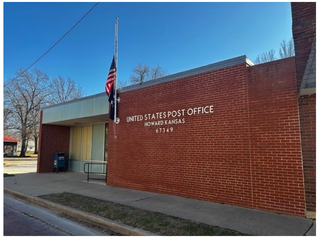
Figure B27: East and rear elevation of the Howard Post Office (Haylee Rose, 2025).
