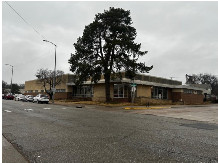
Figure 70: Similarly, to Design 123 the Manhattan Post Office constructed in 1965 has a blond running bond brick veneer with limestone accents and vertical picture windows (Haylee Rose, 2025).
