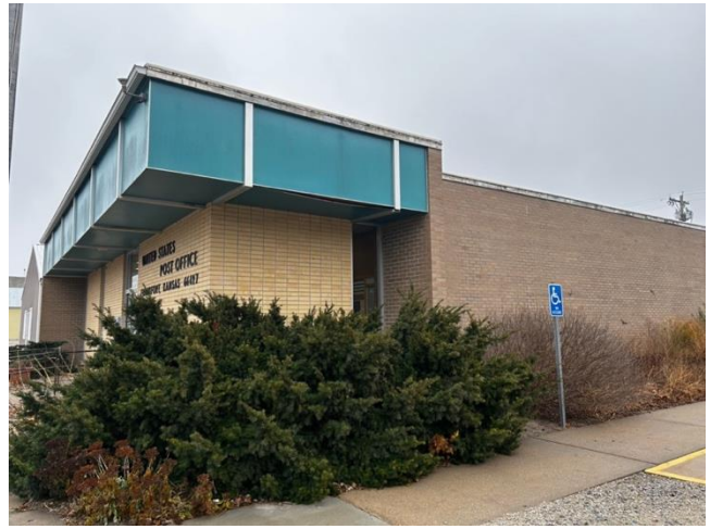
Figure B59: West oblique of the Frankfort Post Office showing the different use of brick colors and pattern on the front and side elevations (Haylee Rose, 2025).
