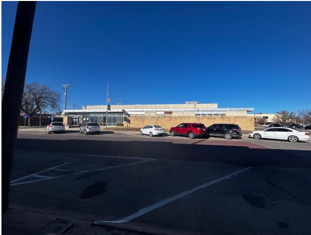
Figure B40: Front elevation of the Liberal Post Office (Haylee Rose, 2025).
