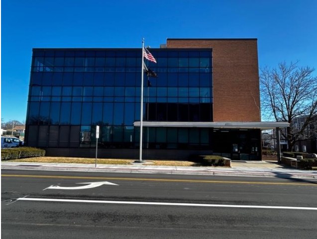
Figure B7: Front elevation of the Leavenworth Post Office and Federal Building (Haylee Rose, 2025).
