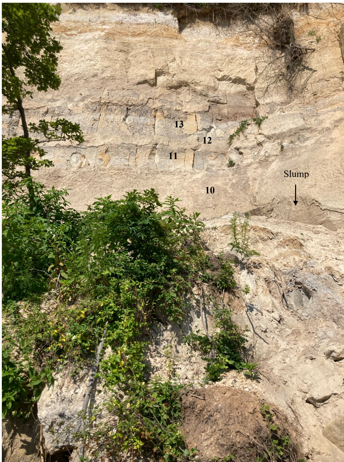
FIGURE 2.2. Slumped section of Shattuck (1904) Bed 10 located below the vertical cracking of Bed 11 (38.67356°N, 76.53076°W).
