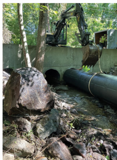
Figure 7, 8. Culvert after trenchless repairs [10].
