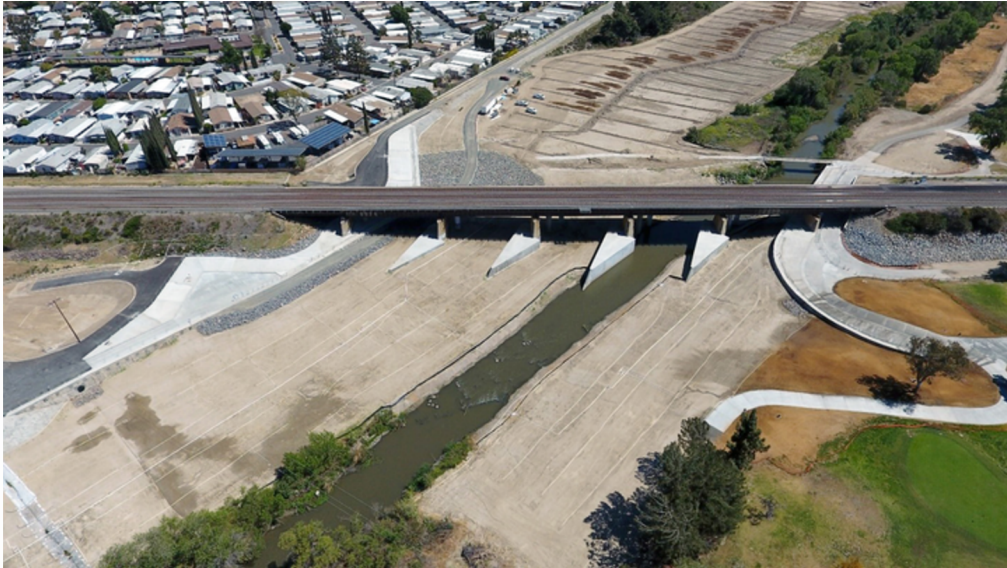
Figure 13. Scour Prevention Measures in Southern California [15].
