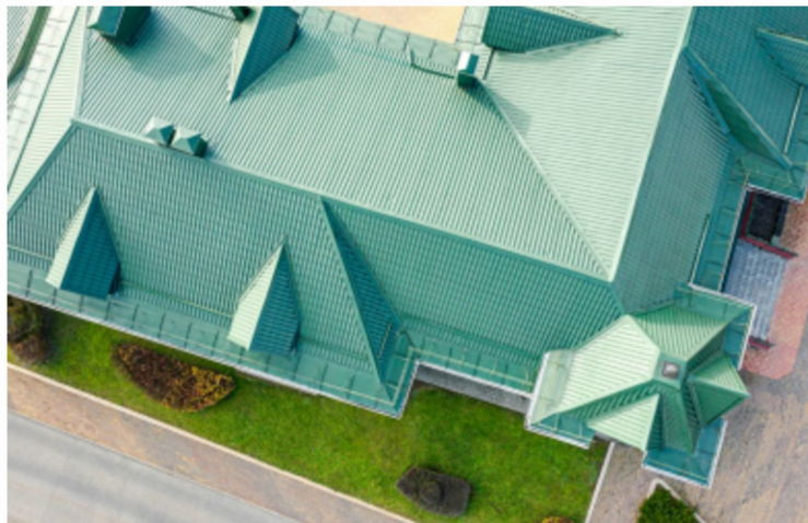
Figure 17. Metal or tile can protect roofs from ignition [20].
