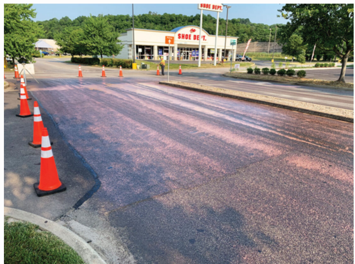
Figure 11. Asphalt rejuvenation [13].
