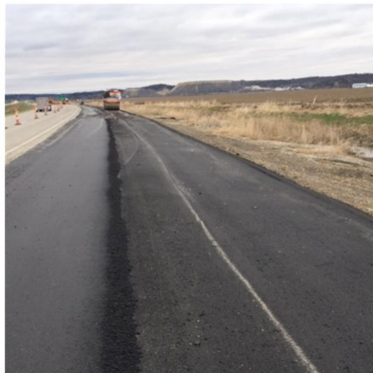
Figure 3.5. Additional Shoulder to Bear Most of the Damage and to Leave the True Shoulder Unaffected, from Bowers & Gu (2021).
