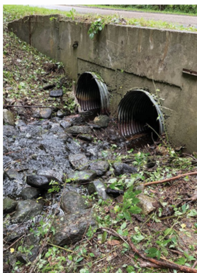
Figure 5, 6. Culvert before trenchless repairs [10].
