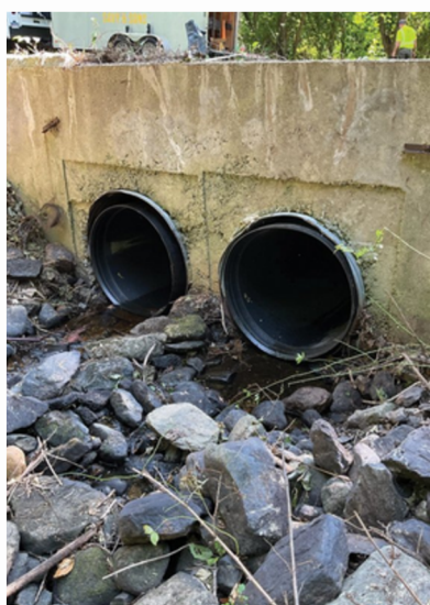
Figure 7, 8. Culvert after trenchless repairs [10].
