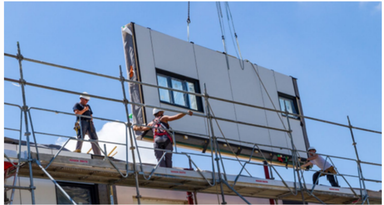
Figure 16. Prefabricated, insulated panels regulate heat and speed up the retrofit process [19].
