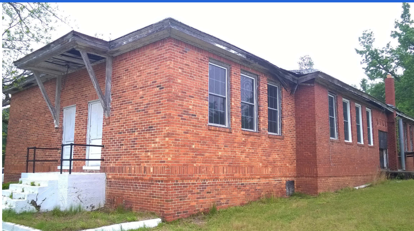
Roof damage is allowing water to penetrate the interior and deteriorate the soffits.
