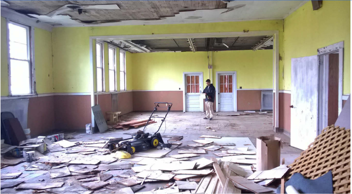
Existing condition of the Dining Hall. Roof is damaged and interior is filled with rubble.
