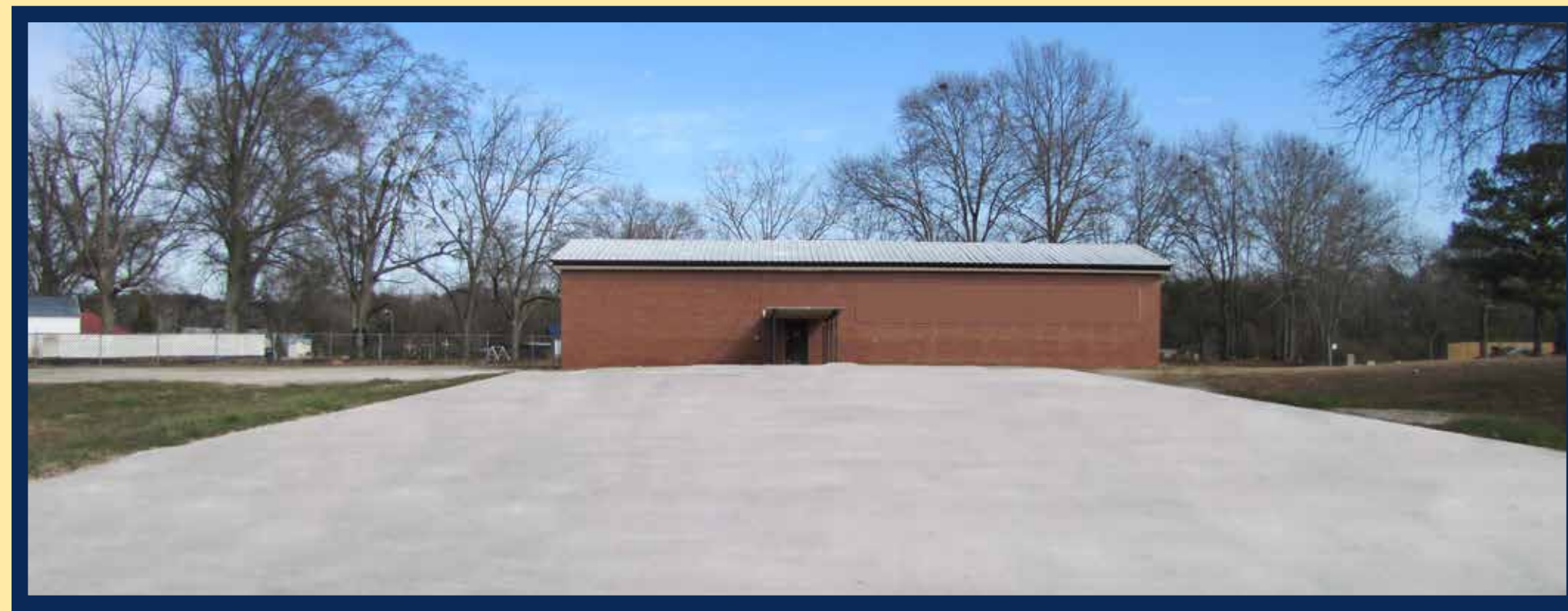
Skim-coat concrete and paint plywood
