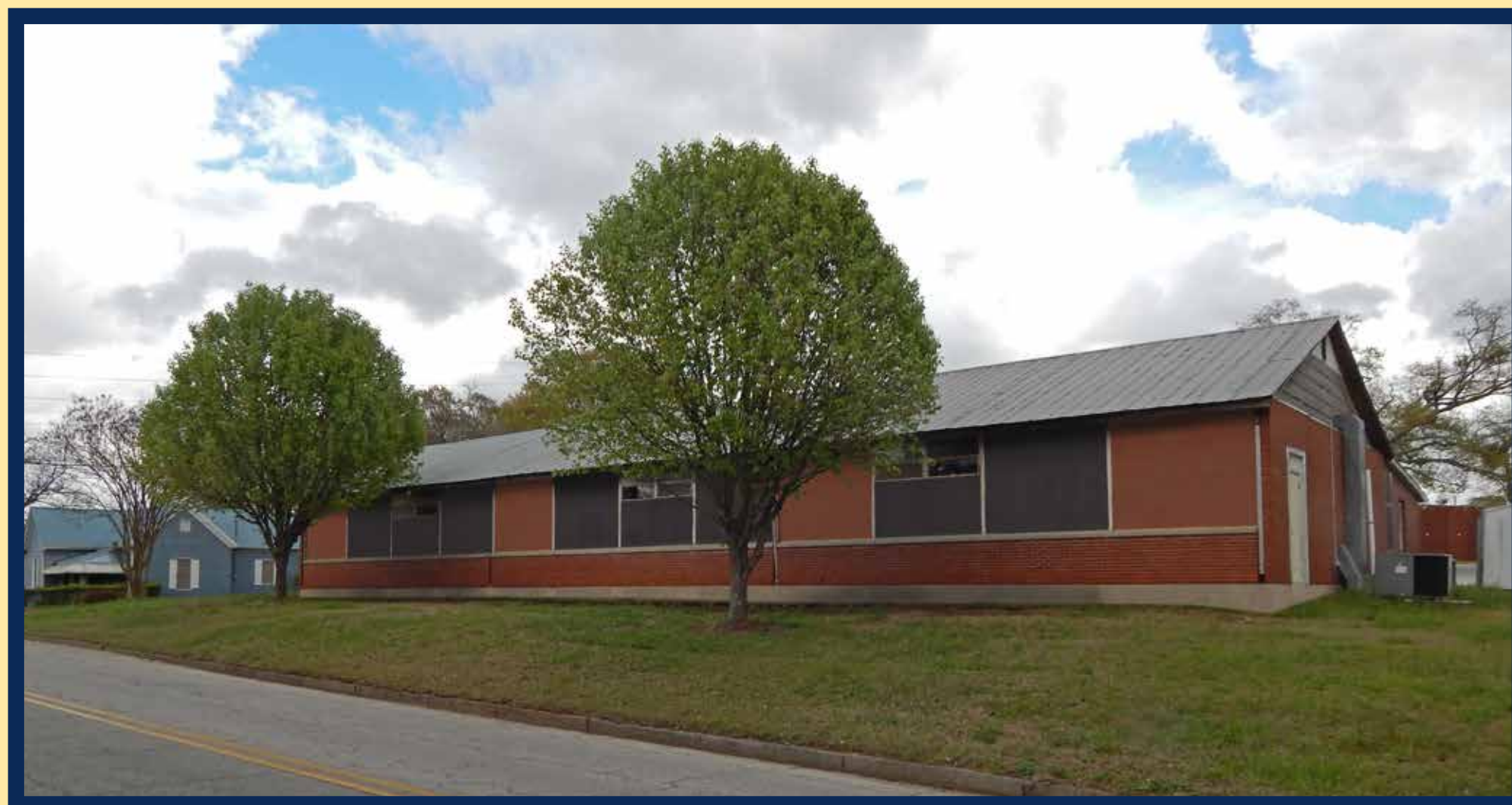
Paint cinderblock and plywood
