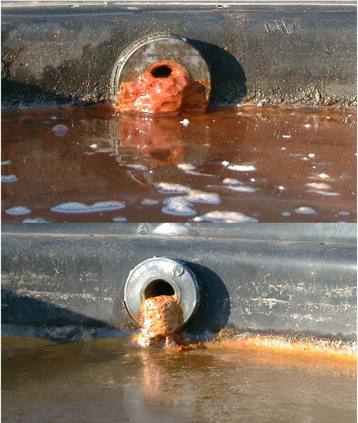
Figure 4.8. Photographs of the tank influent orifice showing iron oxyhydroxide crust precipitated at pH ~2.4. These low pH iron oxyhydroxides crusts may have played a significant role in the sorption and retention of arsenic from the influent ARD.
