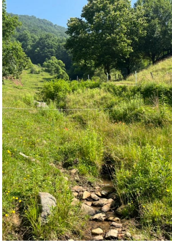
Figure 7. The stream running through the lower pasture, surrounded by grasses and minimal brush. The lack of dense riparian vegetation and the steep gradient in the background contribute to erosion and streambank instability. Photo by author, July 29, 2023.
