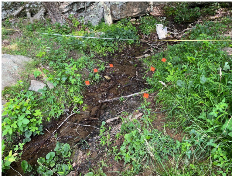
Figure 22. The stream shows signs of erosion and invasive species along its sides. The streambed is full of debris. Photo by author July 12, 2023.
