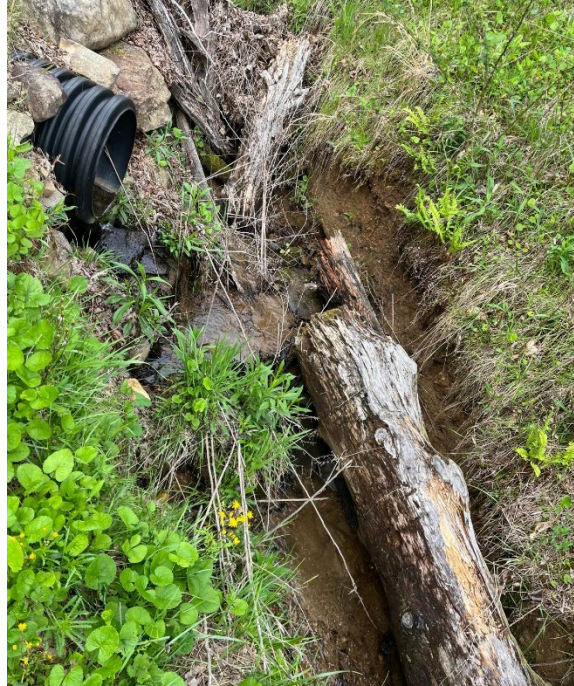
Figure 8. Stream section showing human modifications, including a log obstruction and a plastic corrugated pipe directing water into the stream. Photo by author, April 29, 2023.
