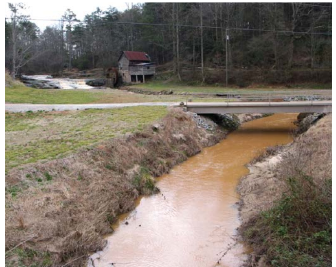
Little Hazel Creek contaminated with sediment.
