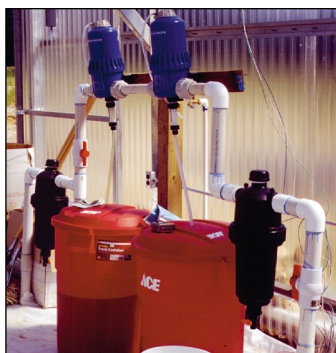
Figure 4. Dual tanks and injectors ensure that chemicals will stay concentrated in the solution.
