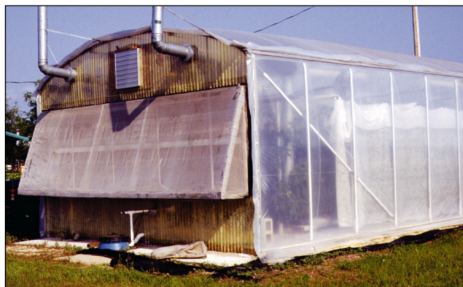
Figure 5. Fine mesh screening over openings prevents insect entry.
