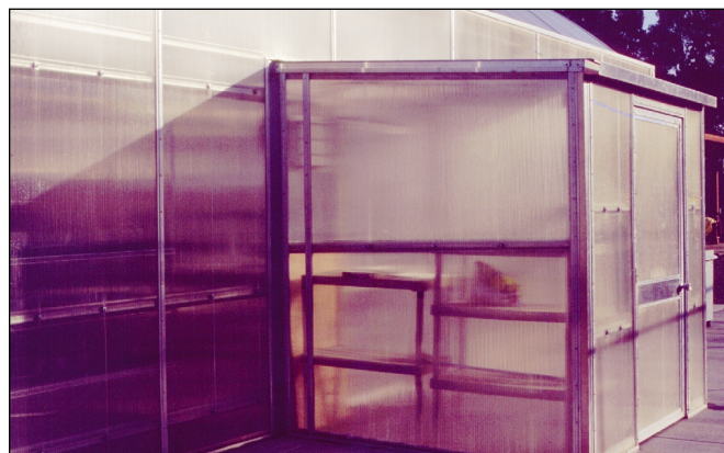
Figure 6. Vestibules at all entries help prevent insect entry.
