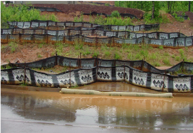
Erosion at construction sites is usually controlled with silt fences.
