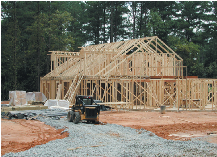
Figure 11. During inspection, most wood members are hidden from view.
