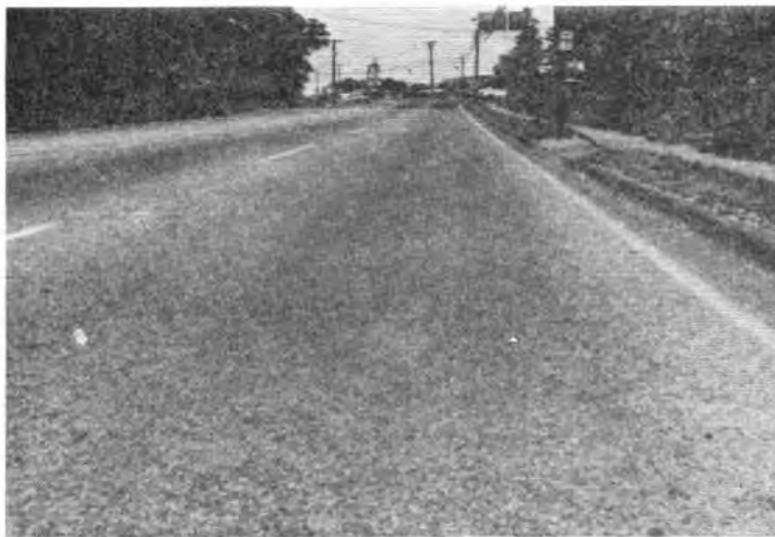
FIGURE 56. MARIANNA SECTIONS AFTER 1.2 \times 10^6 EQUIV. LOADINGS - 3 IN. SURF. AND 4 IN. LOW STABILITY SAND-ASPHALT BASE
